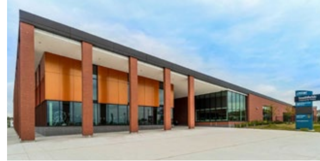
2 View of Southfields Community Centre located at the south east corner of Kennedy Road and Dougall Avenue
