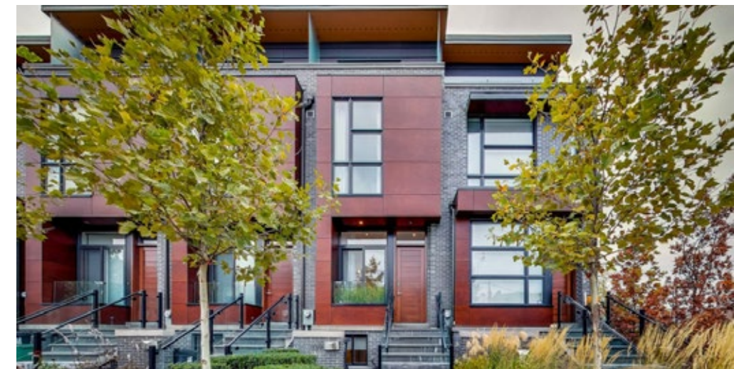
Back-to-back townhouses can provide additional amenity space by incorporating balconies above the garage and front entrance.
