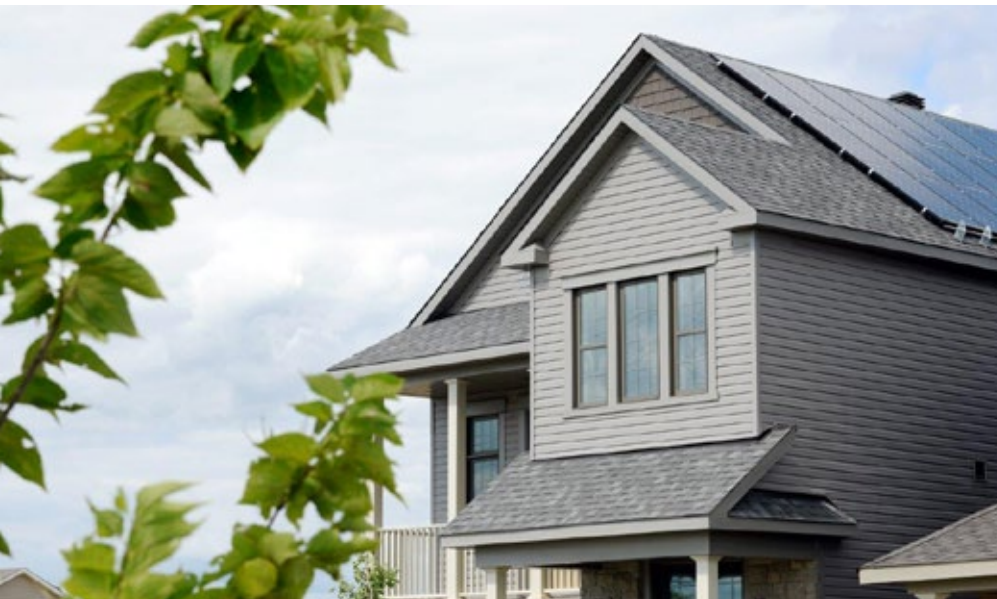
Solar paneling located on residential roofs can provide an alternative and sustainable energy source
