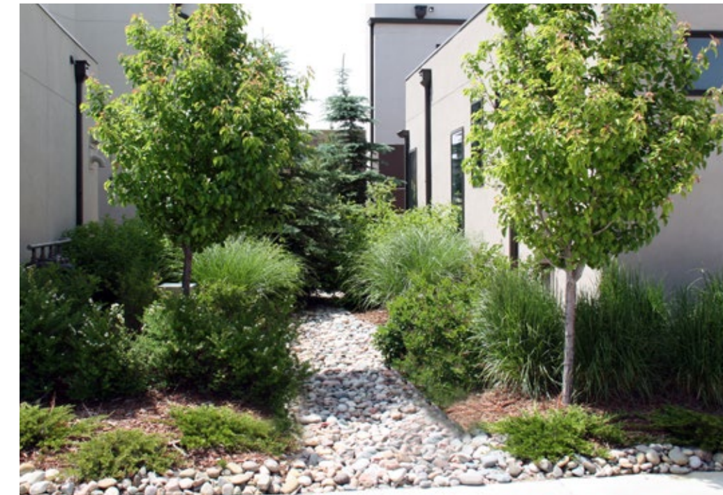
Roof downspouts help direct excess water into soakaway pits. Paired with xeriscape planting, the combination performs well in urban environments due to low-maintenance requirements
