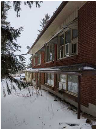
Picture 3: View of the northern side of 12976 Kennedy Road.
