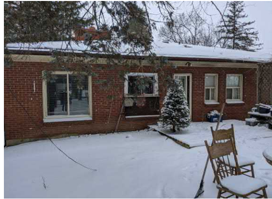
Picture 2: View of the western side of 12976 Kennedy Road.
