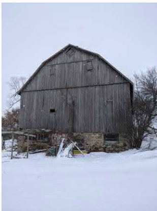
Picture 11: View of the barn located southwest of 3431 Old School Road.
