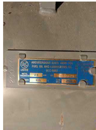
Picture 10: View of the manufacturers stamp on the fuel oil AST.
