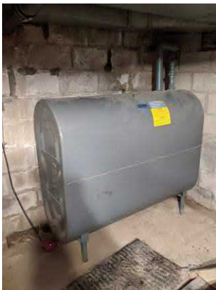
Picture 9: View of the fuel oil AST in the basement on 3431 Old School Road.
