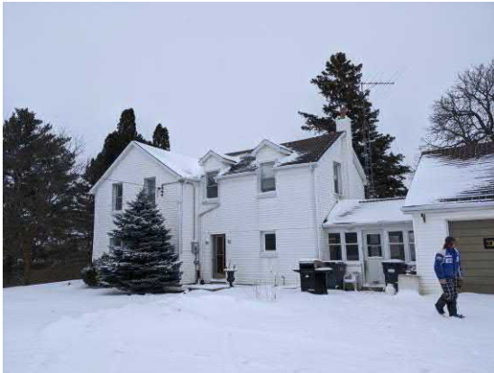
Picture 7: View of the north side of 3431 Old School Road.
