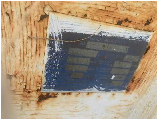
Picture 7: View of the manufacturer's stamp on the gasoline AST.
