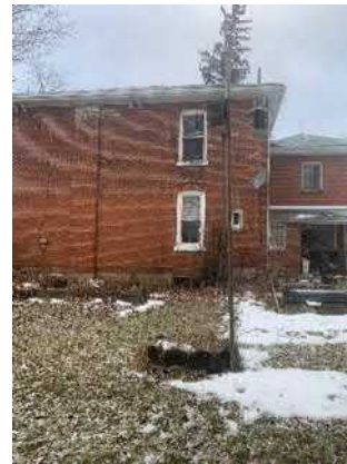
Picture 2: View of the southern wall of Site Building A.
