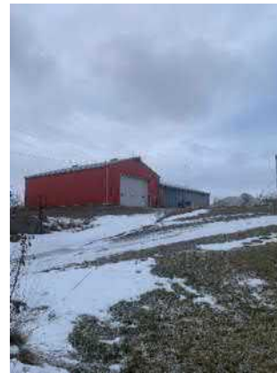
Picture 14: View of the southwestern side of Site Building D.
