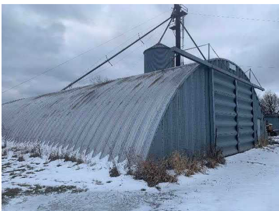
Picture 17: View of the northeastern side of Quonset Hut 1.
