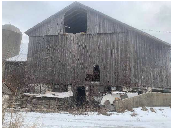
Picture 10: View of the southeastern wall of Barn 1.
