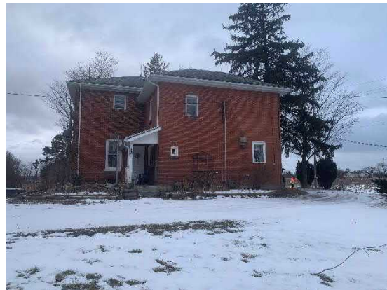
Picture 4: View of the eastern wall of Site Building A.
