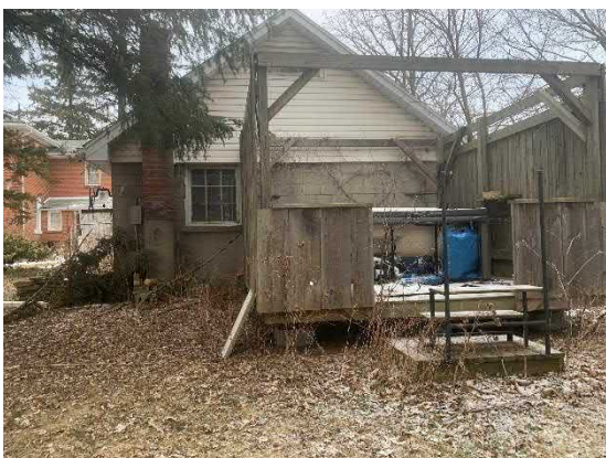
Picture 5: View of the south wall of Shed 1.
