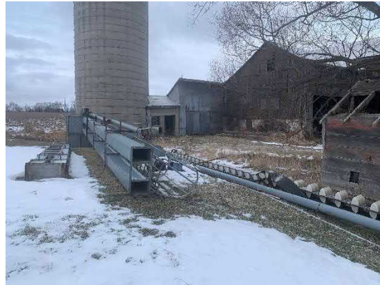
Picture 8: View of the southwestern extent of Barn 1.
