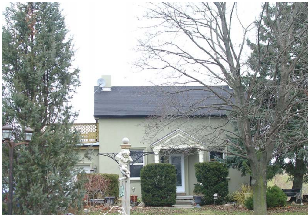
View of west (front) elevation of No. 12409 Kennedy Road.
