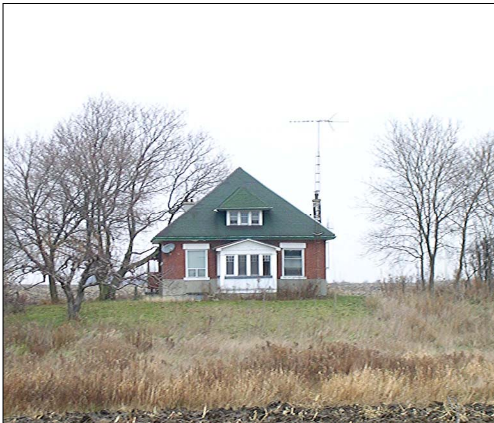
View of west (front) elevation) of farmhouse located at No. 12669 Kennedy Road
