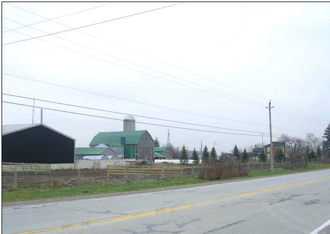
View southeast to farm complex at No. 12035 Dixie Road.
