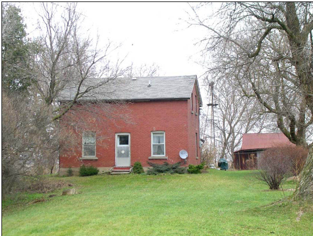
View of west (front) elevation of No. 12551 Kennedy Road.
