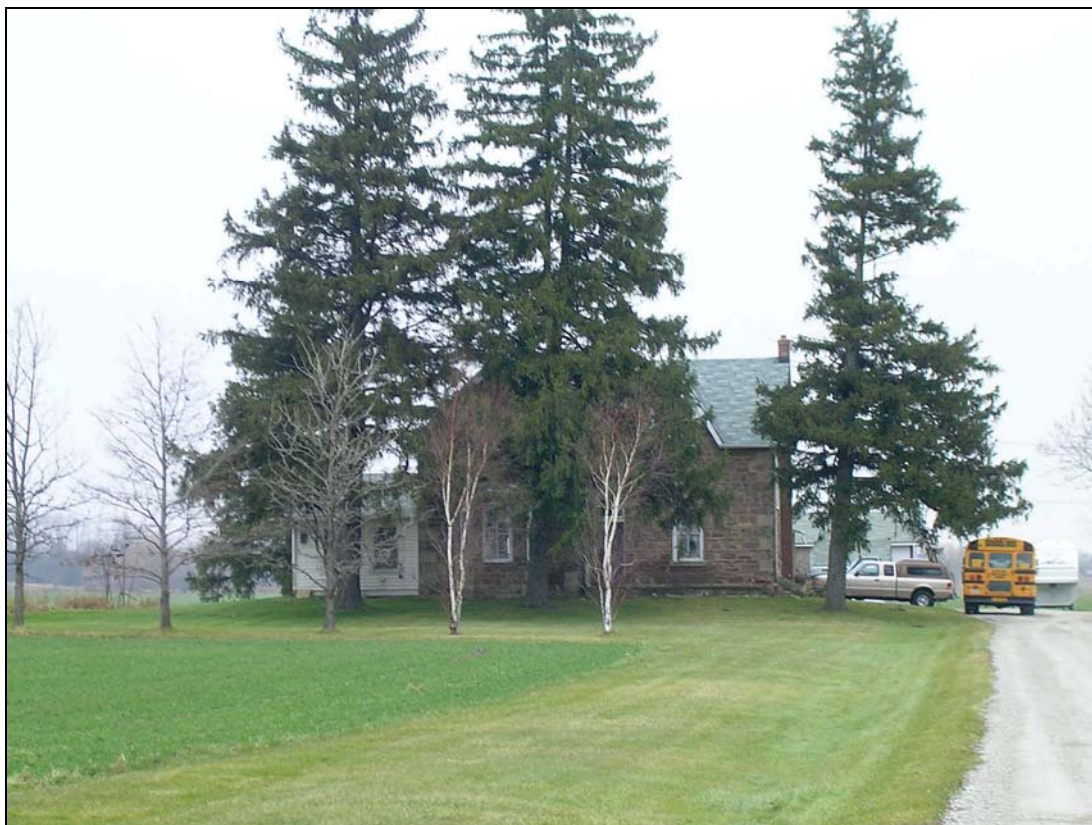
View of west (front) elevation of No. 12701 Highway 10.
