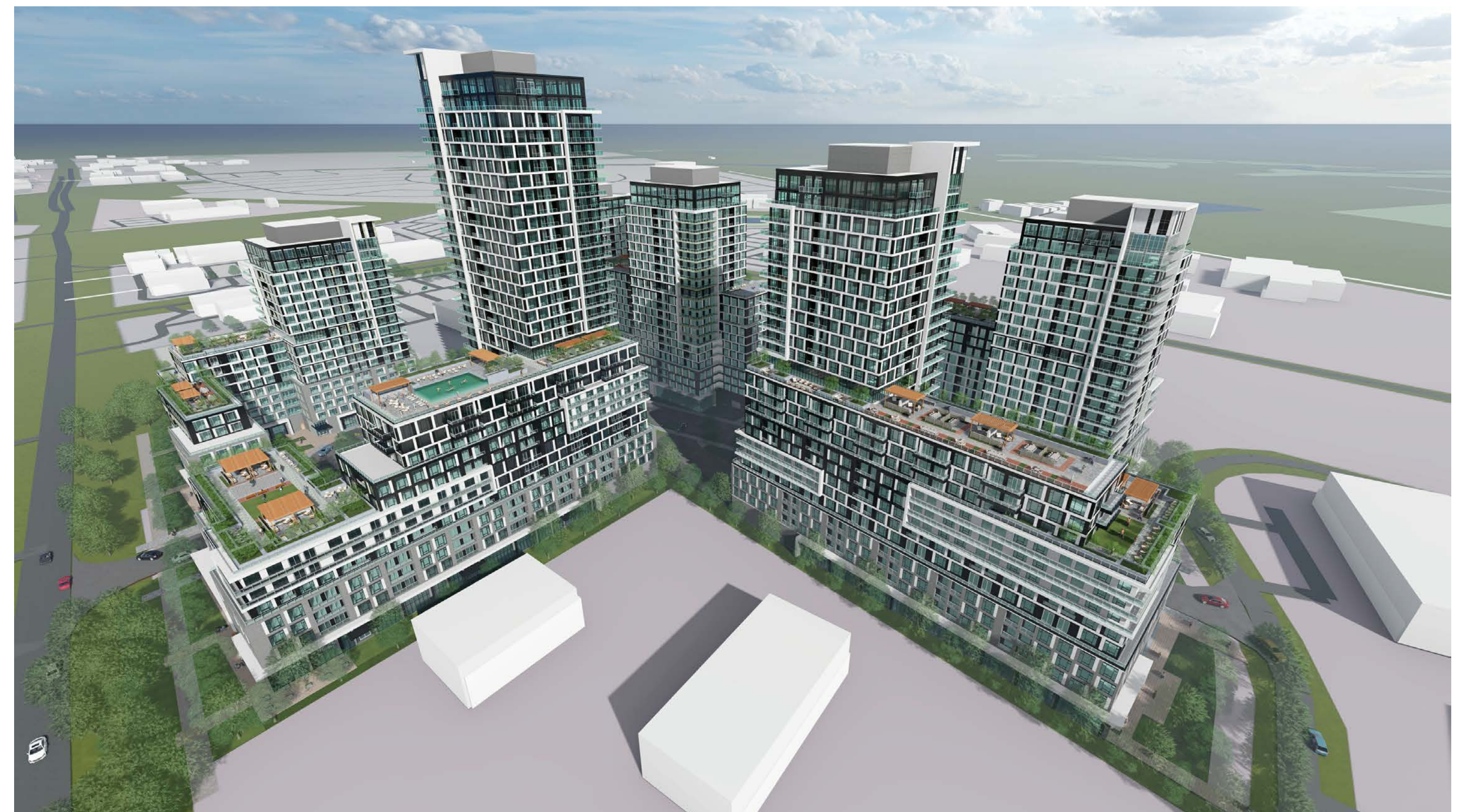
AERIAL VIEW OF THE DEVELOPMENT FROM THE SOUTH 1 NTS A601
