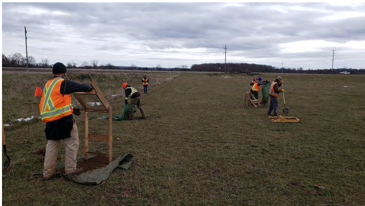
Image 43: Test pit survey at 5 m intervals; facing southeast, November 3, 2020.
