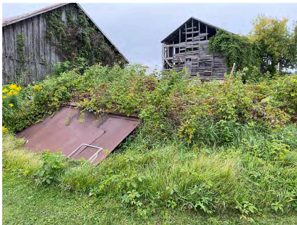
Image 4: A representative example of previous disturbance within the Study Area, old barn structures; facing west, September 14, 2021.
