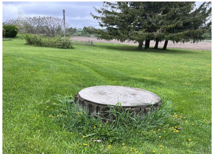
Photo 6: Potable well. Facing north.
