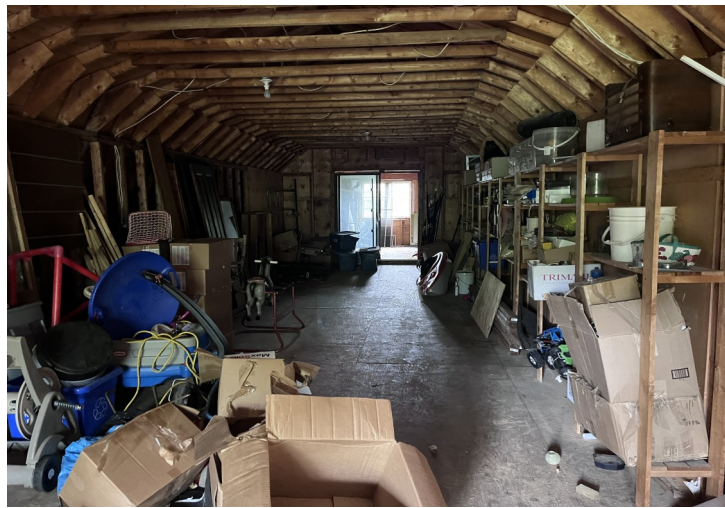
Photo 9: View of upper level of garage.
