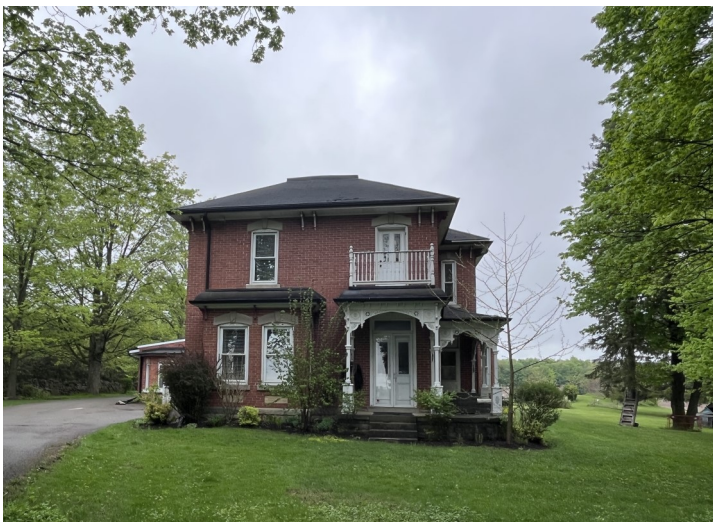
Photo 1: Front of Building A (residential/commercial structure.) Facing northwest
