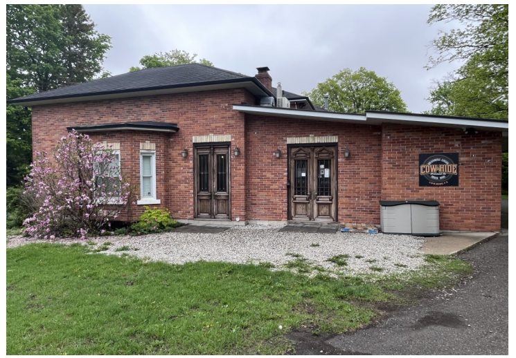
Photo 2: Rear of Building A—(residential/commercial structure.) Facing southeast.
