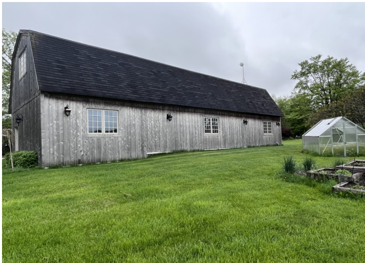
Photo 3: Garage. Facing northwest.
