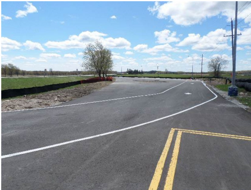
Photo 6 – View of paved driveway area located immediately south of the western portion of the Site, facing southwest.
