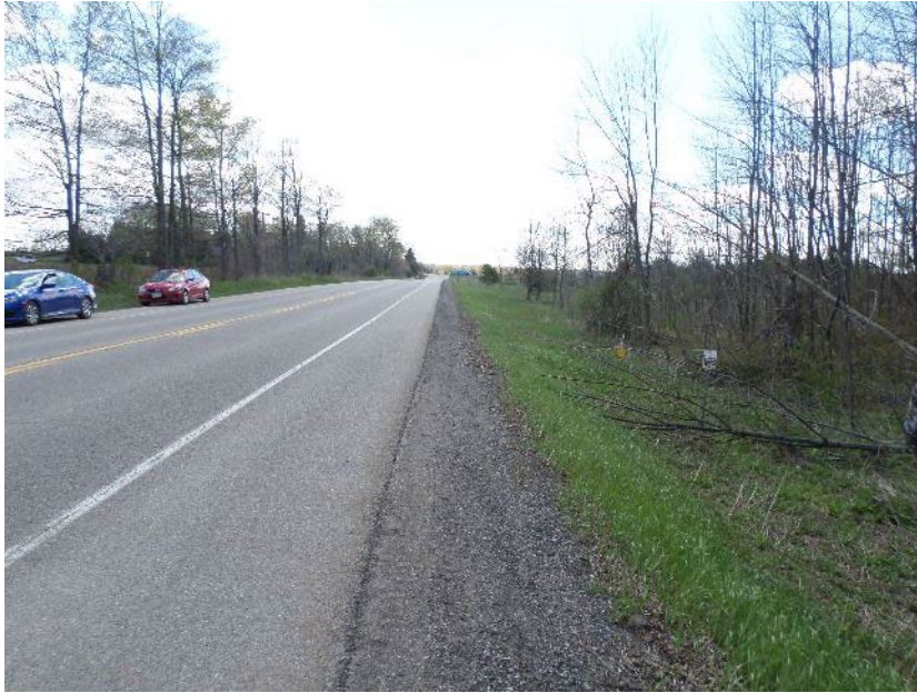
Photo 7 – View of Main Street, east of the Site, facing south.
