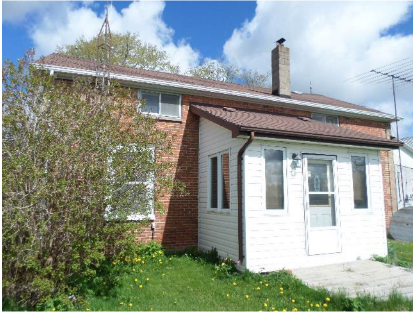
Photo 1 – View of the south side of Building #1, facing north.
