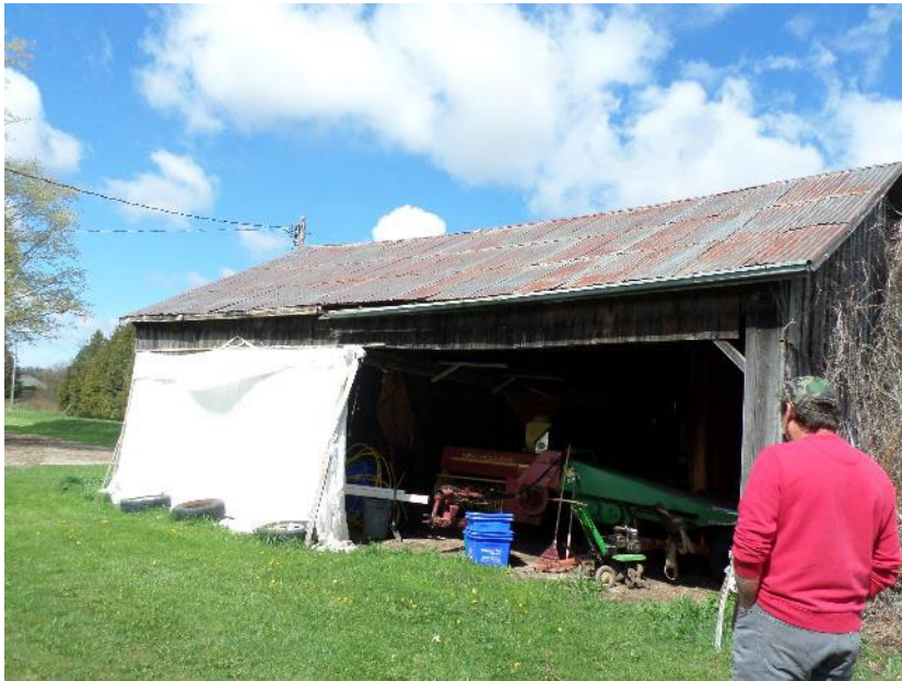
Photo 9 – View of the south side of Building #4, facing northwest.
