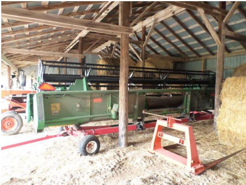
Photo 14 – Interior view of the central portion of Building #5.
