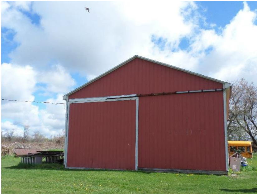
Photo 5 – View of west side of Building #3, facing east.
