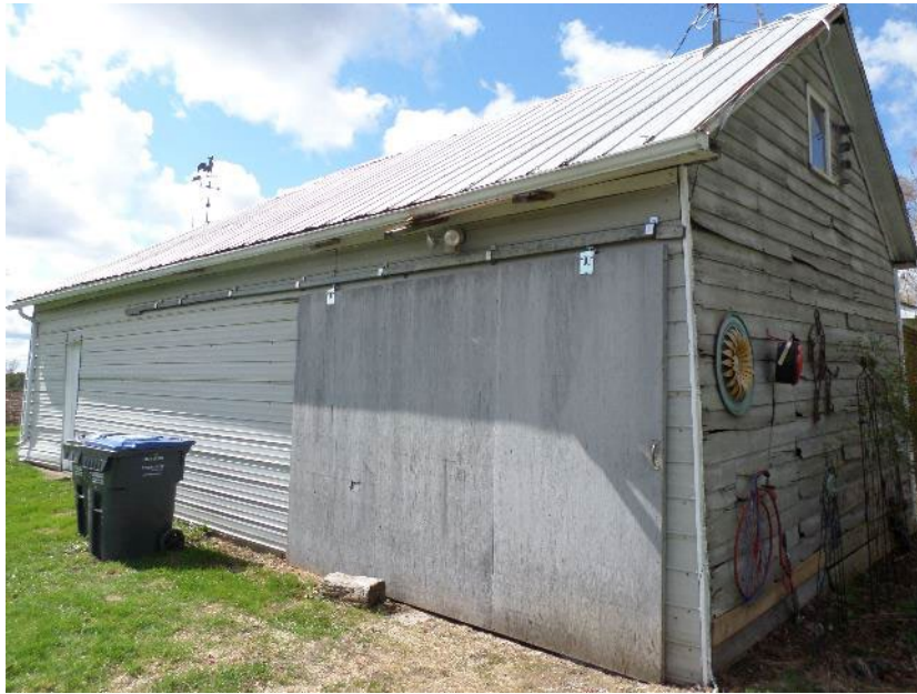
Photo 3 – View of the north and east sides of Building #2, facing south.
