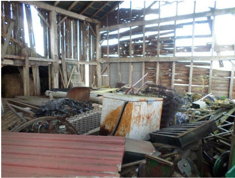
Photo 13 – Interior view of the eastern portion of Building #5.
