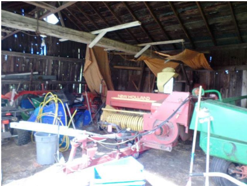
Photo 10 – Interior view of Building #4.
