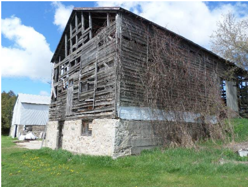
Photo 12 – View of the south and east side of Building #5, facing northwest.
