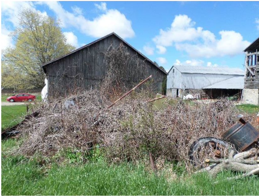
Photo 11 – View of the east side of Building #4, and scrap metal area located immediately east of Building #4, facing west.
