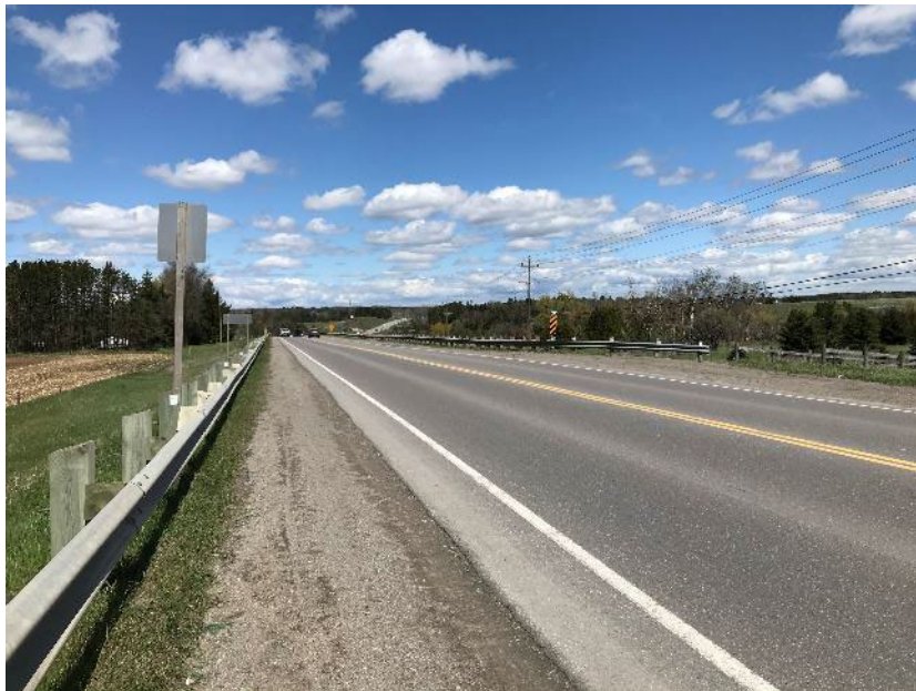
Photo 6 – View of Charleston Side Road, facing east.
