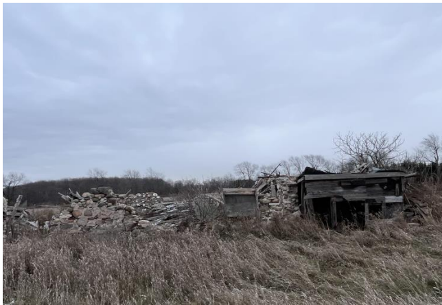
Photo 7: View of the second demolished building (Building 3) that was present on Site located 35 m southeast of the current building, facing east.
