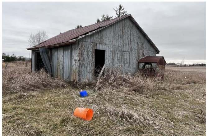
Photo 4: View of the exterior of a storage building (Building 1) located 60 m east of Charleston Sideroad, facing northeast.
