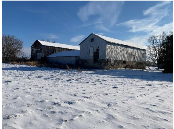
Plate 31: Barn complex, facing east
