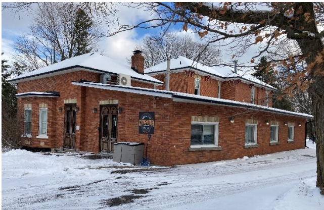
Plate 15: Oblique view of north and west elevations, including rear and side additions
