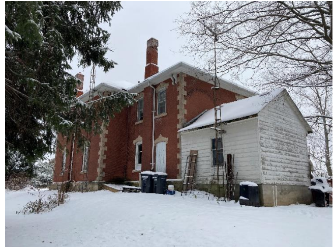
Plate 3: Oblique view of west and south elevations, including rear addition
