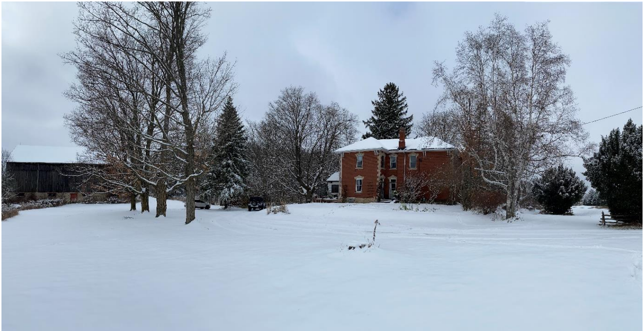
Plate 1: View across driveway towards house and barn, facing southwest
