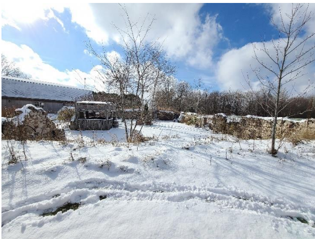
Plate 17: Barn foundation ruins, looking southwest
