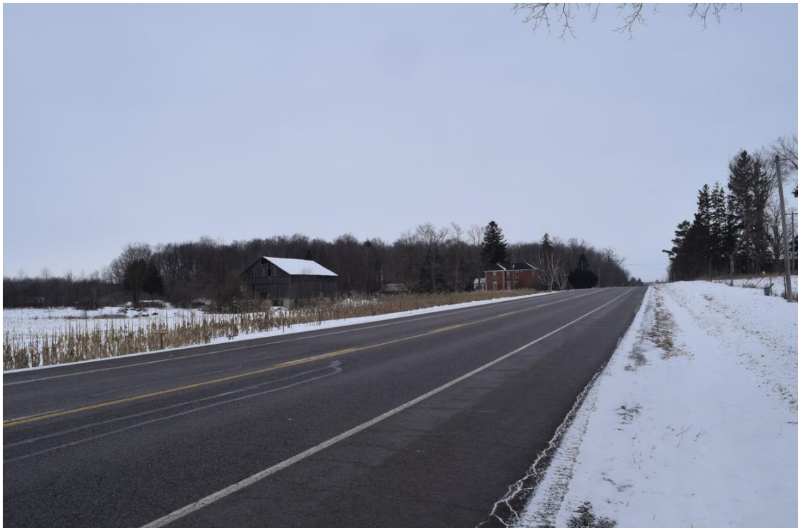
Figure 5: Main Street north of Charleston Sideroad, exhibiting paved asphalt, two-lane roadway with partially paved and partially gravelled shoulder (latter under snow) accompanied by ditch, facing northwest.
