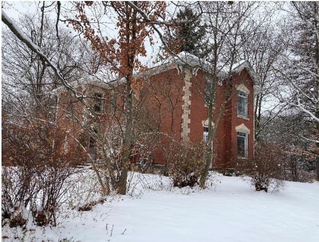
Plate 2: Oblique view of east and north elevations of residence
