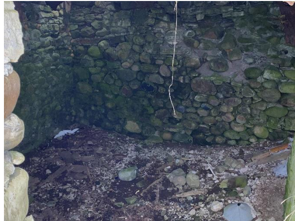
Plate 11: Interior of smaller fieldstone foundation ruins
