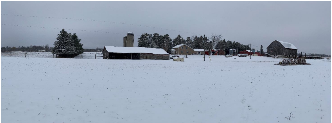
Plate 20: View towards the building complex, facing northwest
