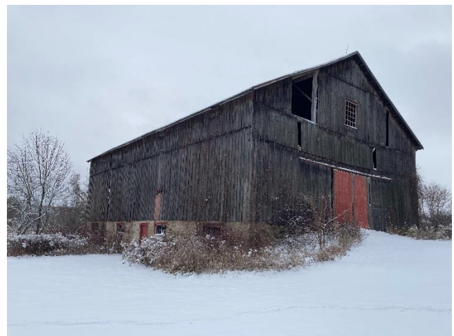
Plate 5: North and west elevations of the barn
