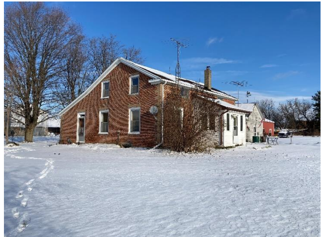
Plate 29: Oblique view of south and east elevations
