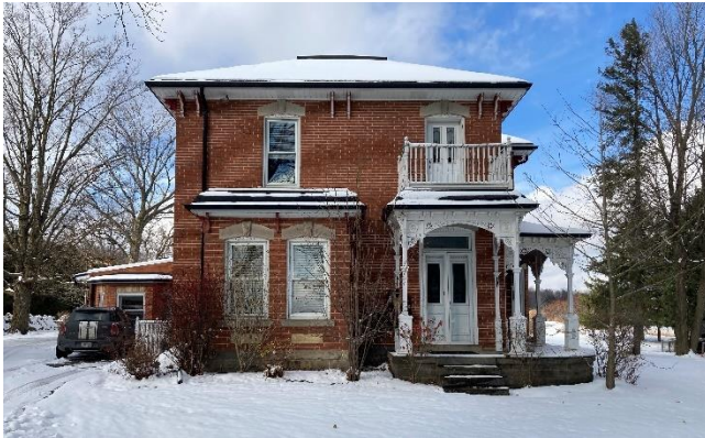
Plate 13: South elevation of the residence
