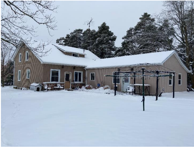
Plate 21: Oblique view of south and east elevations of the residence.
