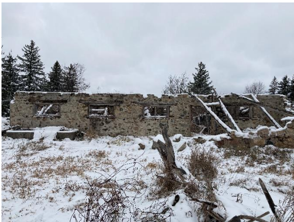
Plate 8: Larger fieldstone foundation ruins
