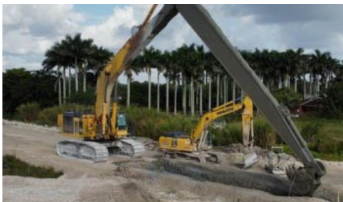
Figure 18: Self-Hardening CB (Cement-Bentonite) Slurry Wall Method (Geo-Solutions, 2025)
