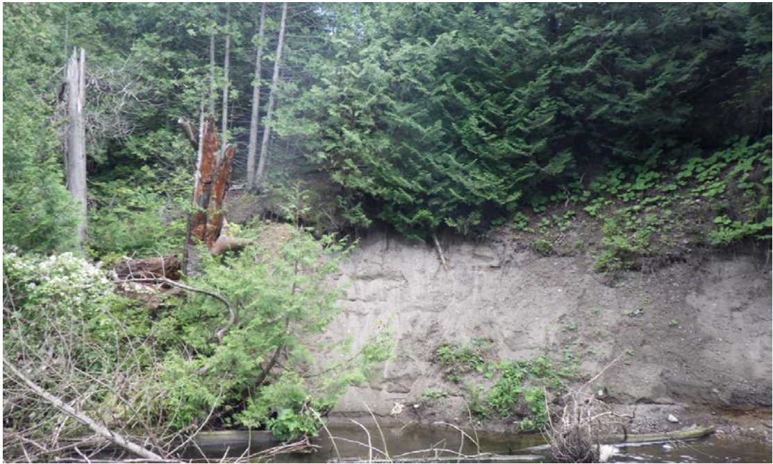
Photo 17 Credit River, Caledon, ON July 25, 2024
