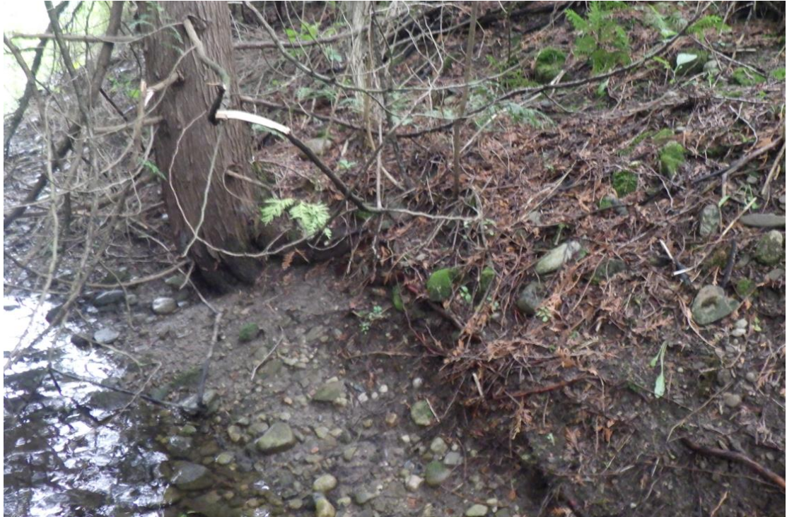
East Ponds Outlet Channel – Bank materials consisted predominantly of silt and fine to medium sand, with small to large cobbles.
