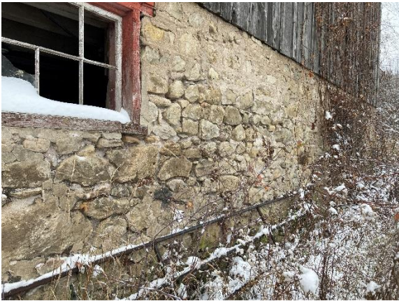
Plate 34: Barn fieldstone foundation
