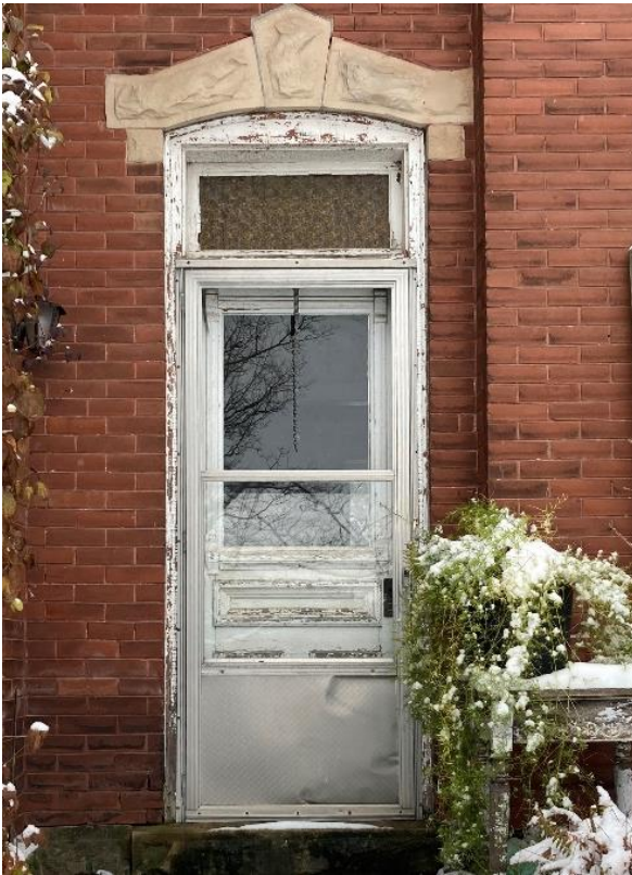
Plate 16: Detail of one of the east entrance doors
