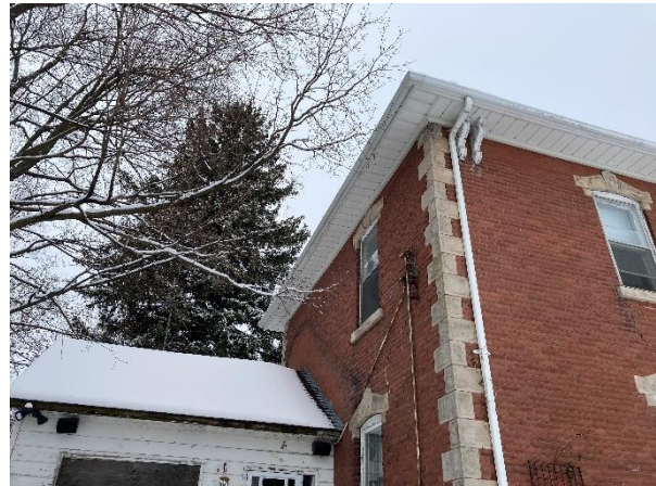
Plate 29: Second floor and eaves of south elevation
