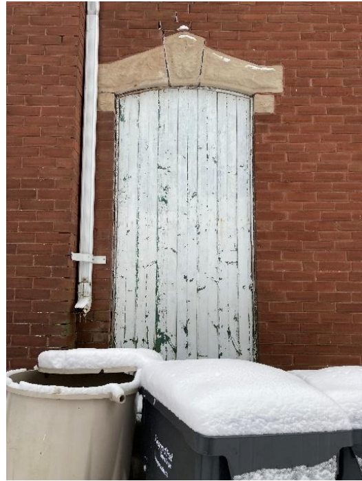
Plate 25: Blind entrance on west elevation
