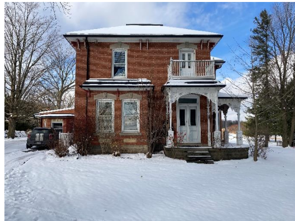
Plate 3: Farmhouse at 1402 Charleston Sideroad
