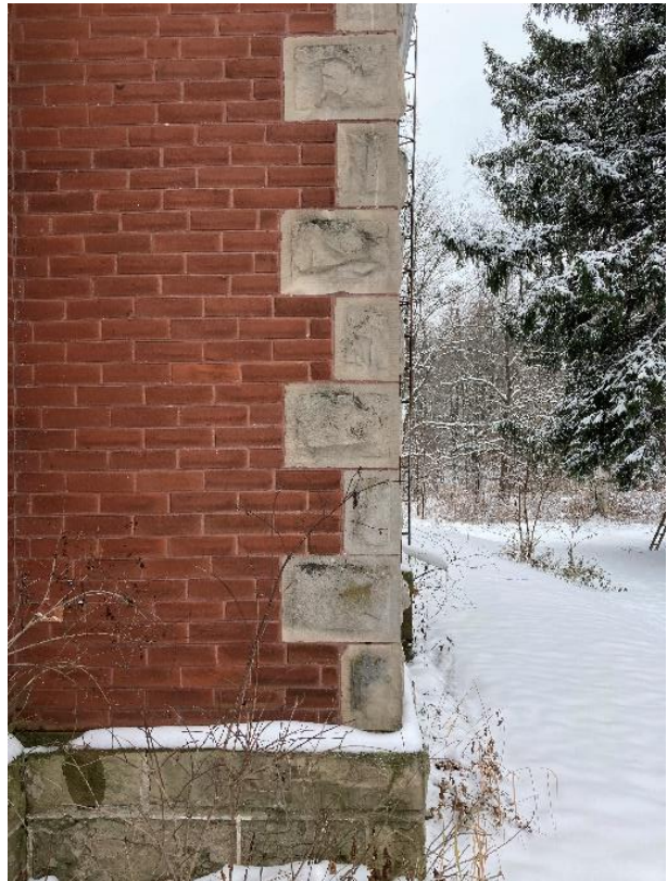
Plate 17: Representative example of stone quoins
