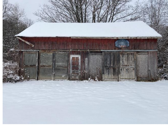
Plate 37: Board-and-batten driven shed
