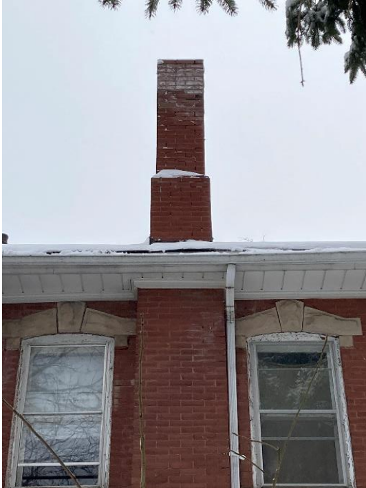
Plate 24: South chimney on west elevation
