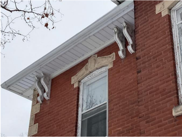
Plate 12: Overhanging eaves and paired bracket detail
