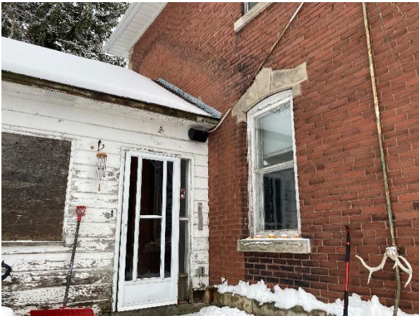
Plate 28: Main floor window and entrance of south elevation
