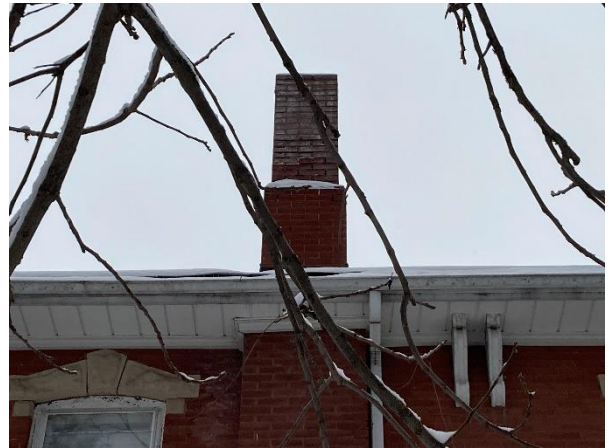
Plate 23: West chimney of west elevation
