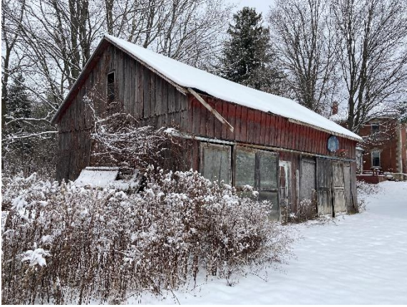
Plate 36: Board-and-batten driven shed
