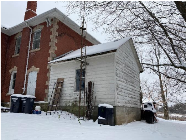
Plate 30: Basement access on west elevation
