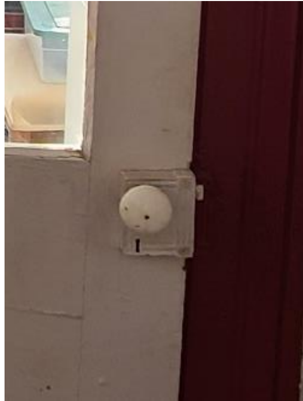
Plate 26: Rim lock detail of east entry door
