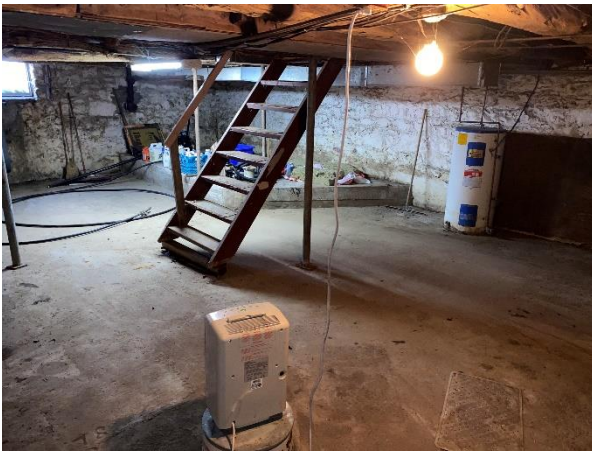
Plate 30: Basement of the farmhouse
