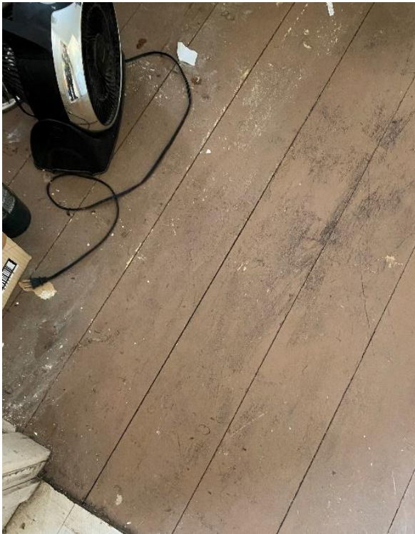
Plate 72: Wood floors of side addition storage room
