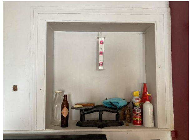
Plate 41: Frame from original west elevation window
