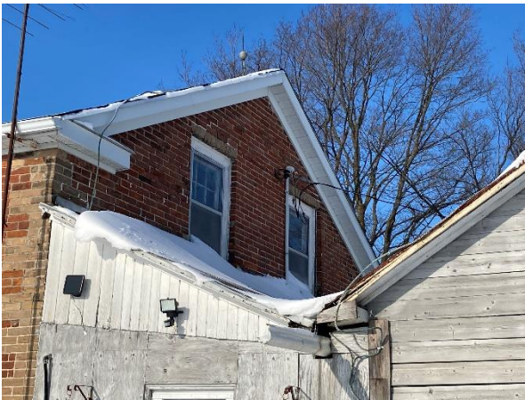
Plate 27: Portion of north elevation of original main block visible from exterior
