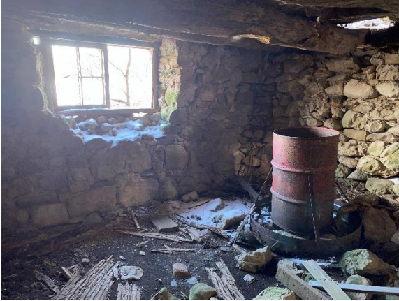
Plate 93: North barn interior showing rubble stone foundations
