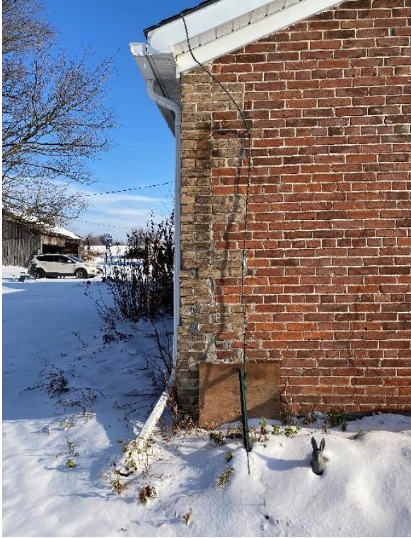
Plate 64: Detail of southwest corner, showing quoins
