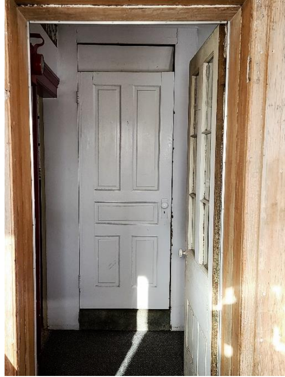
Plate 46: Five panel door leading to the second floor
