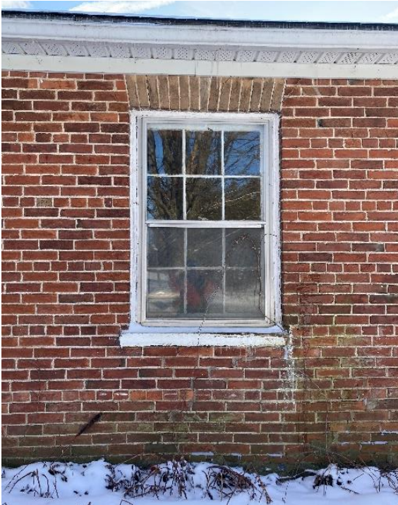
Plate 66: West elevation window
