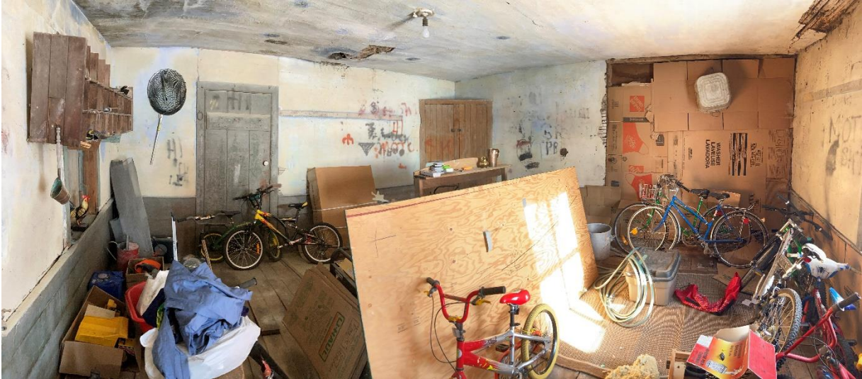
Plate 82: East storage room of north addition
