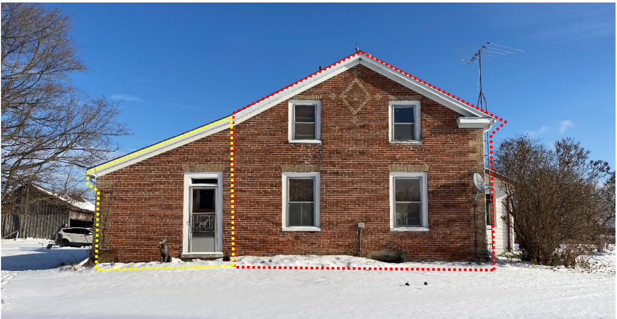
Plate 13: South elevation, original main block is outlined in red, rear addition is outlined in yellow
