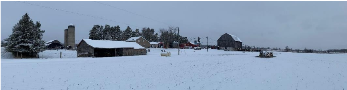
Plate 3: Farm complex at 18501 Mississauga Road (Listed on the Town of Caledon's heritage register)
