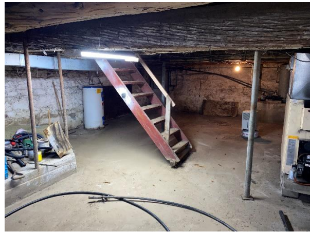
Plate 31: Basement of the farmhouse
