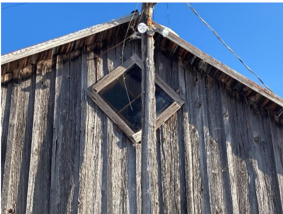
Plate 103: Diamond gable window on south elevation of Outbuilding No. 1
