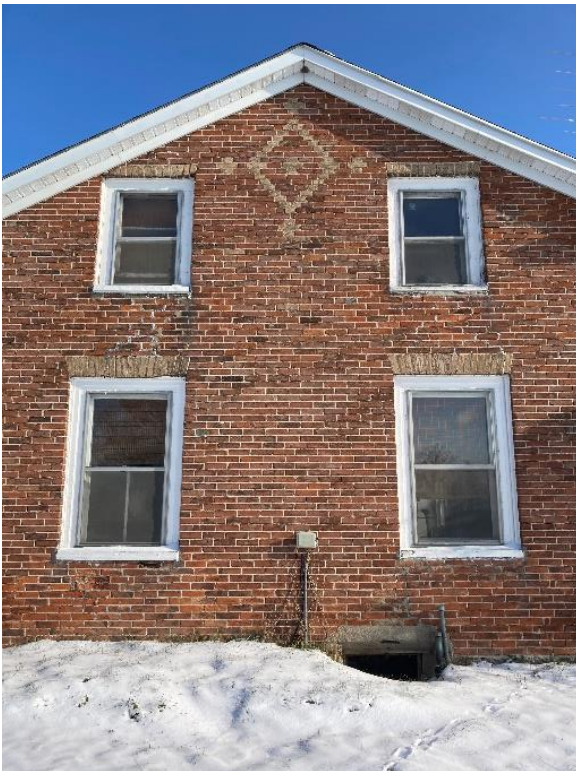
Plate 17: South elevation of main block
