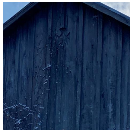
Plate 104: Diamond cross owl hole on north elevation of Outbuilding No. 1
