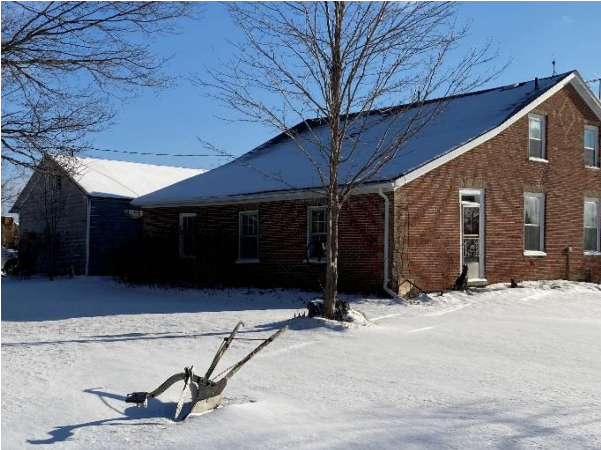
Plate 63: Oblique view of side addition
