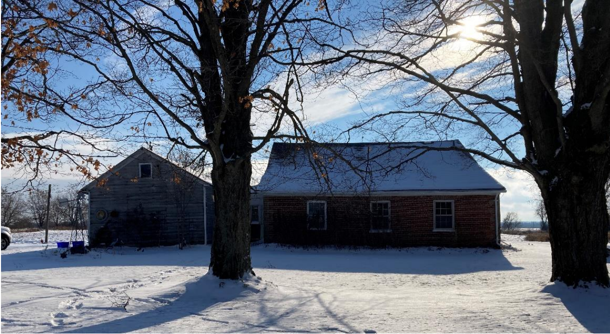
Plate 16: West elevation of the farmhouse
