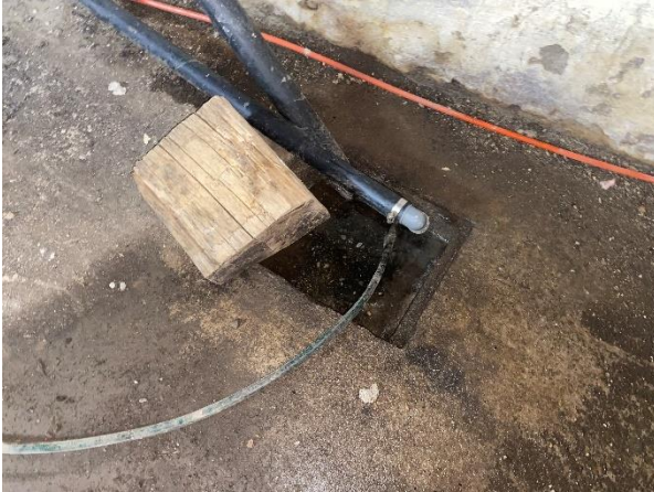
Plate 32: Poured concrete basement flooring
