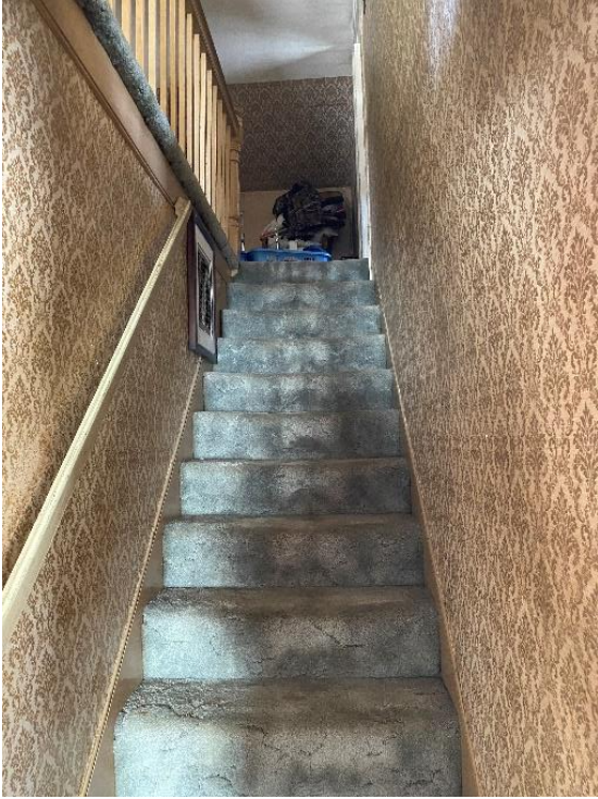
Plate 45: Stairway to second floor
