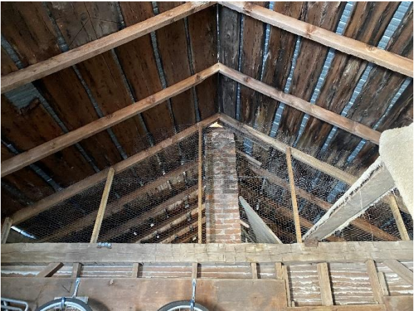
Plate 84: Central brick chimney remnant in north addition
