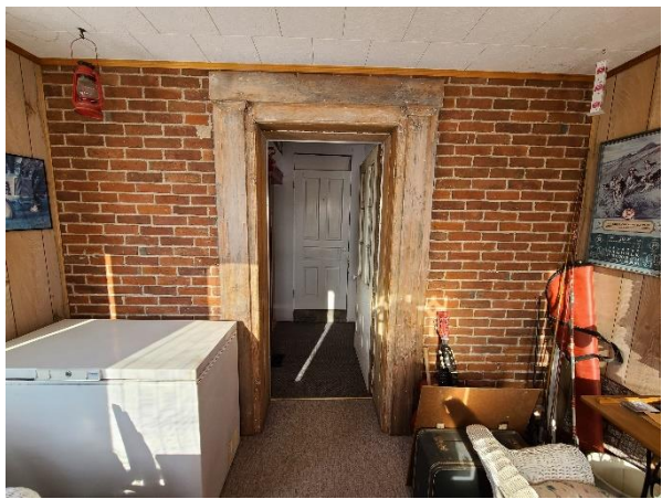
Plate 24: Entrance to house, within porch
