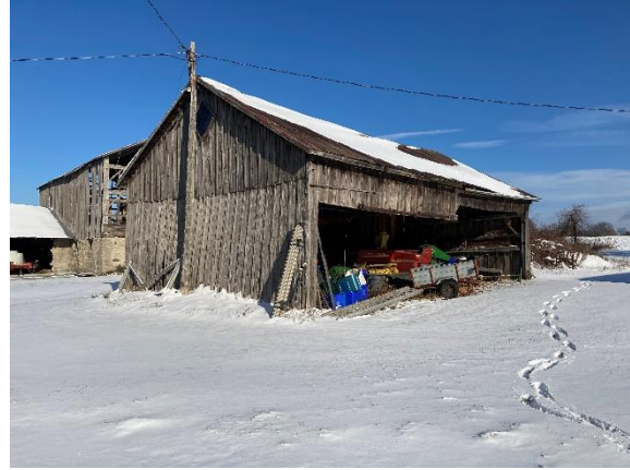
Plate 100: Outbuilding No. 1 (timber framed drive shed)
