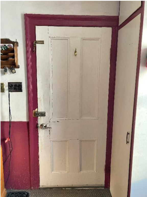
Plate 29: Interior view of north elevation entry door
