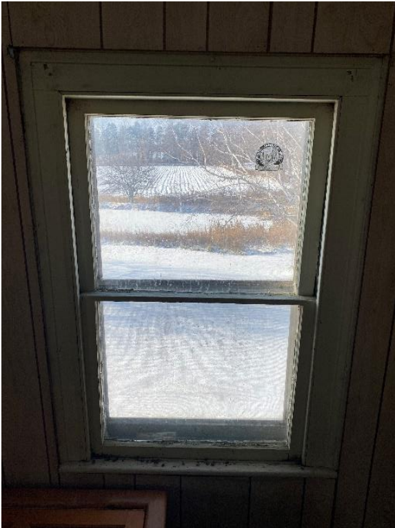
Plate 49: Detail of south window of southeast second floor room
