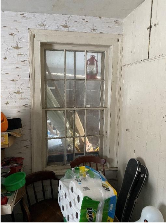
Plate 74: North elevation window
