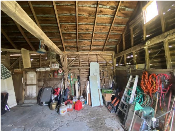
Plate 83: West storage room of north addition
