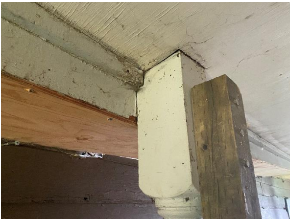
Plate 78: Original veranda pillar
