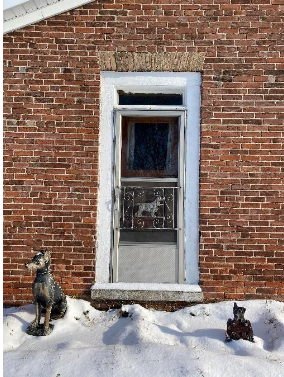
Plate 65: South elevation entrance
