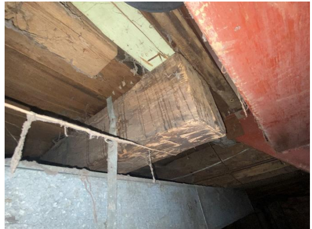
Plate 35: Hand squared floor joist
