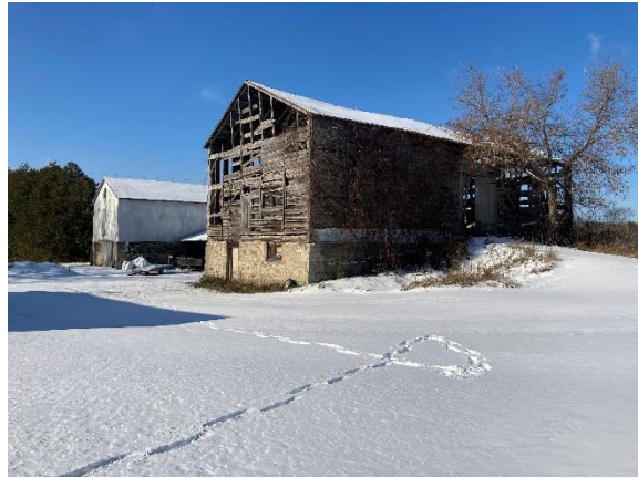
Plate 90: North and east elevations of north barn
