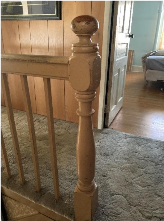
Plate 47: Newel post, handrail, and balustrade of second floor
