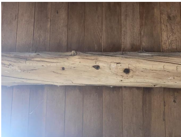
Plate 36: Main block plank subflooring
