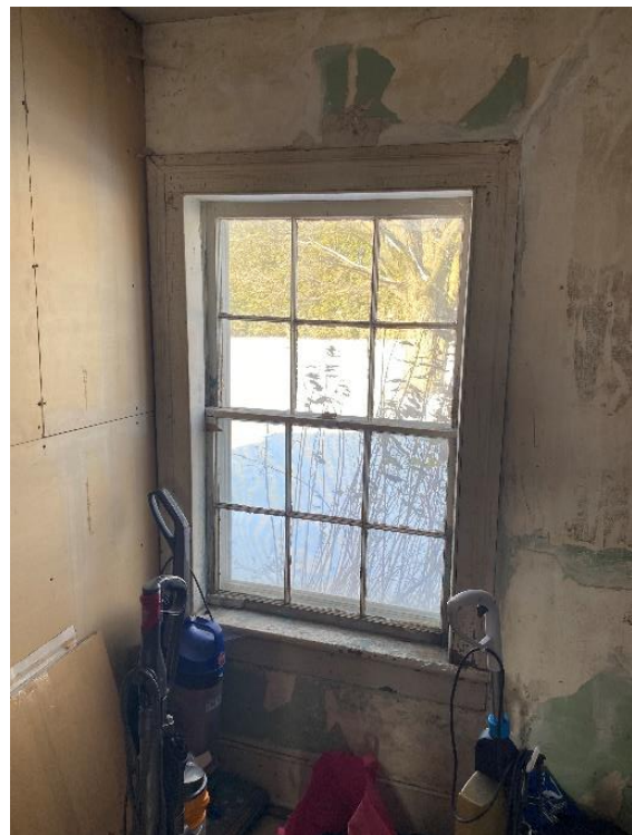
Plate 73: Side addition storage room window on west elevation
