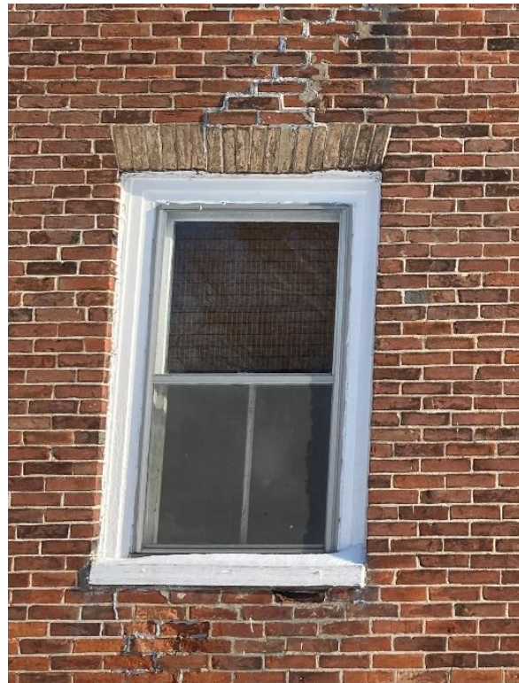
Plate 18: Main block window example
