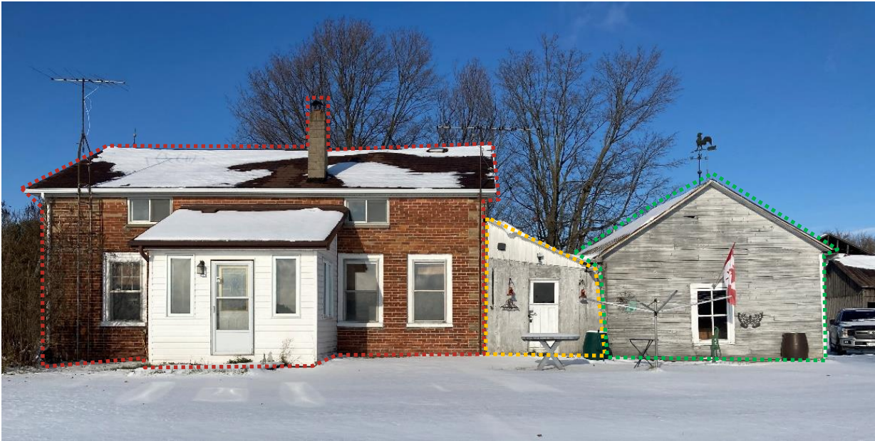
Plate 12: Front façade (east elevation) of the farmhouse, showing original main block (outlined in red), side passage (yellow), and summer kitchen (green).
