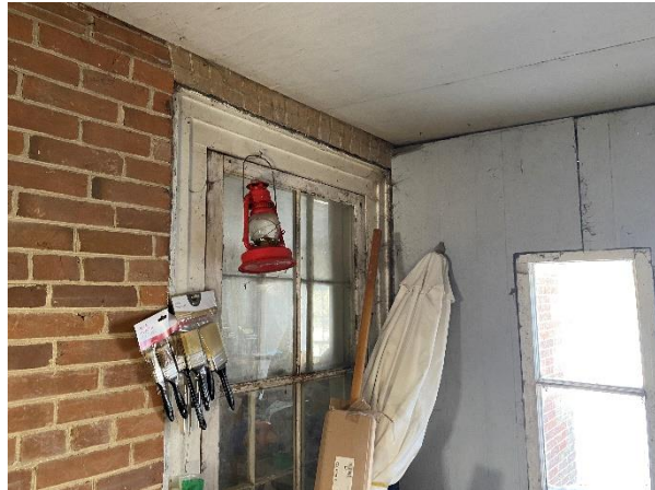
Plate 67: North elevation window
