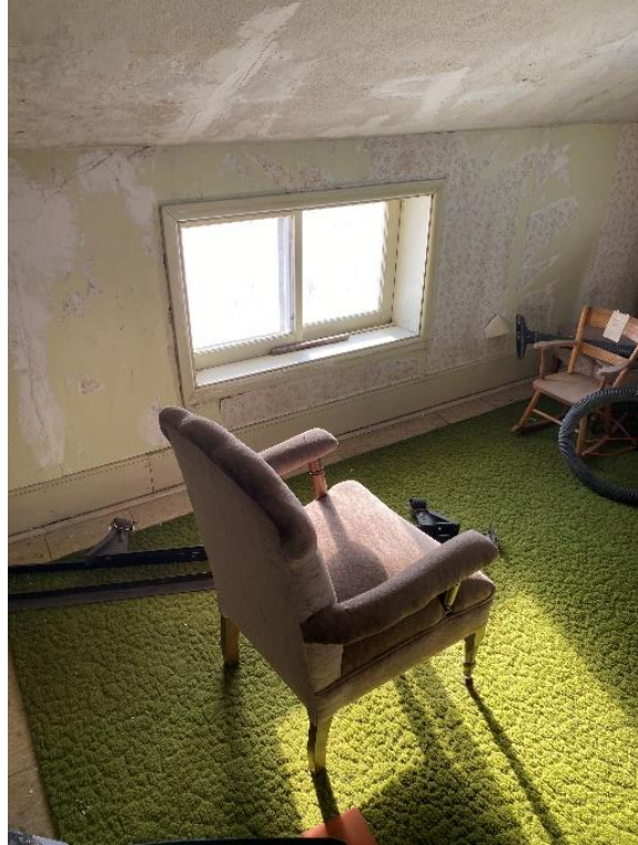
Plate 50: East window of southeast second floor room
