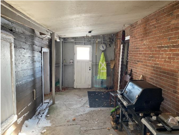
Plate 76: Enclosed frame and plywood side passage on the north elevation
