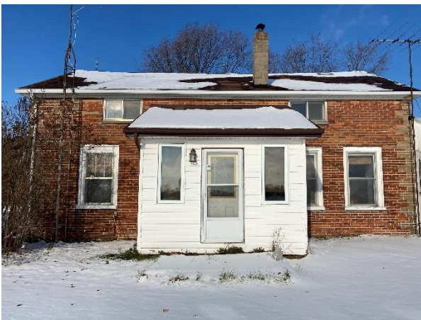
Plate 23: Porch entry on east elevation (original front façade)
