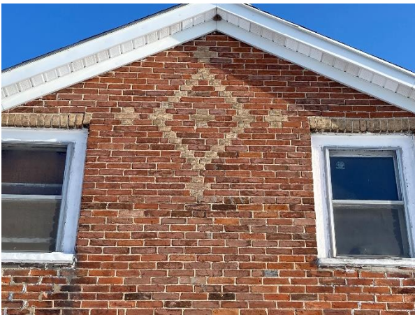
Plate 21: Buff brick diamond and cross pattern
