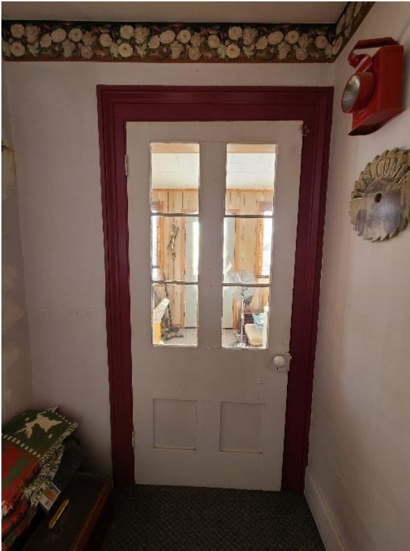
Plate 25: Interior view of original front entry door (located on the east elevation)
