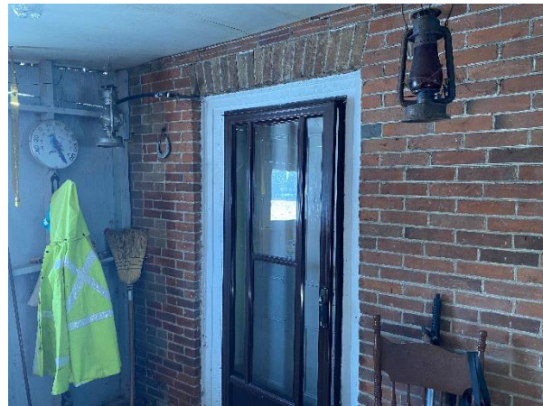
Plate 28: North elevation entrance
