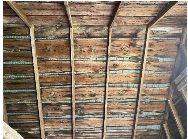
Plate 86: Wide board roof sheathing
