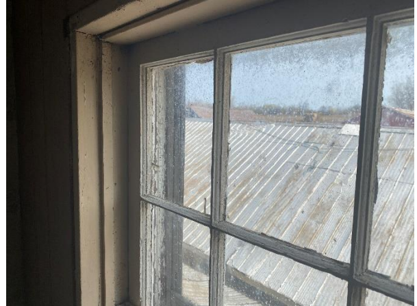
Plate 52: Detail of six-over-six sash window
