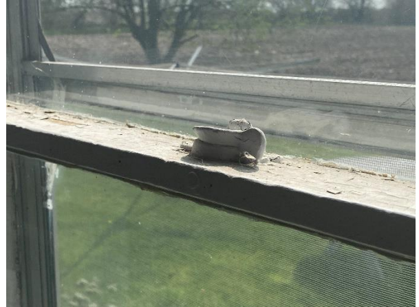
Plate 43: East elevation window
