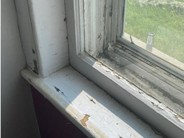
Plate 42: East elevation window
