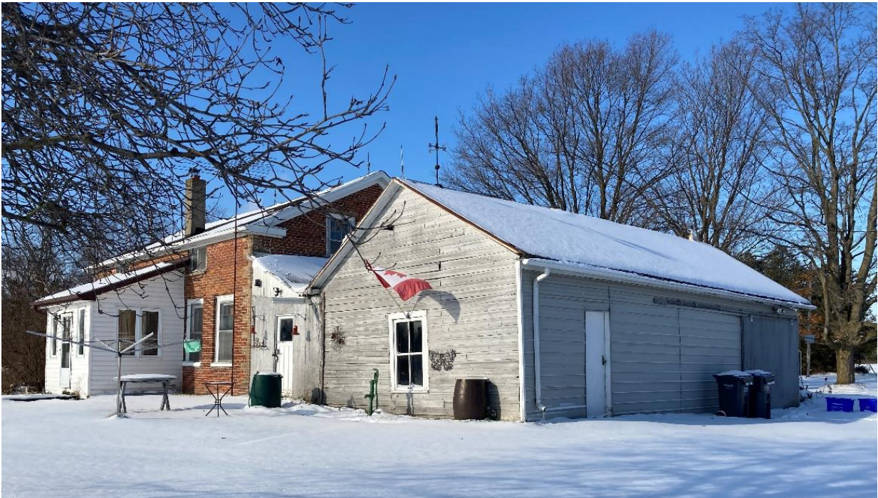
Plate 15: Oblique view of east (left) and north (right) elevations
