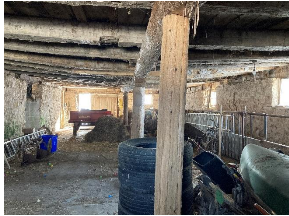
Plate 96: South barn interior showing hand hewn beams and redundant mortices
