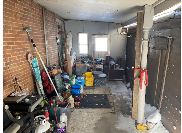
Plate 77: Enclosed frame and plywood side passage on the north elevation
