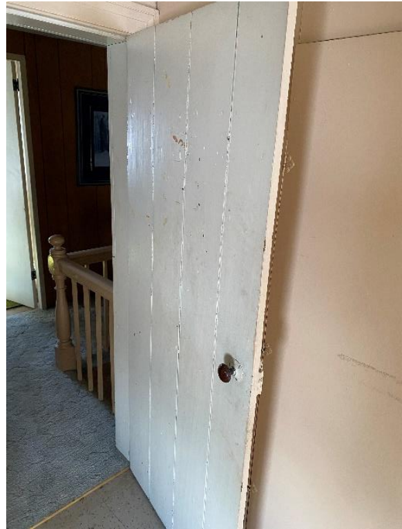
Plate 56: Vertical panel door to northeast room
