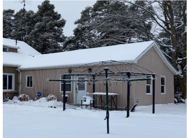
Plate 48: South and east elevations.
