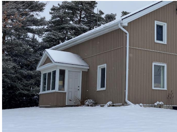
Plate 18: West elevation enclosed porch.
