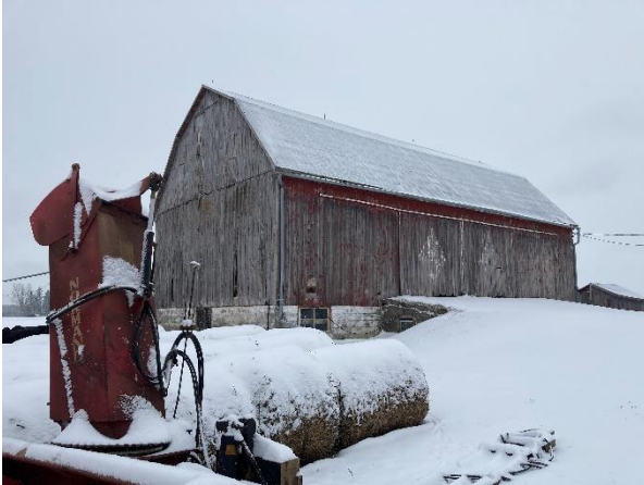
Plate 53: North and west elevation of Barn No. 2.
