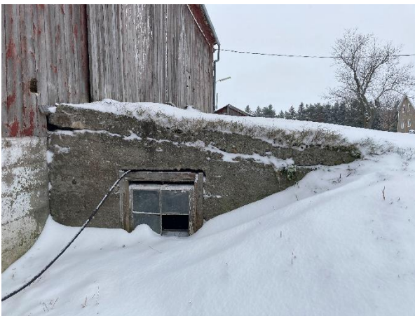
Plate 57: Barn No. 2 wingwall window.
