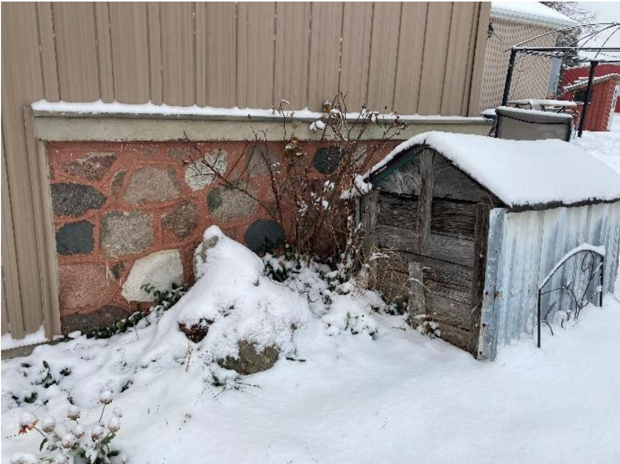
Plate 46: Fieldstone veneer indicating the limit of porch addition on main block.
