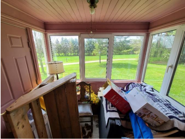
Plate 27: Enclosed front porch on west elevation
