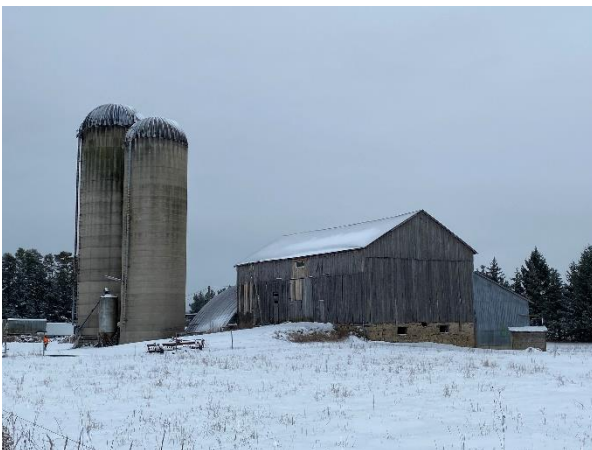
Plate 51: North and west elevation of Barn No. 1.
