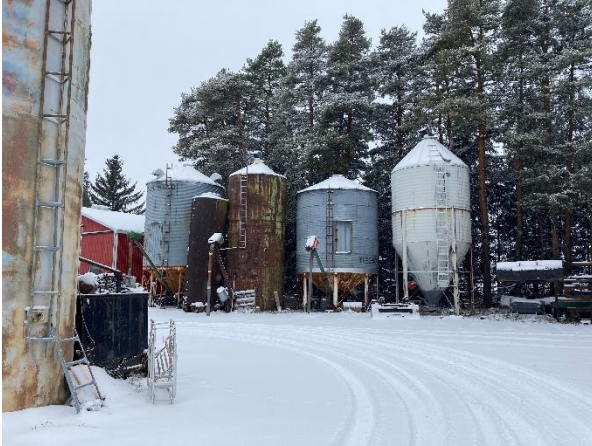
Plate 65: Additional silos between Outbuildings No. 3 and 4.
