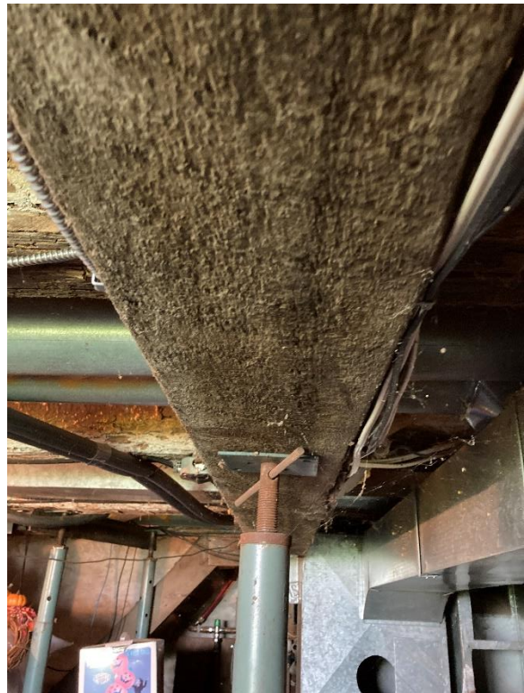
Plate 26: Machine cut timber floor joist
