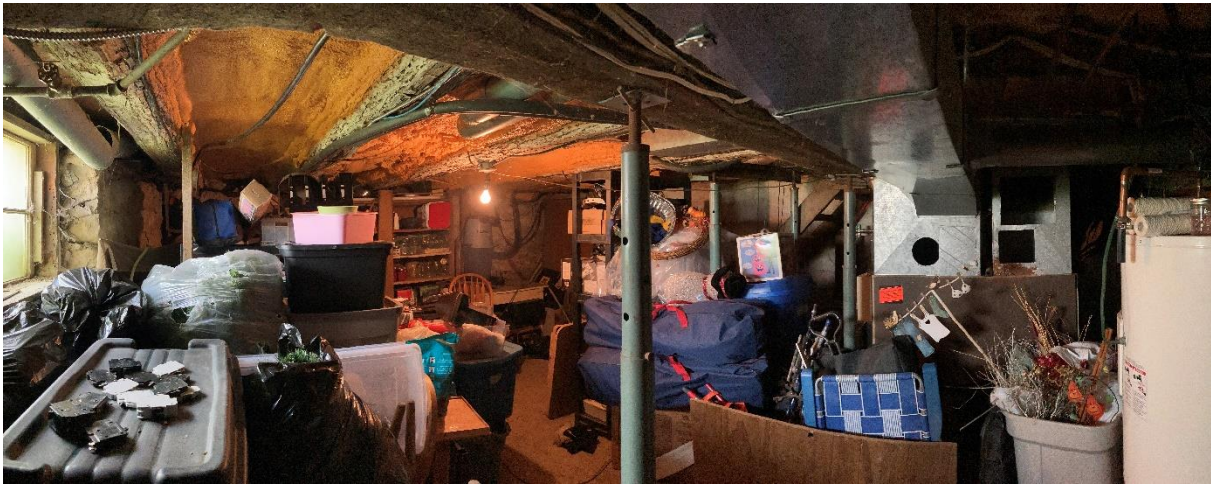
Plate 21: View of basement from southeast corner
