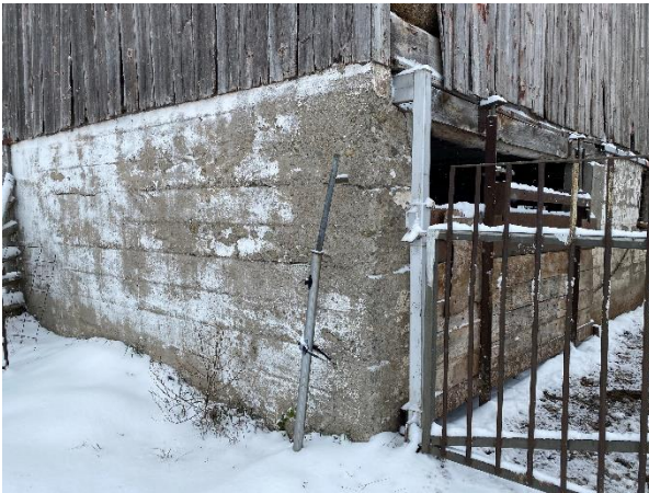
Plate 55: Concrete foundation of Barn No. 2.
