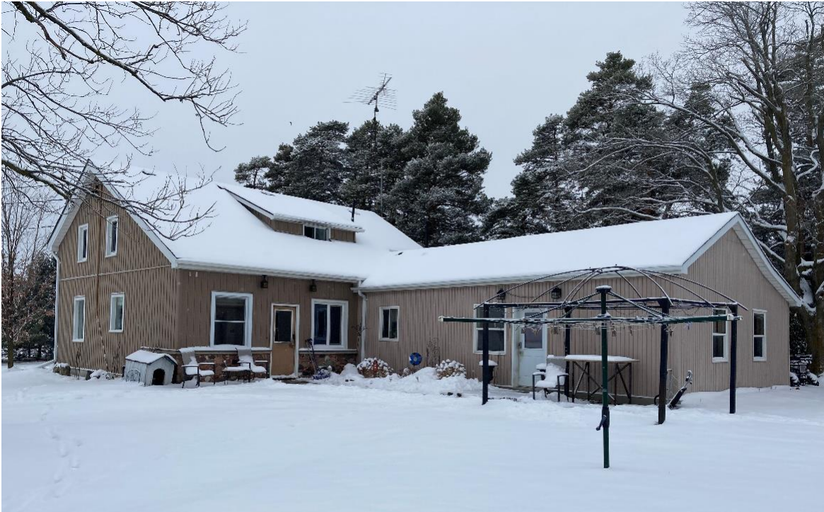
Plate 8: Oblique view of east and south elevations
