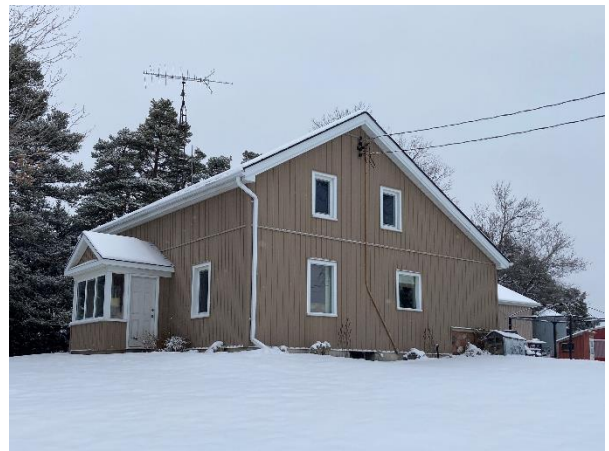
Plate 14: Oblique view of south and west elevations
