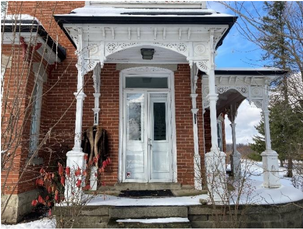
Plate 25: Main entrance porch
