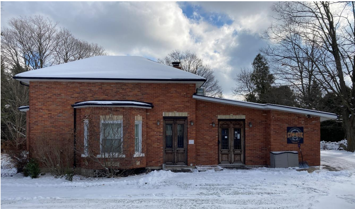
Plate 15: North (rear) elevation
