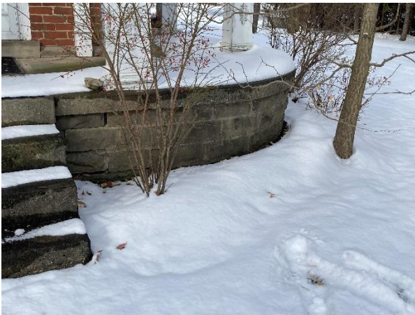
Plate 27: Stone foundation of the front and side porches
