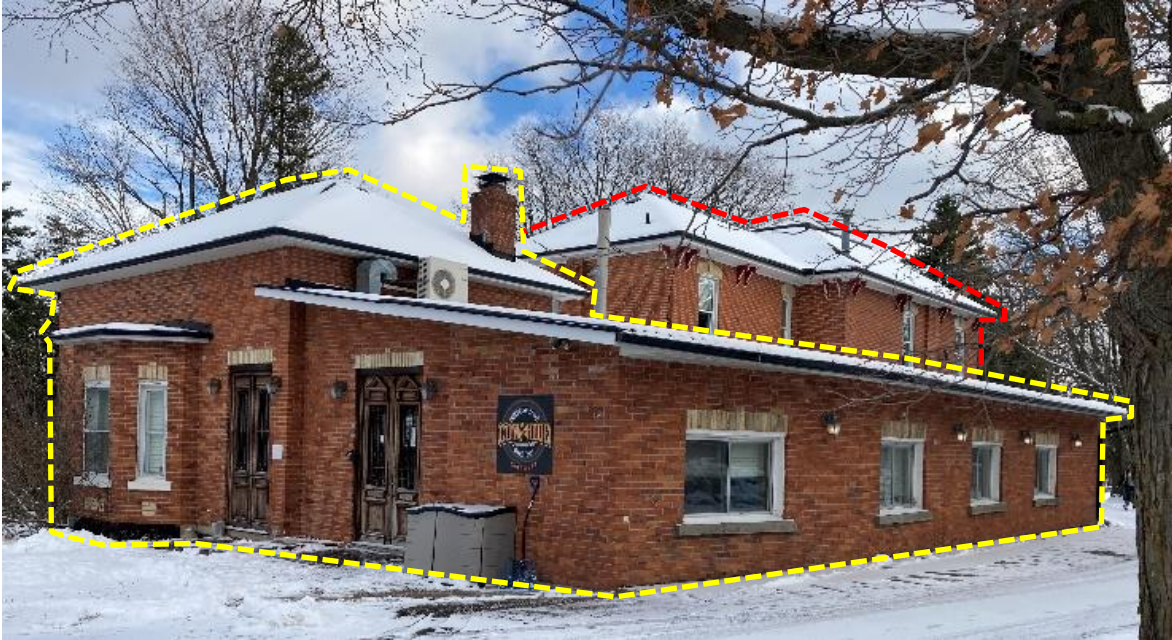
Plate 16: Oblique view of north and west elevations of rear and side additions (outlined in yellow, original main block is outlined in red)
