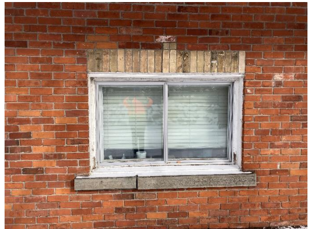
Plate 43: Example of west elevation windows on side addition
