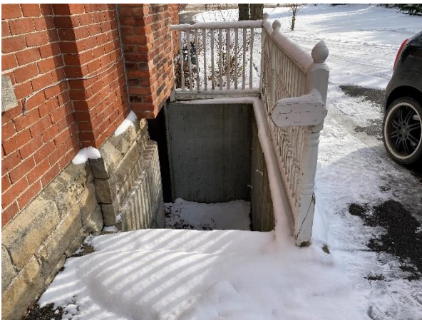
Plate 35: Basement access on west elevation
