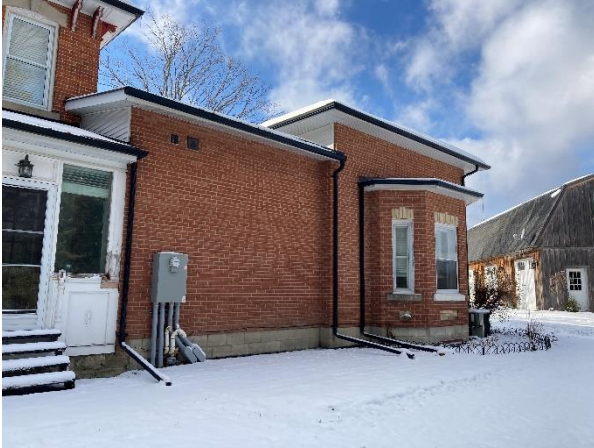
Plate 37: East elevation of rear tail
