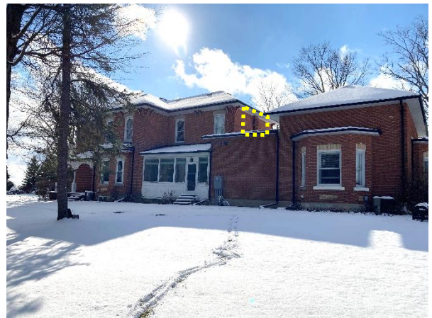
Plate 36: East elevation with former external chimney visible on original main block (highlighted in yellow)
