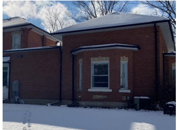
Plate 41: Detail of east elevation bay window
