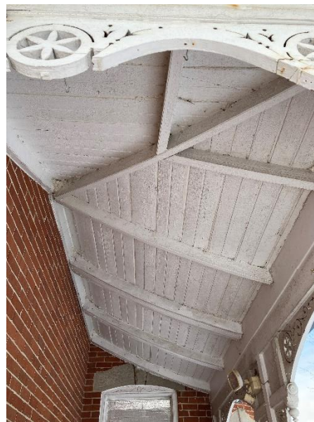
Plate 28: Bellcast roof of the side porch
