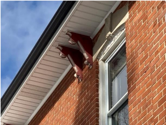
Plate 19: Overhanging eaves and paired bracket detail
