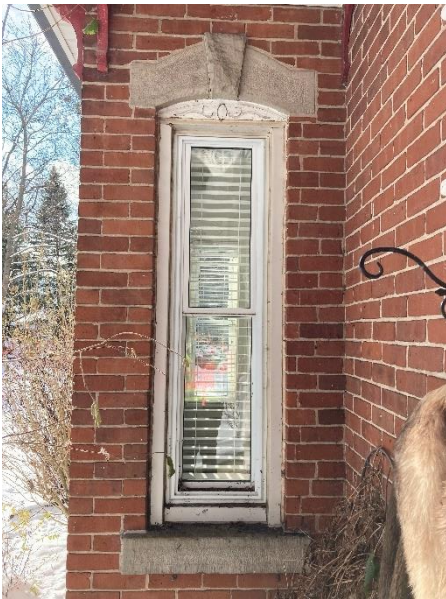
Plate 23: Detail of box bay side windows
