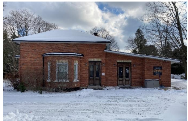
Plate 39: North elevation of rear/side addition
