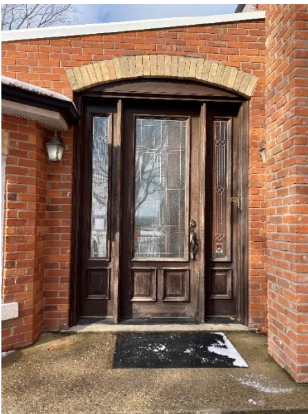
Plate 42: South entrance to side addition
