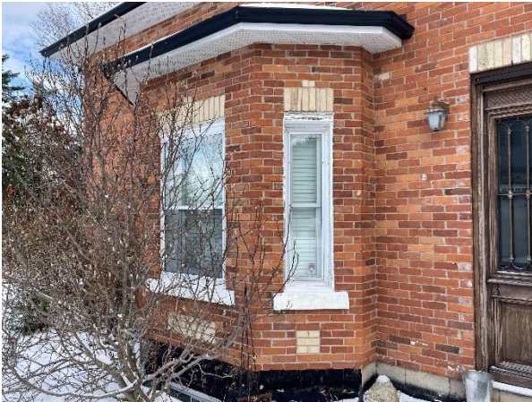
Plate 40: Detail of north elevation bay window
