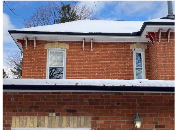
Plate 34: Upper storey windows of main block west elevation showing later replacements of some elements
