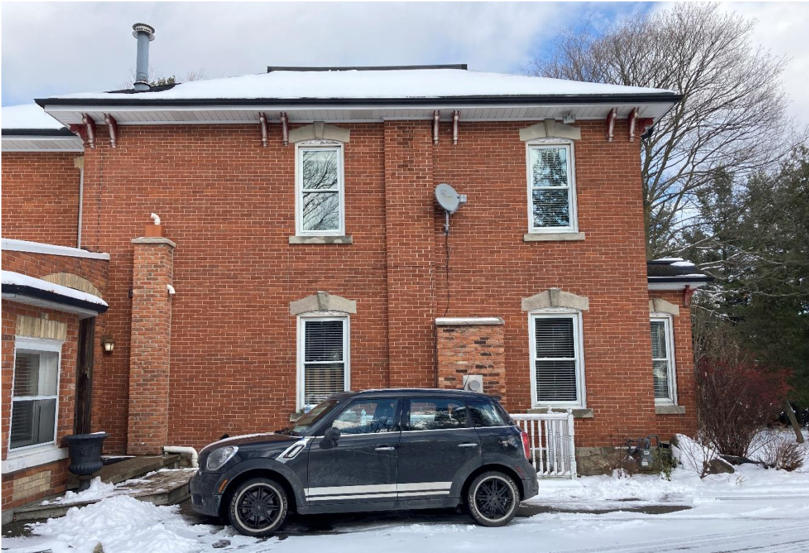
Plate 17: South portion of the west elevation of original main block
