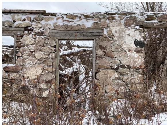
Plate 21: Parged fieldstone wall and doorway
