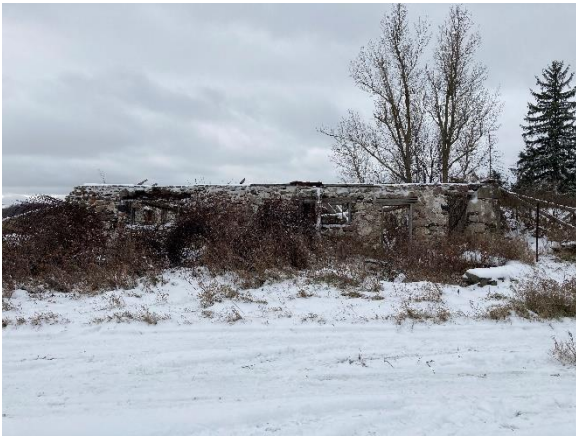
Plate 18: West elevation of Structural Foundation No. 1
