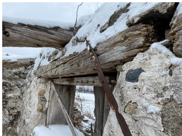
Plate 23: Wood lintel and frame
