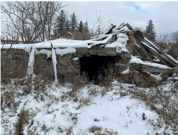
Plate 31: Entrance to below grade cellar
