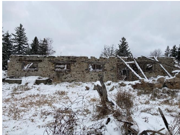
Plate 19: South elevation of Structural Foundation No. 1
