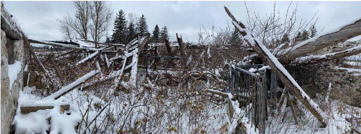
Plate 26: Panoramic photo of Structural Foundation No. 1 interior
