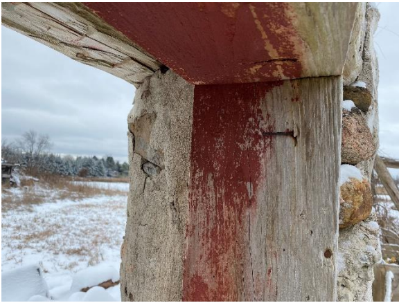
Plate 24: Wood window frame joint
