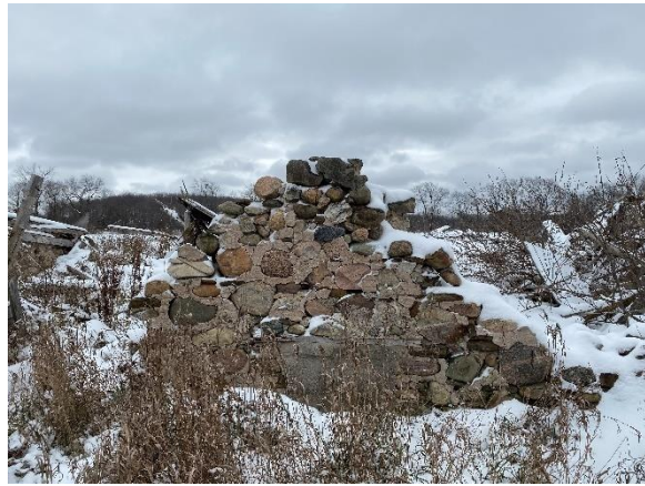
Plate 28: Parged fieldstone walls of Structural Foundation No. 2
