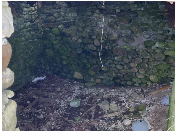
Plate 32: Fieldstone wall of below grade cellar interior
