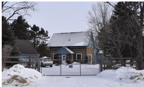
Plate 5: 18309 Mississauga Road (potential built heritage resource)
