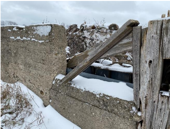
Plate 29: Wood fenestration elements of Structural Foundation No. 2
