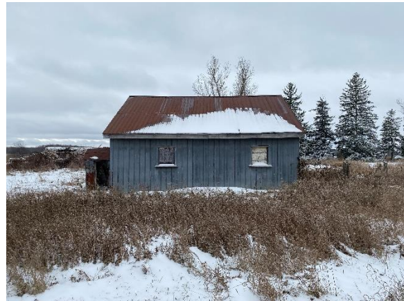
Plate 17: East elevation of outbuilding
