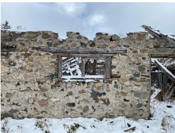
Plate 22: Parged fieldstone wall and window
