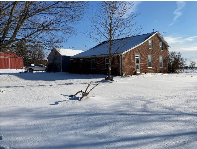
Plate 28: Oblique view of north and west elevations of residence
