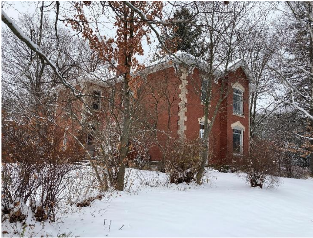
Plate 2: Oblique view of east and north elevations of residence
