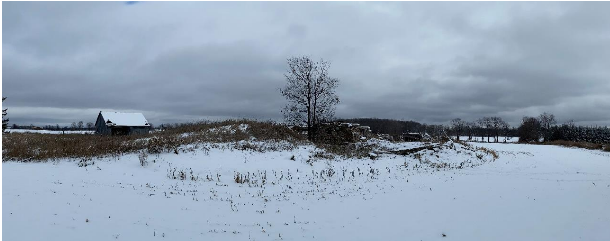
Plate 7: View across extant outbuilding and ruins at 1055 Charleston Sideroad, facing northeast
