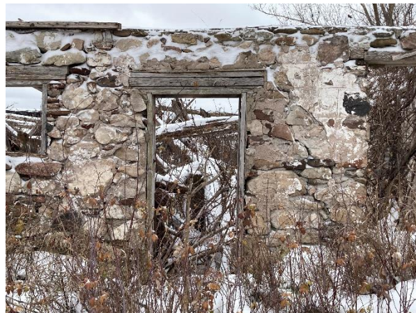
Plate 9: Detail showing wood doorframe and window frames and parged fieldstone foundations
