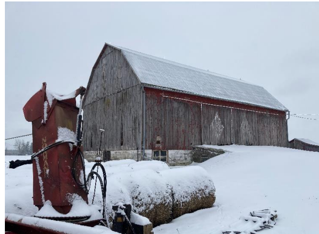
Plate 24: Oblique view of east and north elevations of Barn No. 2.
