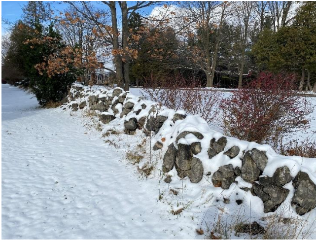
Plate 19: Low fieldstone wall along the southwest side of the property
