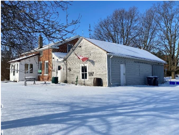
Plate 30: Rear addition, facing southwest
