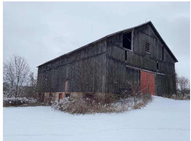
Plate 5: North and west elevations of the barn
