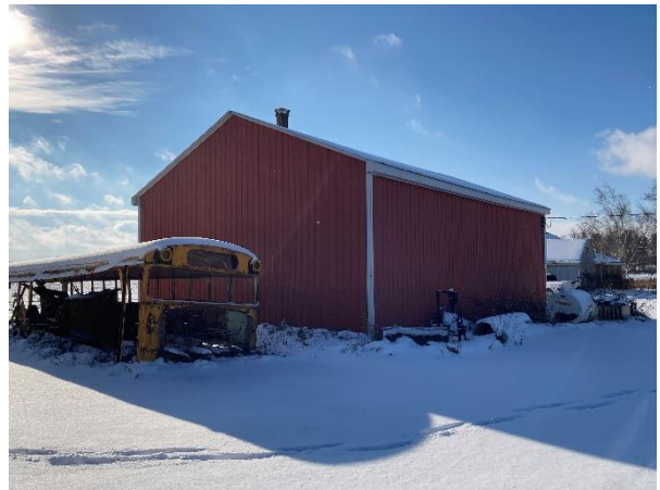
Plate 33: East and north elevations of Outbuilding No. 2
