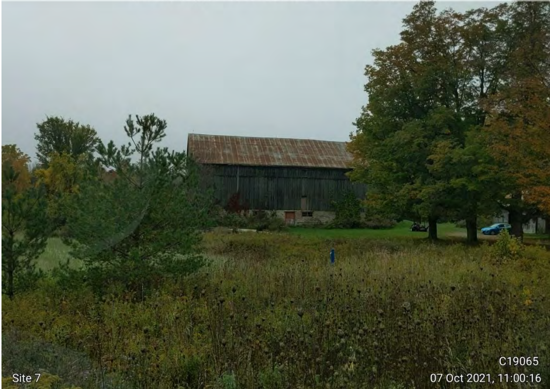
Photo 5: View of Site 7 bank barn within PSA.
