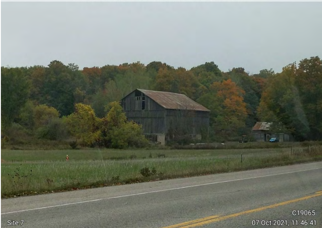
Photo 6: View of Site 7 bank barn and wood shed within PSA.
