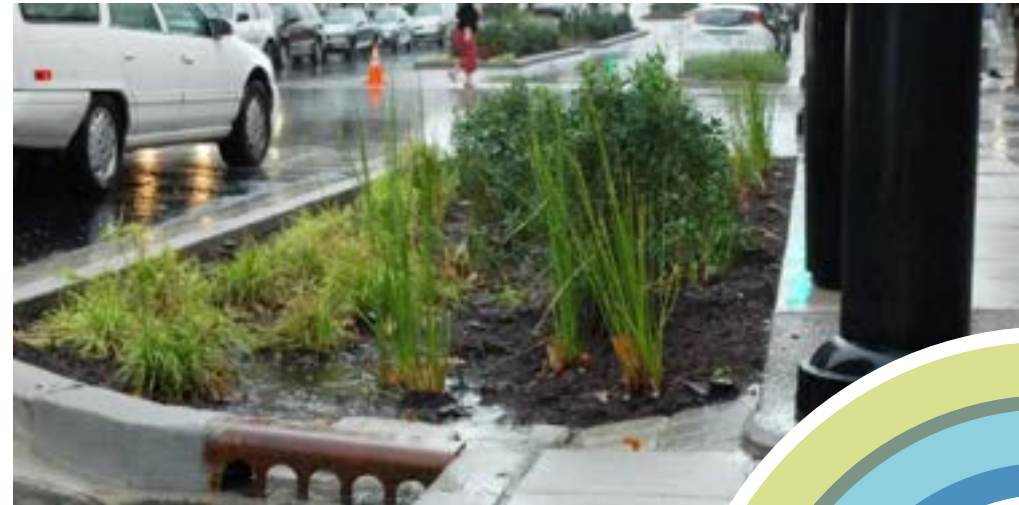
Street Level Stormwater Retention
