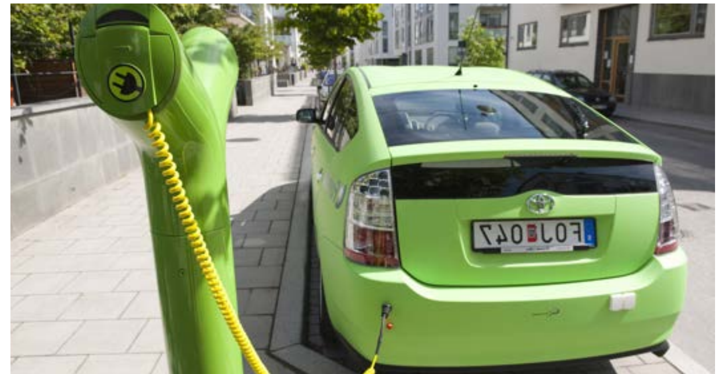
Electrical Vehicle Charging
