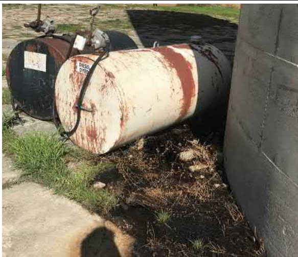
Diesel ASTs - Petroleum sheen and odour under beige tank
