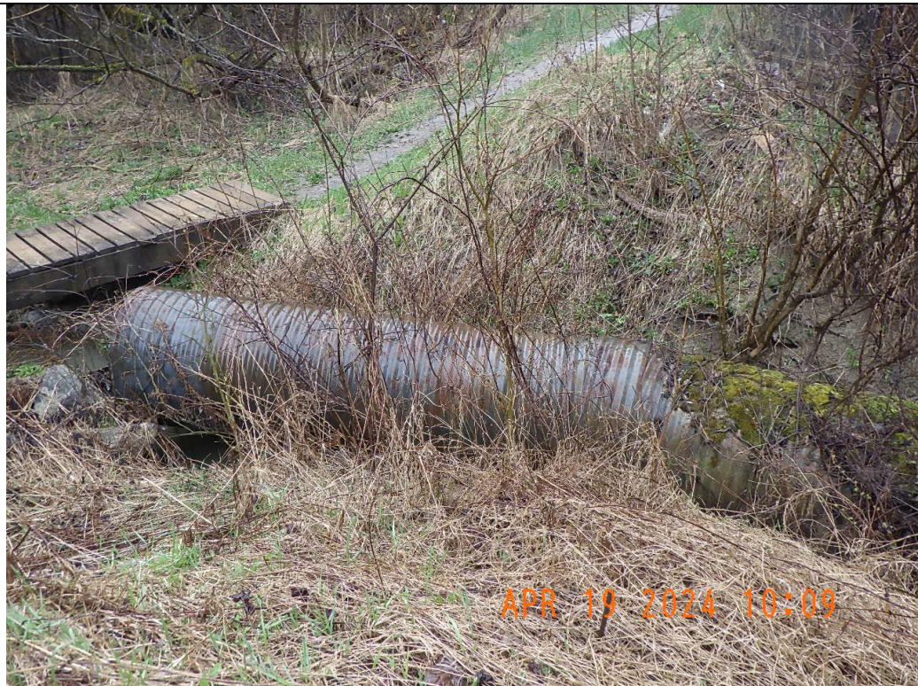
A previously buried culvert was entirely exposed upstream a small crossing.
