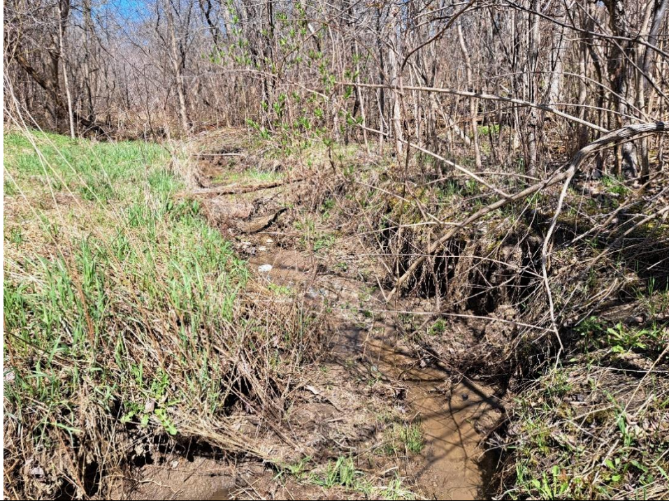
In the upstream portion of the reach erosion and undercutting was commonly observed. Undercuts were measured up to 0.48 m.
