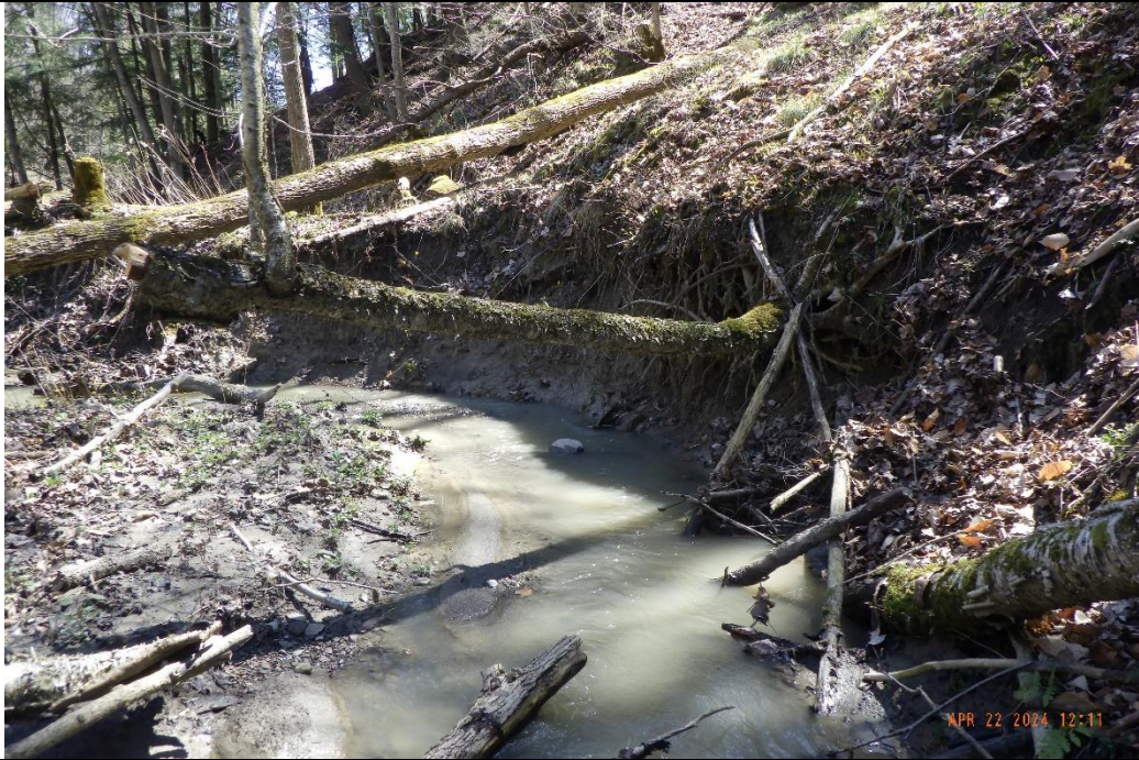
Valley wall contact occurred in multiple locations along the reach. The reach has steep banks, erosion, and undercuts measuring up to 0.5 m.
