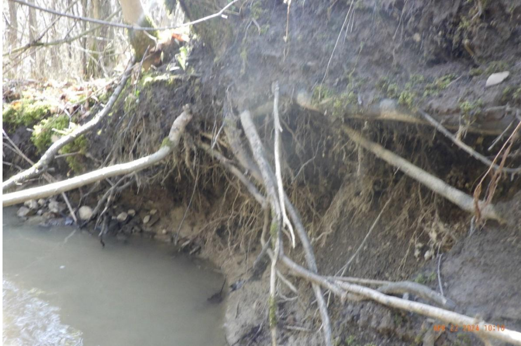
Undercuts were observed in various locations along the reach and measured up to 0.78 m.
