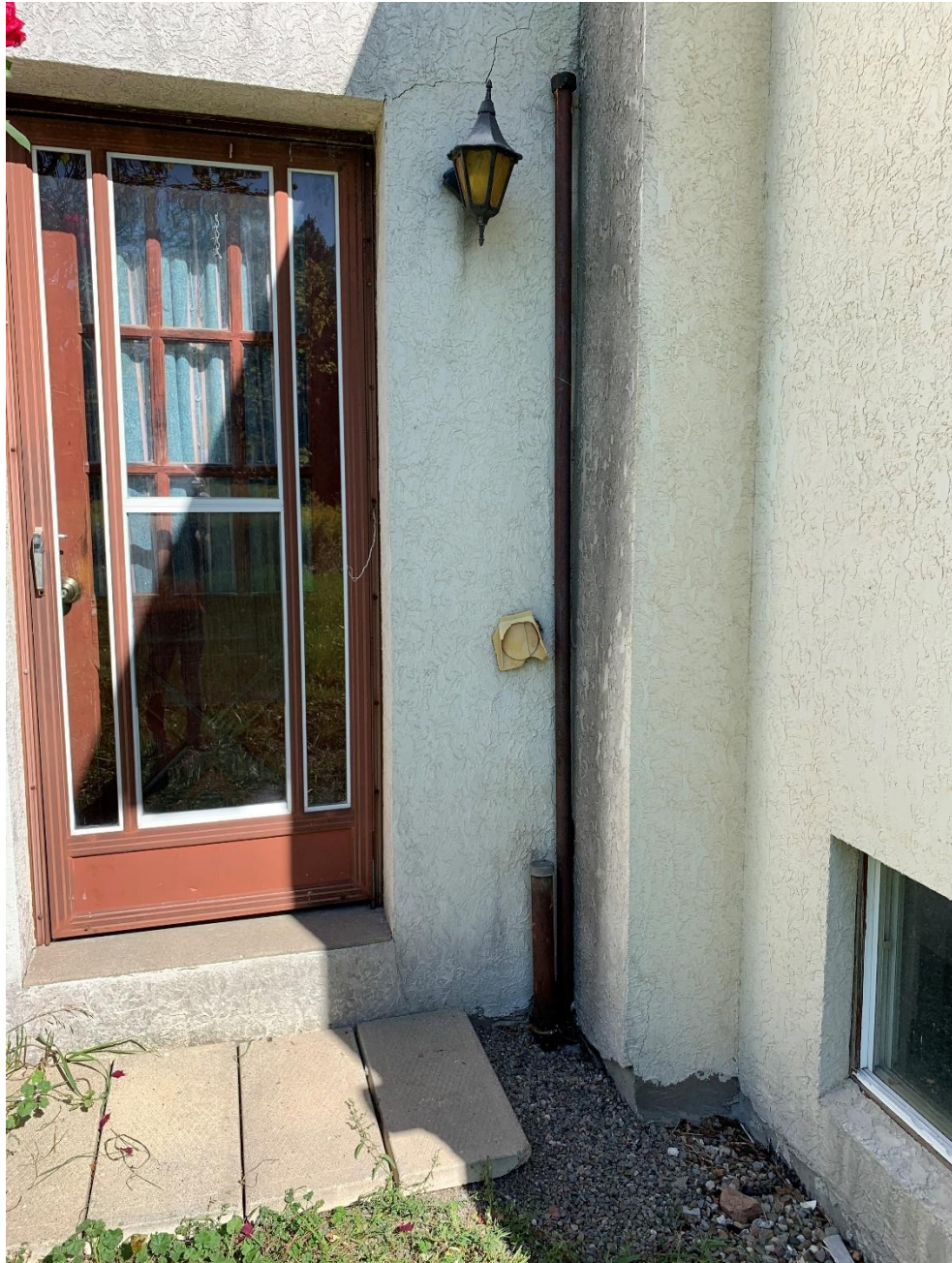
Photo 5: Closer View of the fill-vent pipes of the AST located inside the basement (also shown in Photo 3)
