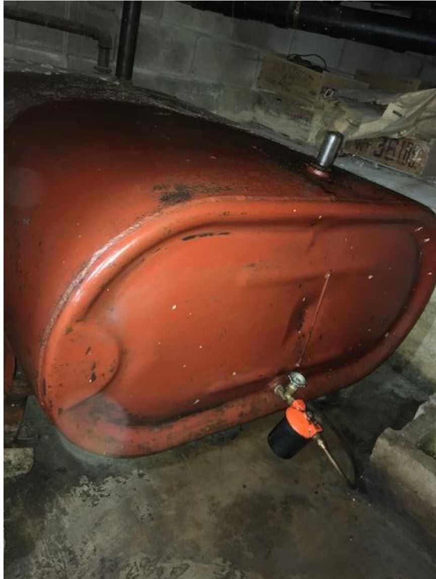
Photo 6: View of the AST located inside the basement of the residential Dwelling
