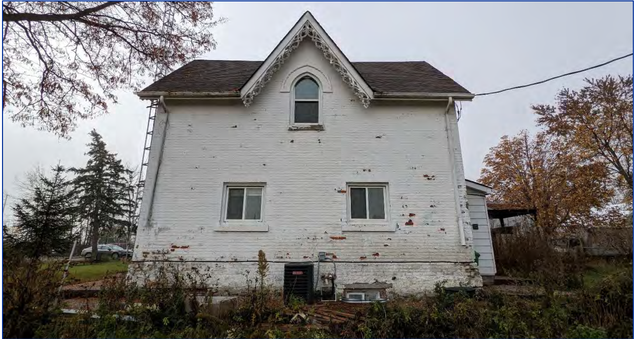
Photo 19: View of east side elevation, looking west.
