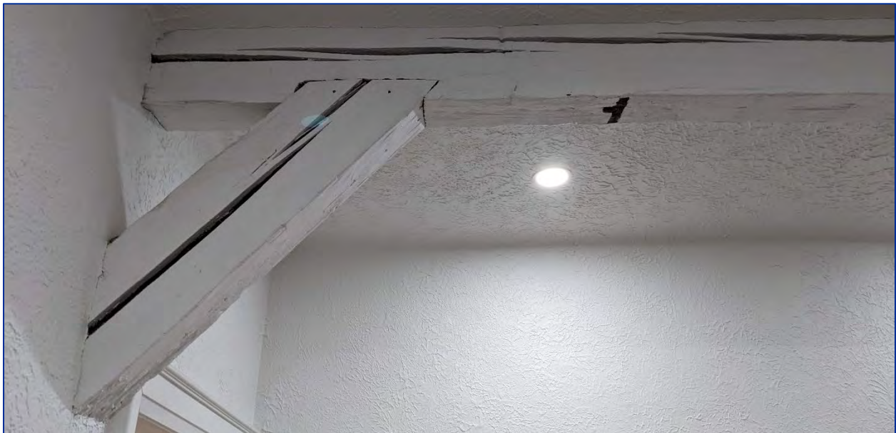
Photo 32: View of the mortise-tenon brackets.
