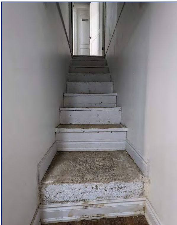
Photo 30: View of the staircase to the basement.
