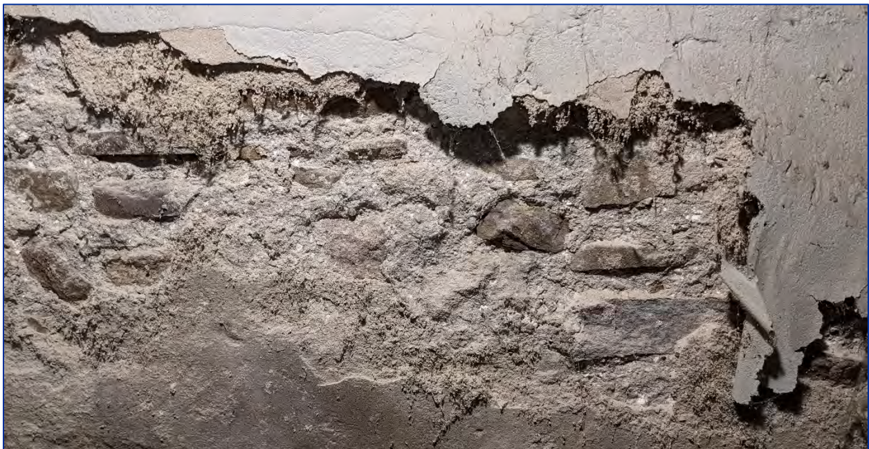
Photo 28: View of the fieldstone foundation, parged with cement.
