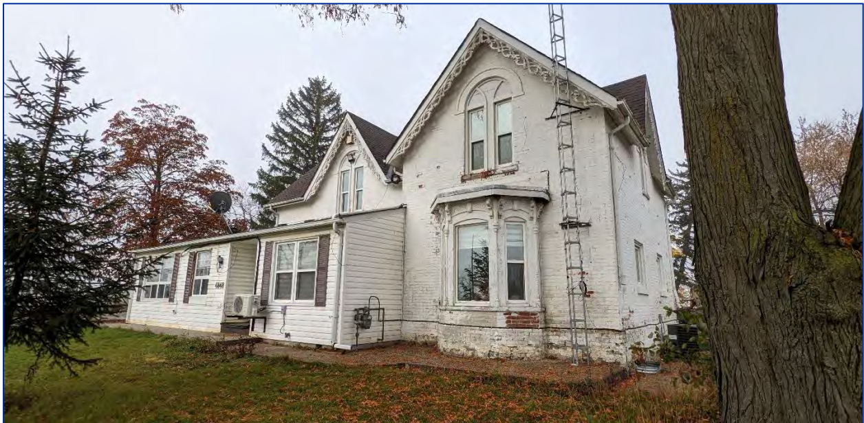
Photo 20: View of front elevation and enclosed porch, looking northwest.
