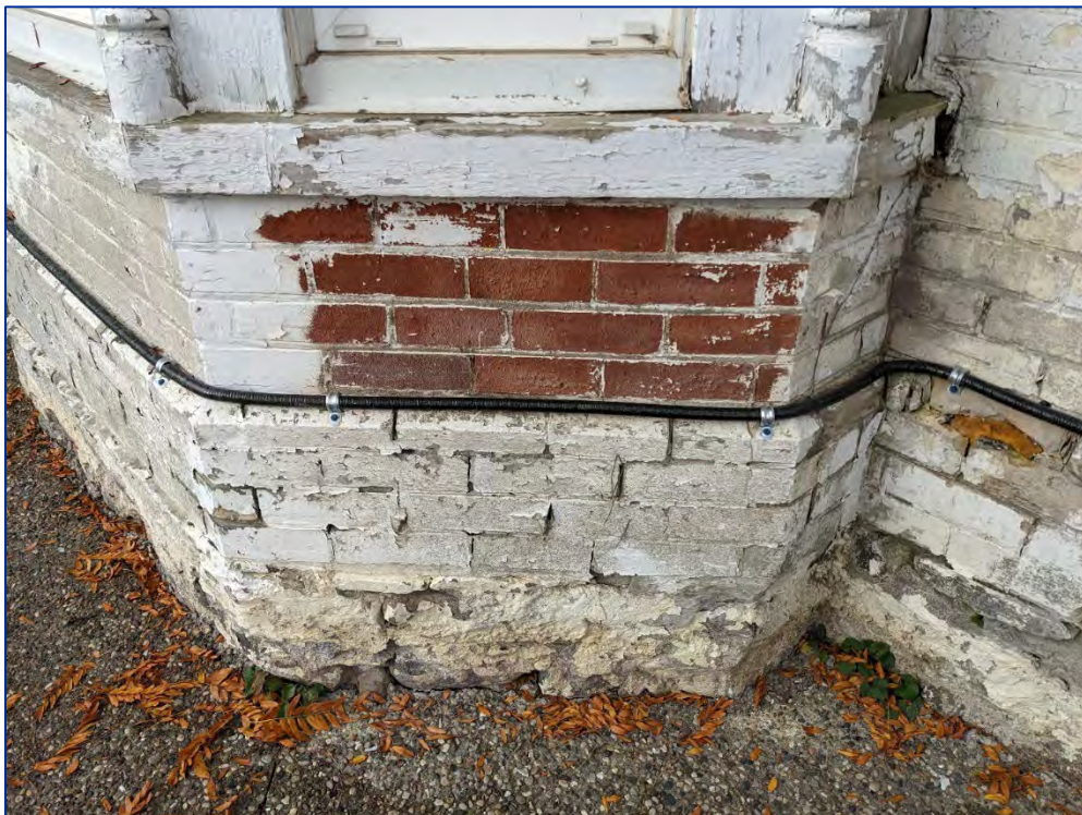
Photo 24: View of field stone foundation and red brick wall.
