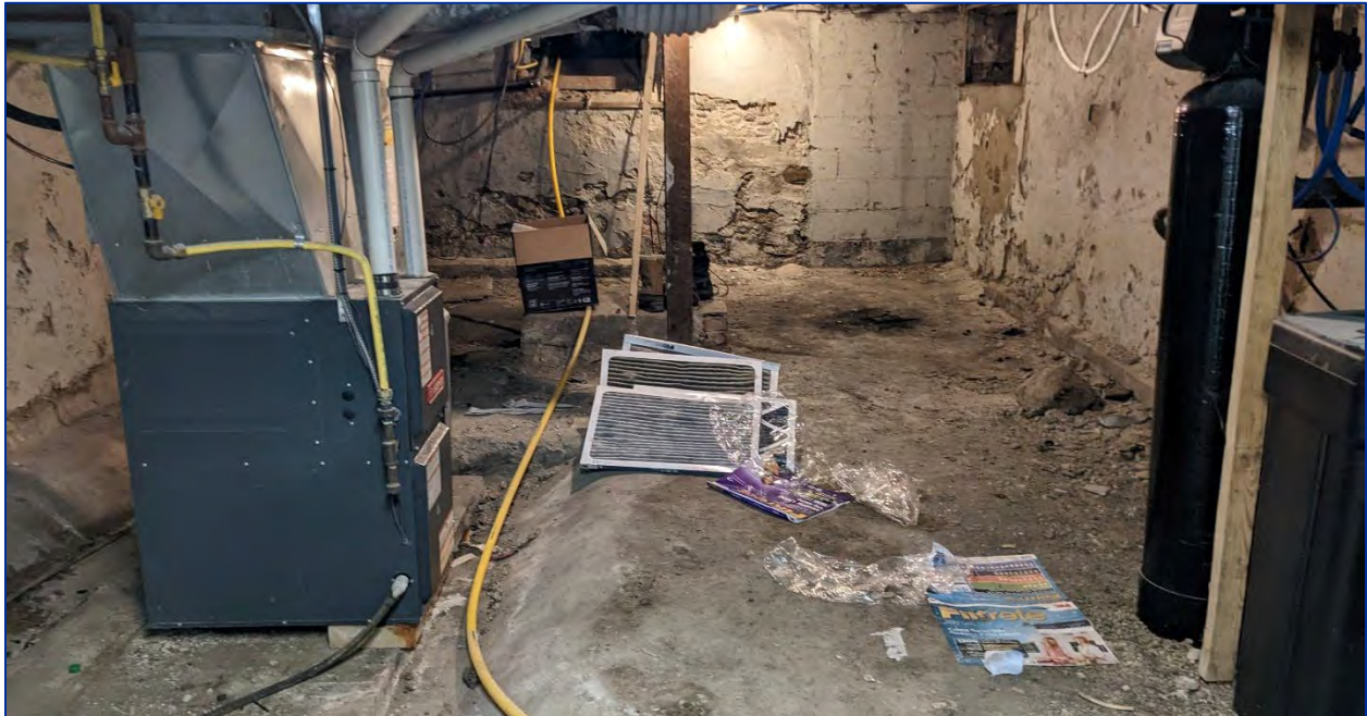
Photo 27: View of the basement.
