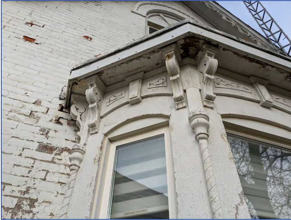
Photo 21: View of decorative wood brackets, window surrounds, keystones, and rope columns.
