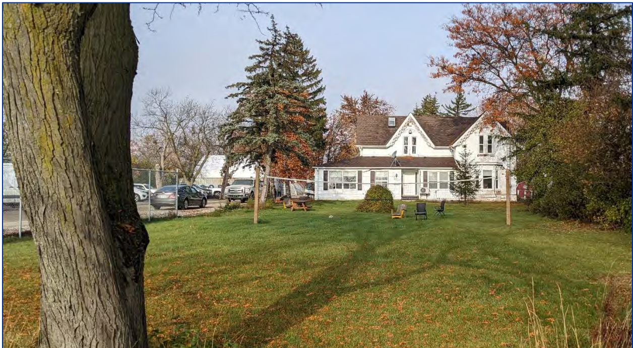
Photo 16: View of front elevation, front yard, and driveway, looking north.
