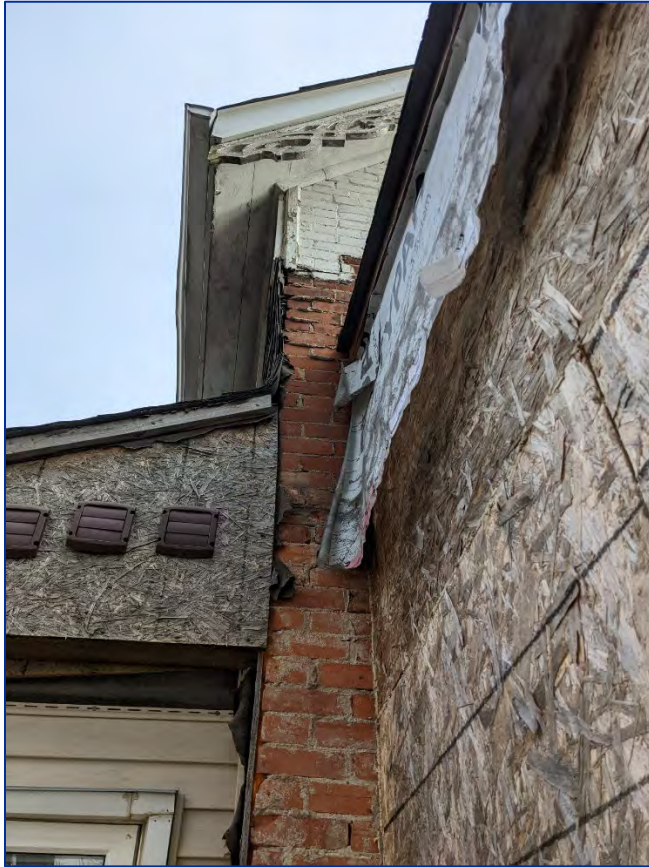
Photo 25: View of red brick and bargeboard.
