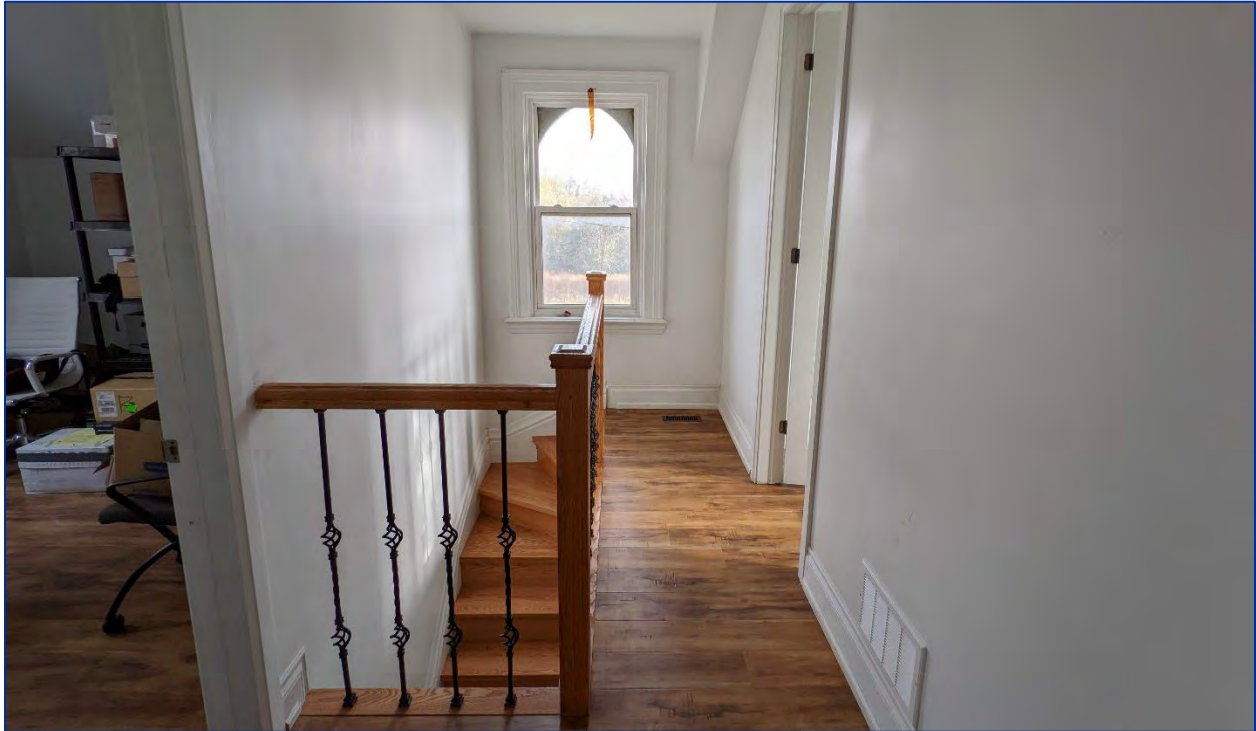
Photo 35: View of a hallway and staircase.
