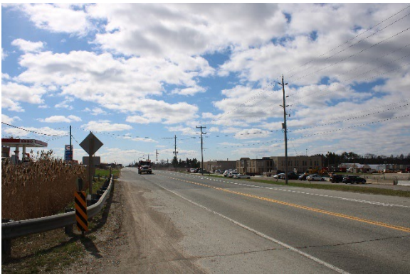
Photo 5: Highway 50, looking south
