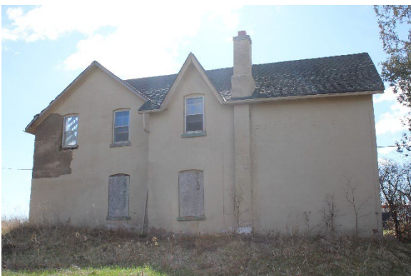
Photo 18: North façade, looking south
