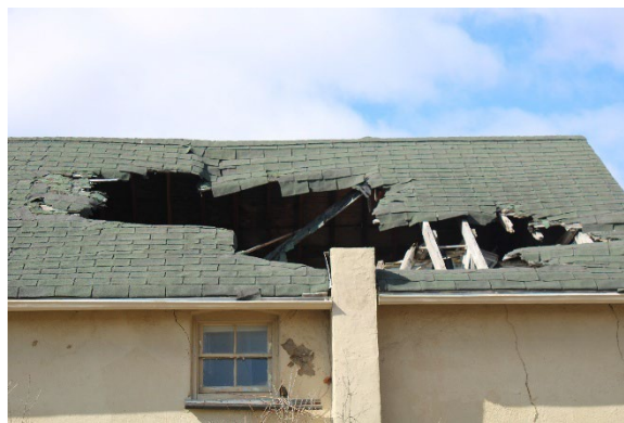
Photo 17: East façade roof, looking west
