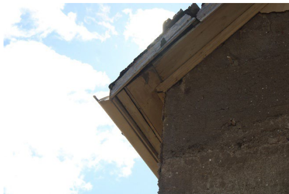
Photo 11: Detail of wood soffit
