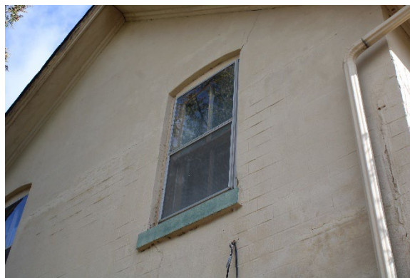
Photo 23: Second storey window on west façade, looking northeast
