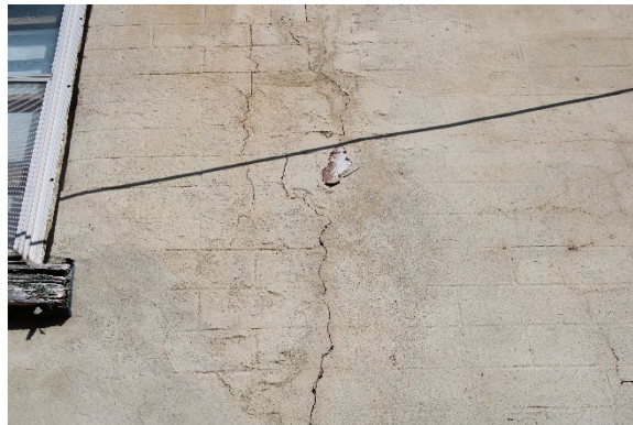
Photo 9: Detail of exterior cladding
