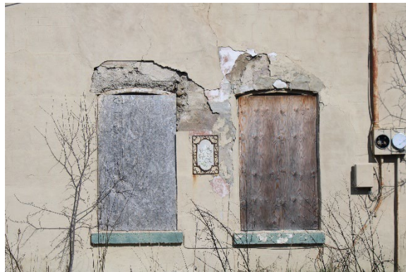
Photo 15: First storey windows on south façade, looking north
