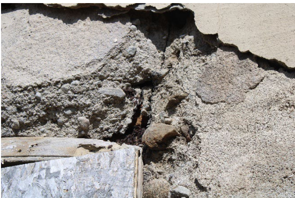
Photo 10: Detail of concrete cladding
