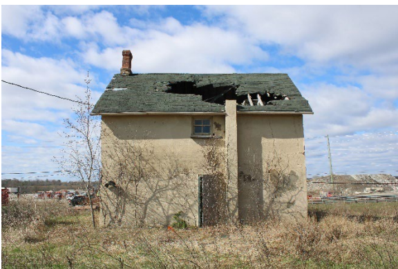
Photo 16: East façade, looking west
