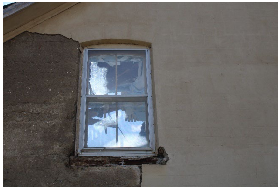
Photo 21: Second storey window on north façade, looking south
