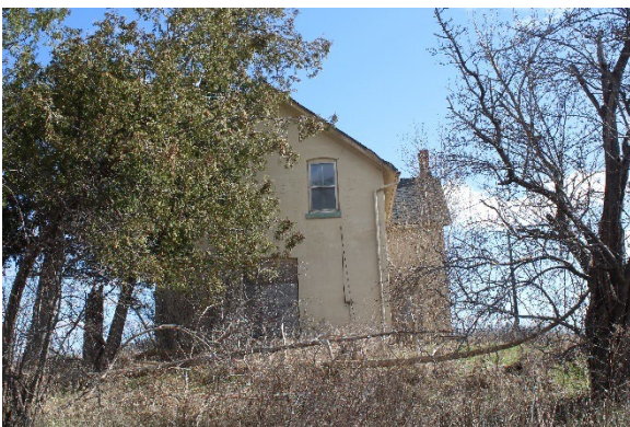
Photo 22: West façade, looking east
