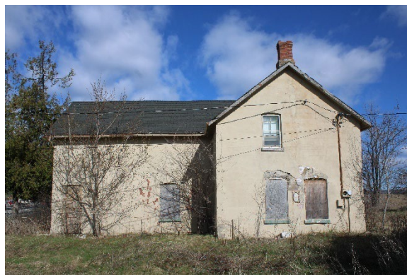
Photo 13: South façade, looking north
