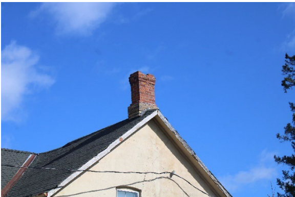
Photo 14: South façade chimney, looking north
