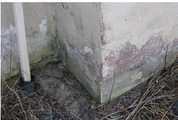
Photo 12: Detail of parged concrete foundation
