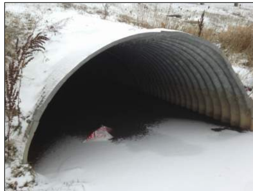
Figure 29: Existing Elliptical Culvert at Mayfield Rd and Maisonneuve Blvd
