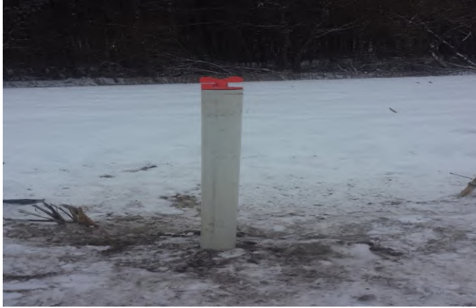
Photograph 4: View of the restored PVC pipe
