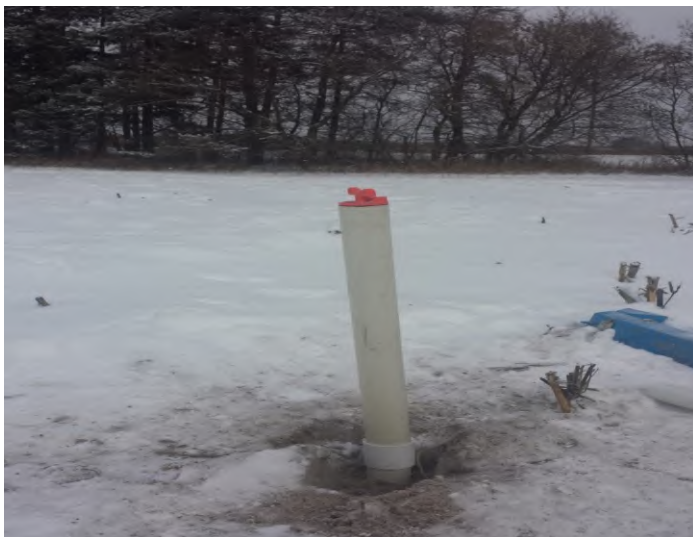
Photograph 3: View of the restored PVC pipe. Due to the hard ground surface, the protective casing could not be set in place.
