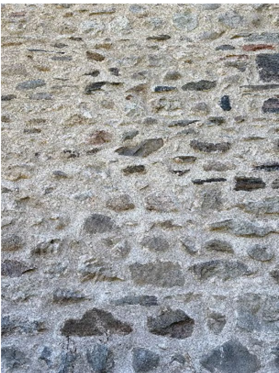
Figure 16: Detail of random masonry on side façade, 2025. Town of Caledon
