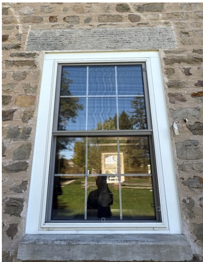
Figure 12: Detail of window opening on front façade showing tooled cut stone lintel and modern concrete lug sill, 2025. Town of Caledon
