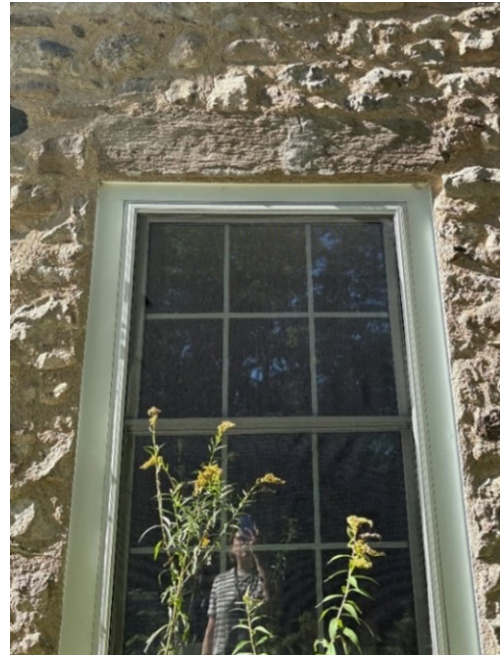
Figure 13: Detail of side façade window openings showing rough cut stone lintels in contrasting colours, 2025. Town of Caledon
