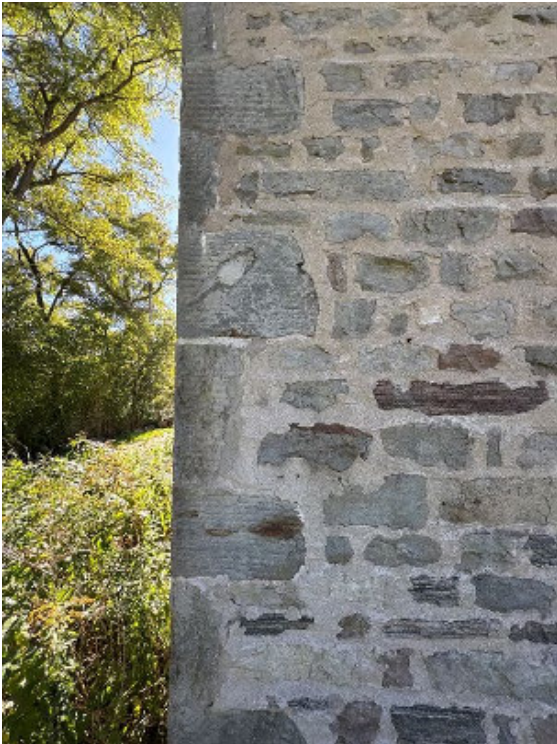
Figure 15: Detail of coursed masonry and tooled stone quoining on front façade, 2025. Town of Caledon
