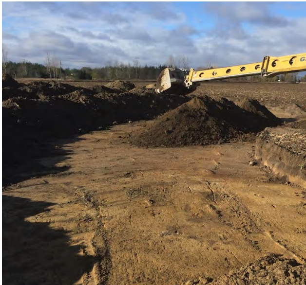
Plate 11: Contrast between subsoil and topsoil during mechanical stripping.
