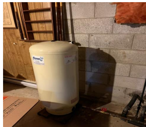
Picture 6: View of the water heater tank in basement of residential home, facing northwest.
