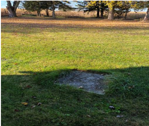
Picture 13: View of the septic tank, located in the backyard of property, facing west.
