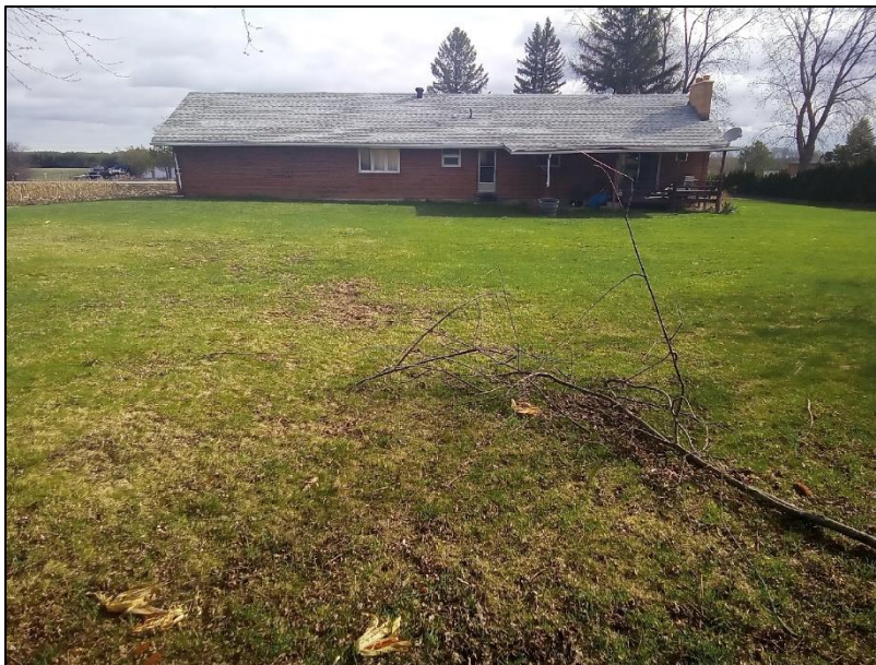
Image 2: View of the rear lawn and the house in the project area.
