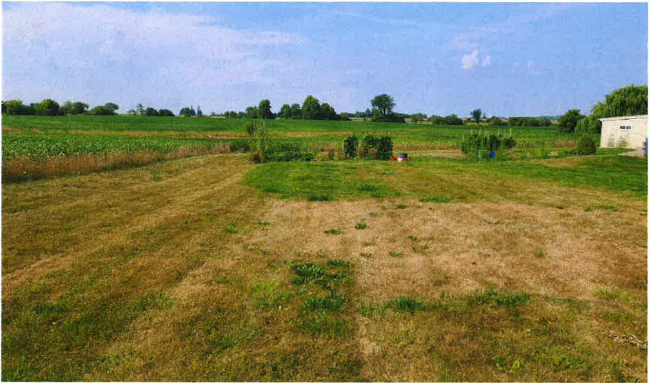
General view of septic system and detached garage at 14166 Humber Station Road (looking west)
