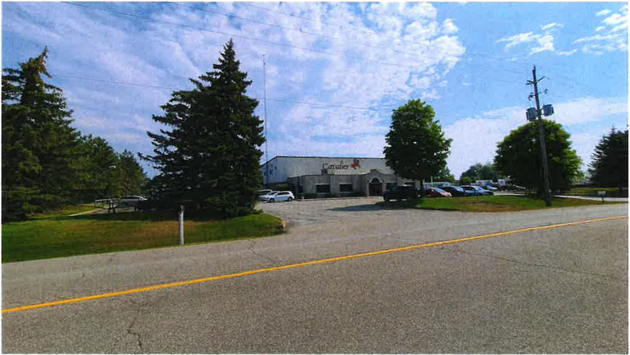
General view of the adjacent Road to the east of the subject site (looking east)
