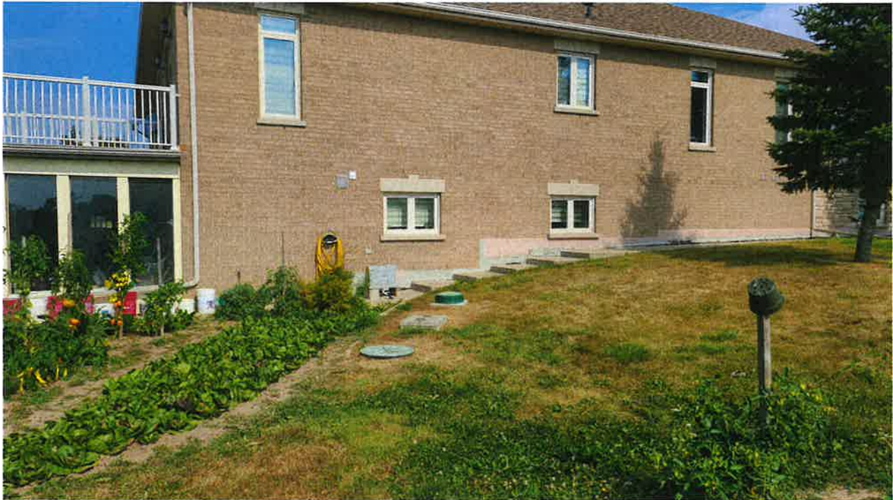
Southeastern portion of house at 14166 Humber Station Road (looking northeast)
