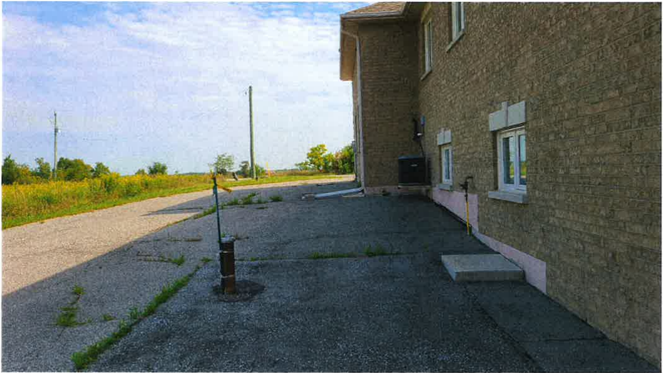
Water well located to the northwest of the house at 14166 Humber Station Road (looking north)
