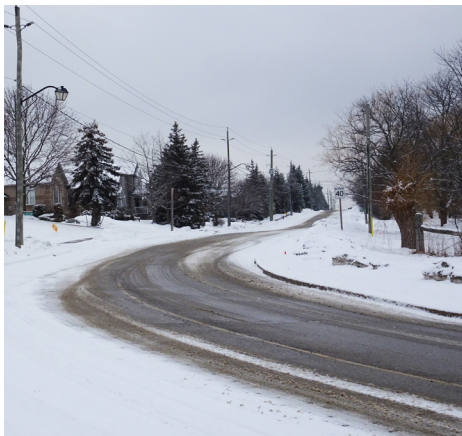
Figure 22. Nunnville Road looking north
