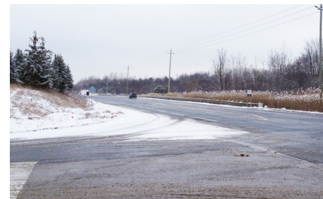
Figure 11. Albion Vaughan Road, looking north
