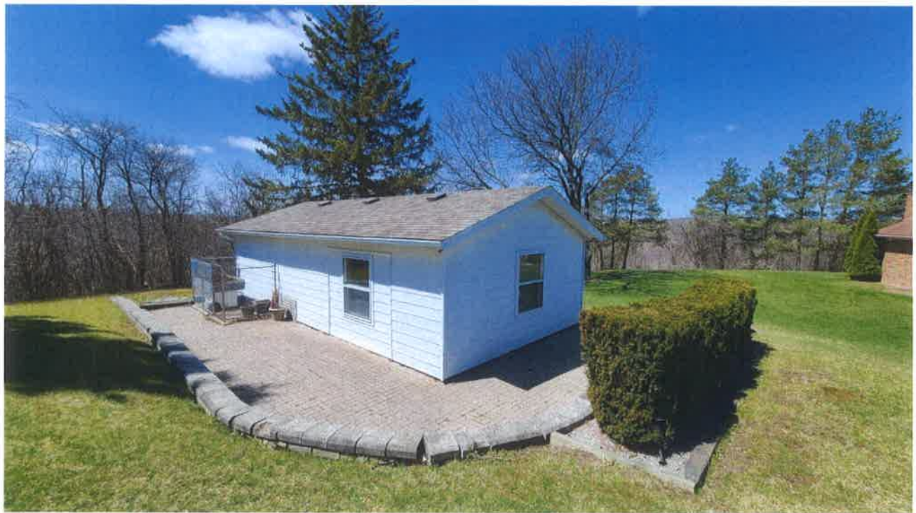
General view of detached garage at south west corner of subject site (looking west)
