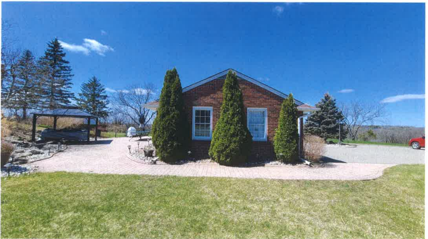
General view of attached garage (looking south)
