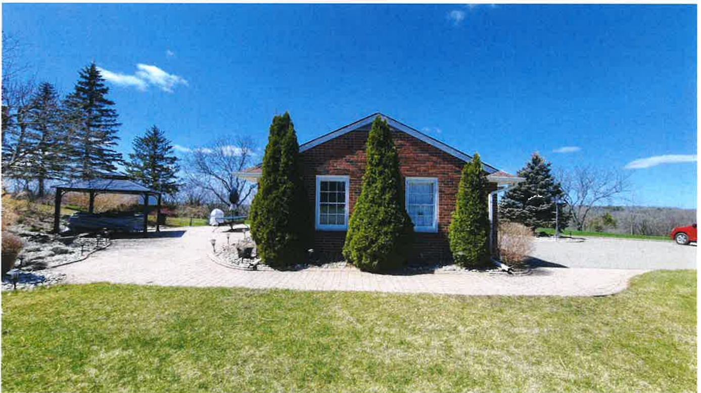
General view of attached garage (looking south)
