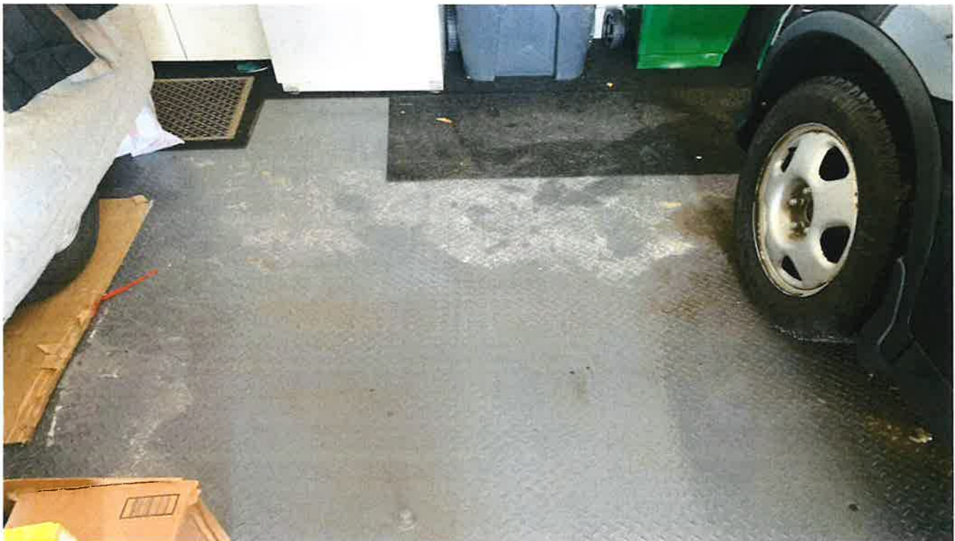
General view of garage floor attached to residential building
