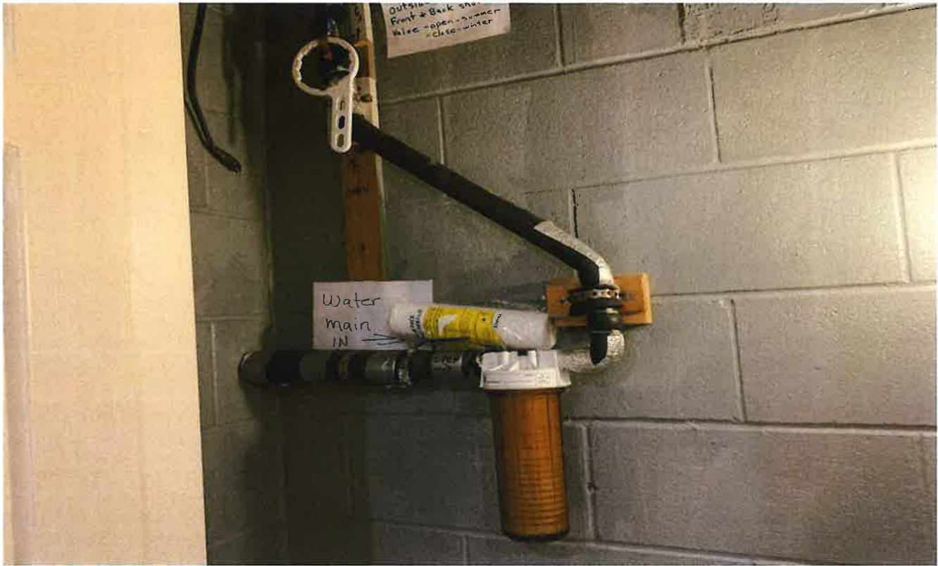
General view of water main in basement
