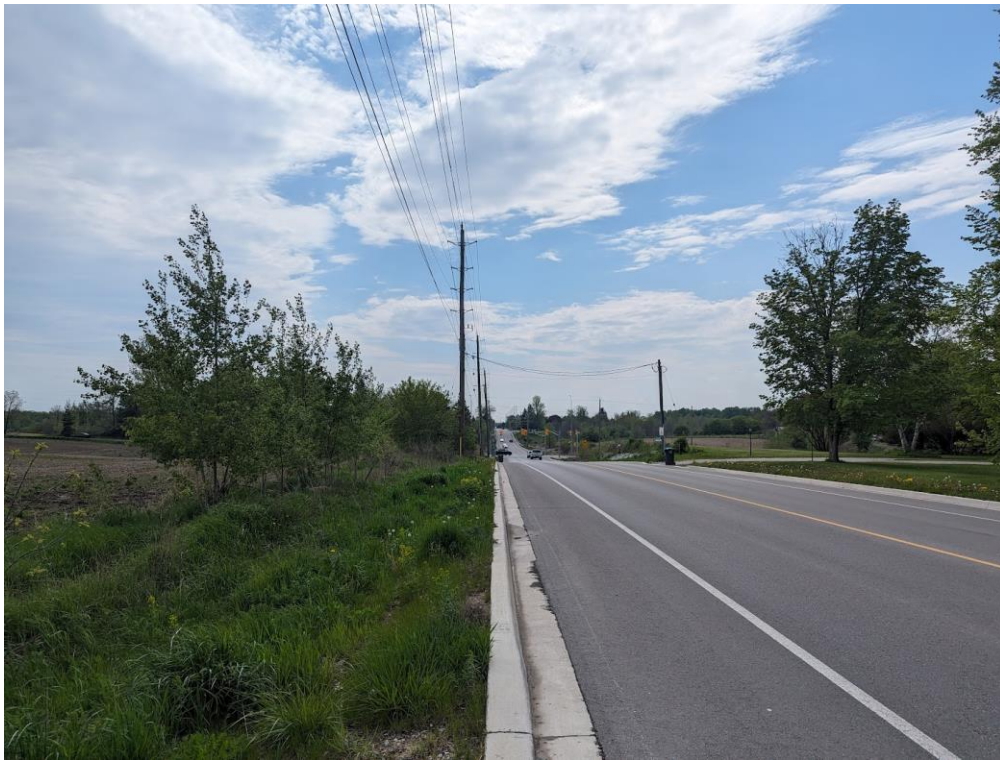
STREET 'B' AT OLD SCHOOL ROAD – FACING WEST
