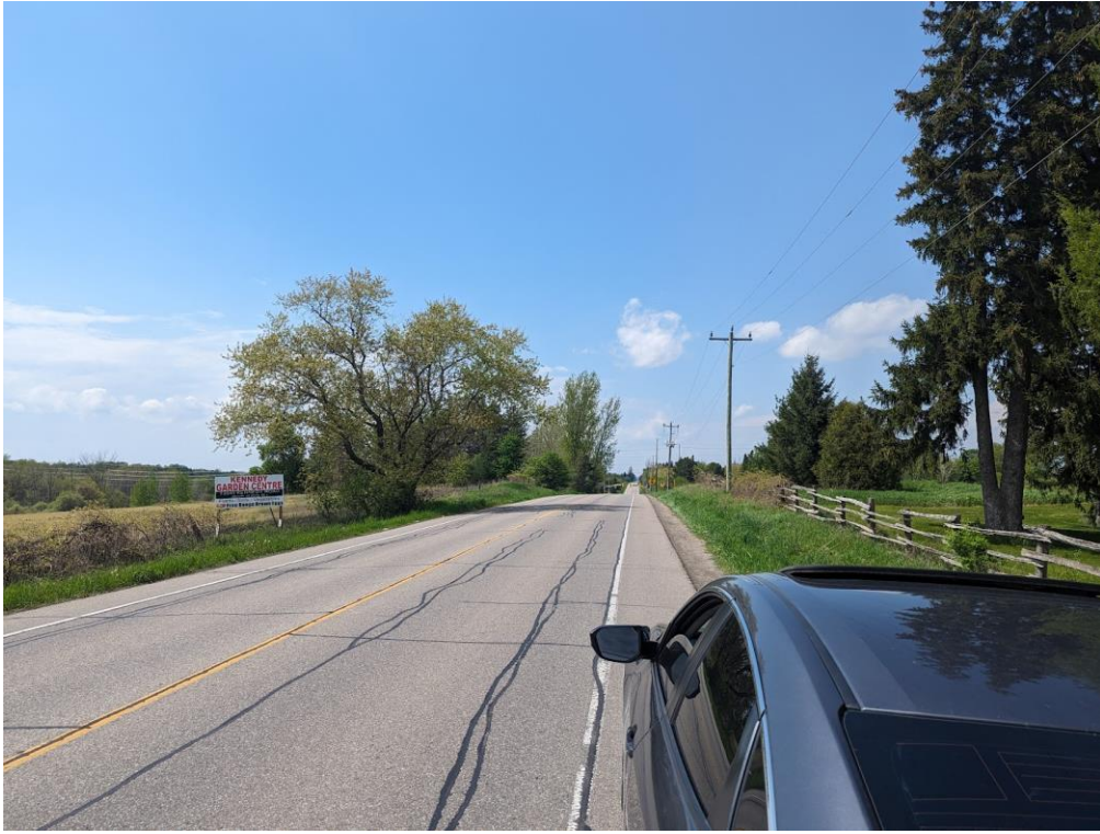
STREET 'A'/PROPOSED COLLECTOR ROAD AT KENNEDY ROAD – FACING NORTH
