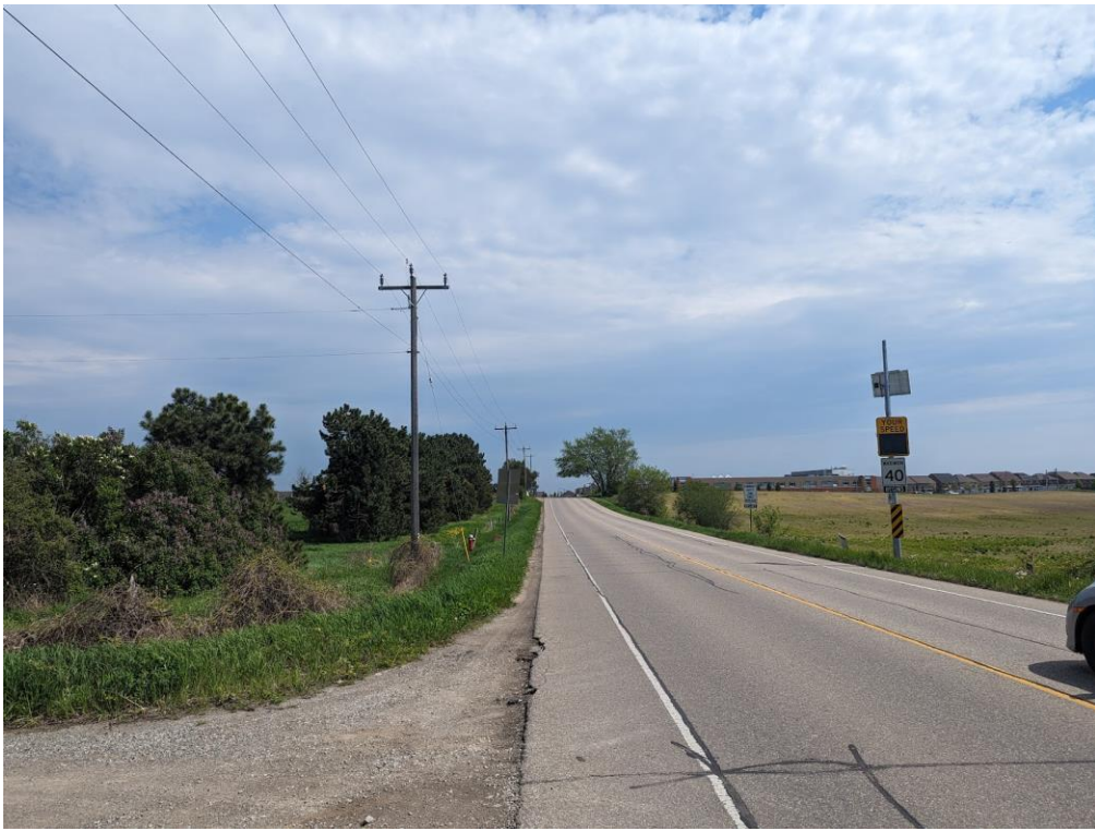
STREET 'A'/PROPOSED COLLECTOR ROAD AT KENNEDY ROAD – FACING SOUTH
