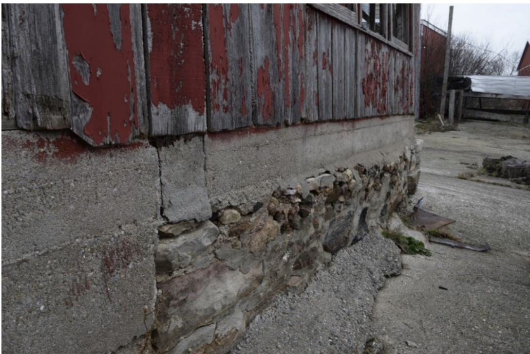
Figure 82: Poor condition of foundation of barn with multiple concrete repair attempts visible
