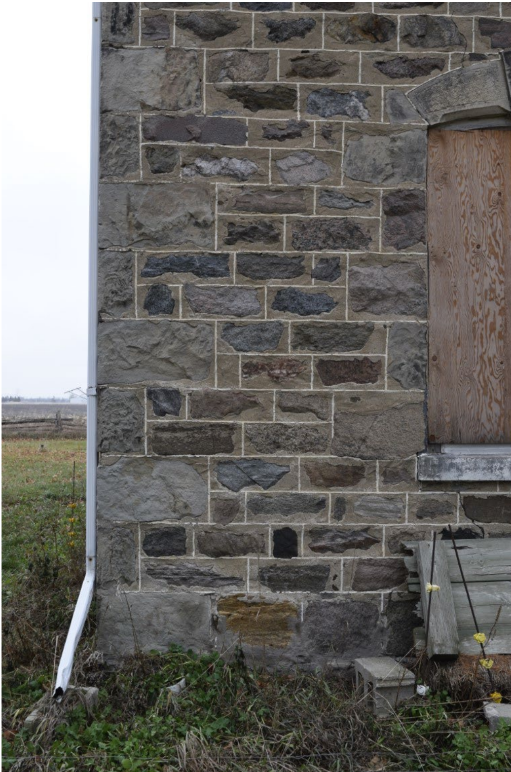
Figure 29: Use of limestone quoining accents at corners and at structural openings on front facade
