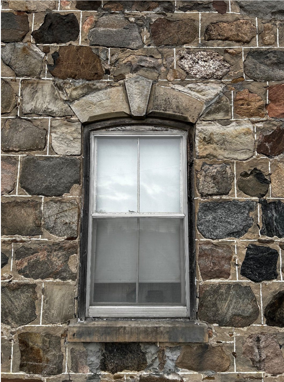
Figure 22: Typical original two over two sash window with original exterior storm, this example is outfitted with a later aluminum exterior storm window
