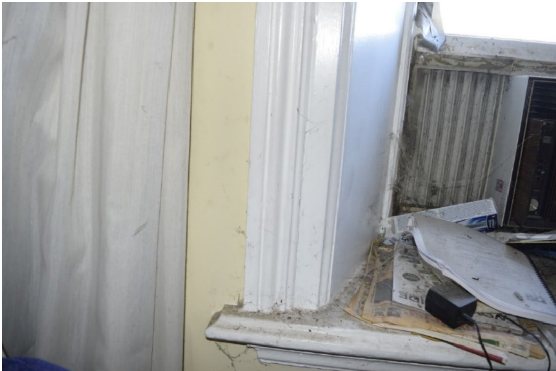
Figure 57: Non-original window trim used in main room first floor, similar to original but not original
