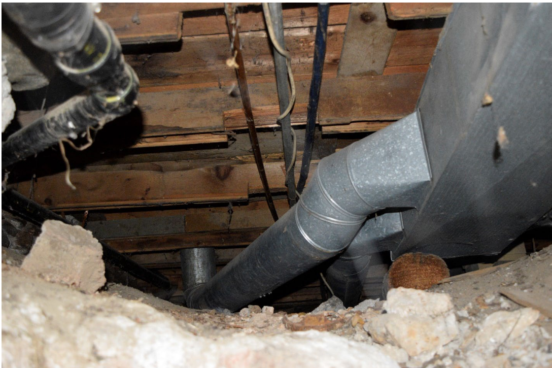
Figure 47: Floor joists under rear wing as viewed through the hole in the field stone foundation to accommodate HVAC system
