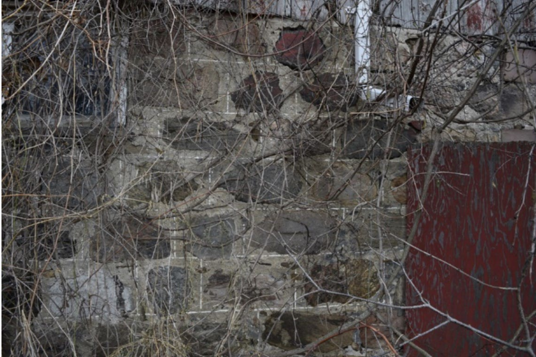
Figure 73: Foundation of bank barn, displaying the same finish as the walls of the residence
