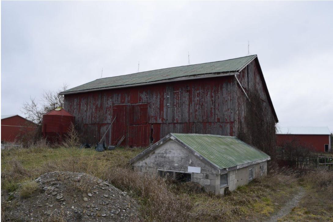
Figure 65: 1885 bank barn with semi subterranean concrete block milk house in foreground
