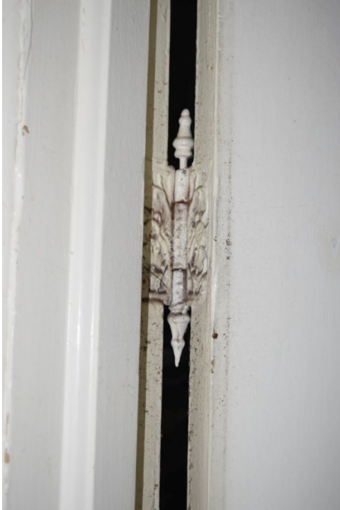
Figure 60: Example of original door hinges with cast designs
