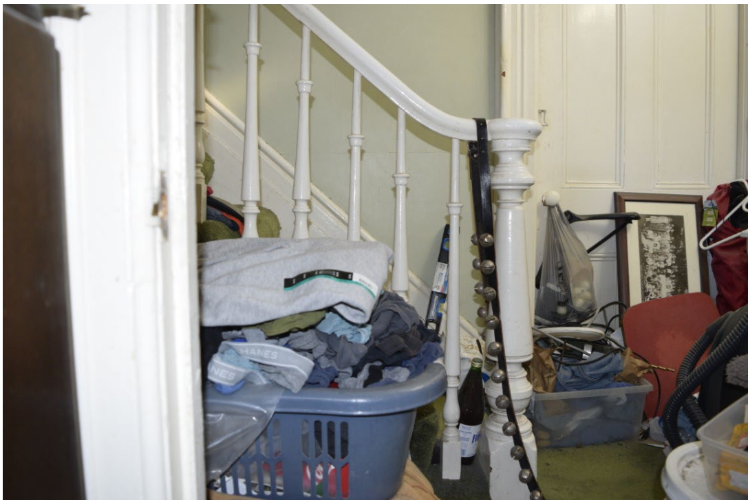
Figure 35: Original newel post and balustrade located inside front door
