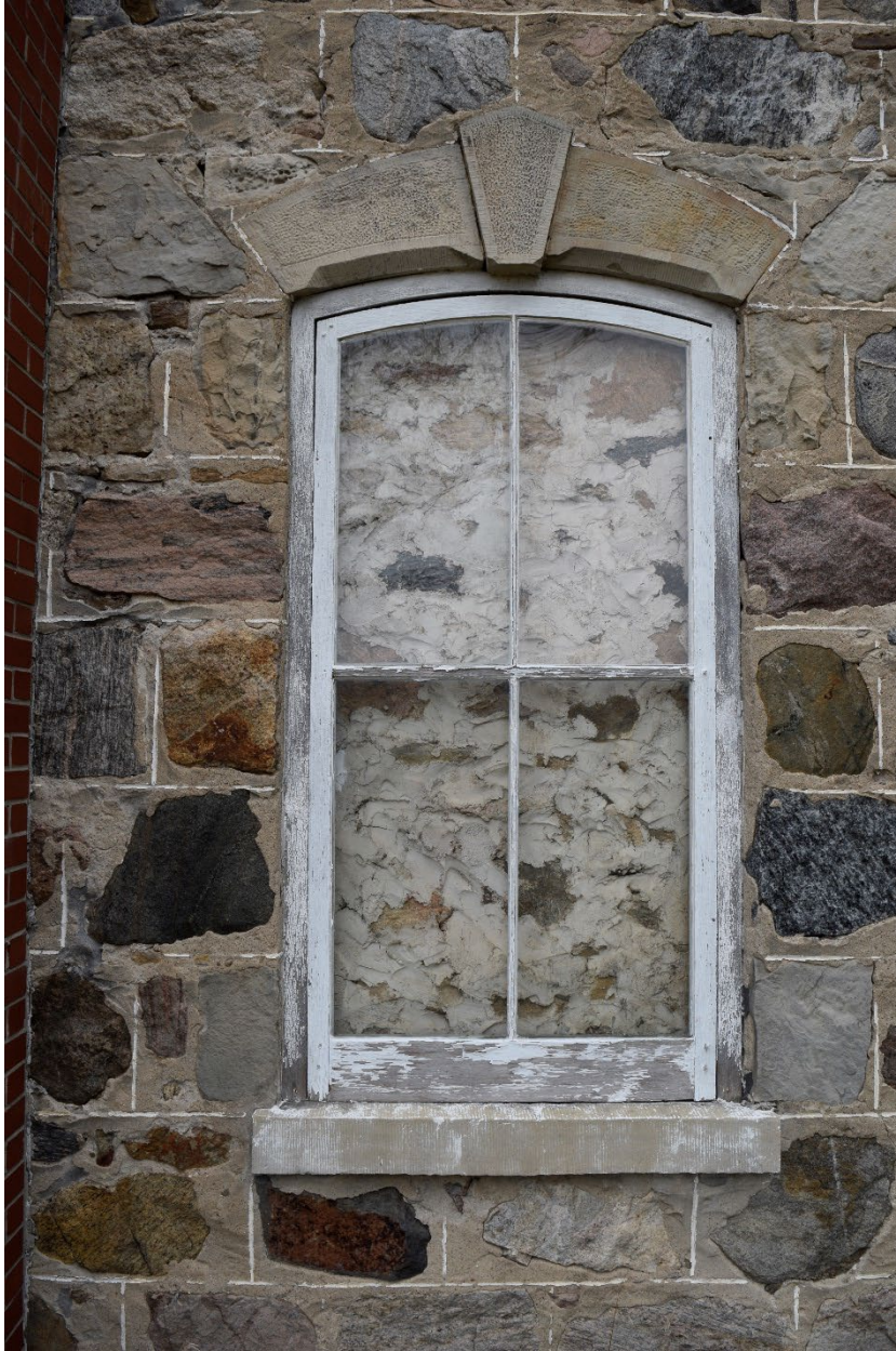
Figure 23: Blind window on north face of structure, stone and mortar are visible through the window, window is the original two over two sash window with original exterior storm
