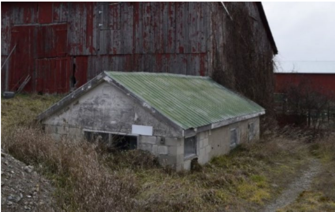
Figure 84: Semi subterranean milk house constructed of concrete masonry units
