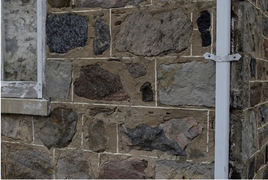
Figure 25: Close up of masonry as seen on gable ends and rear of structure, finish is not as finely dressed as that seen on front façade, note use of ribbon pointing (white lines) to create the appearance of coursed block
