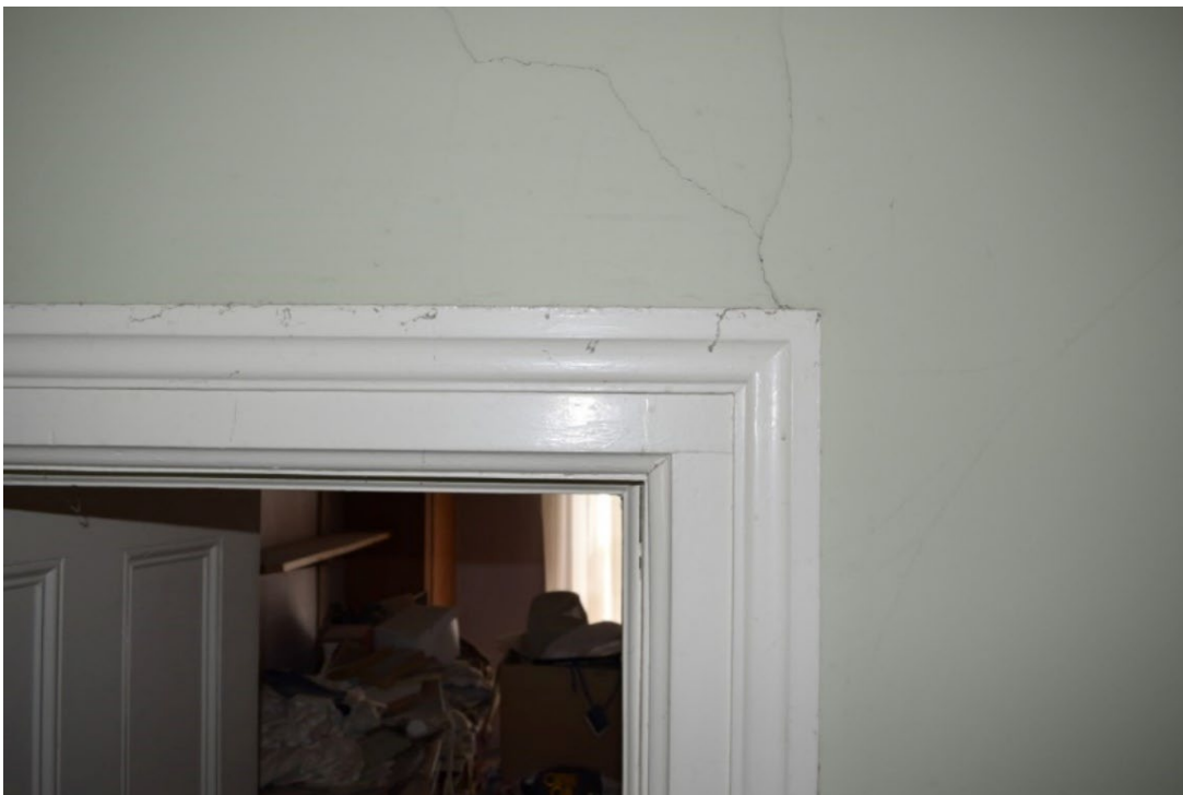
Figure 59: Trim profile used on second floor
