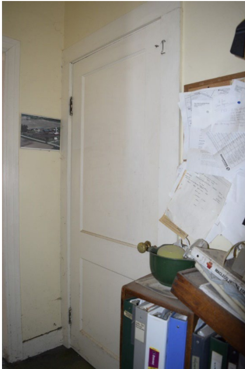
Figure 64: Example of replacement door typical of c.1950 renovations
