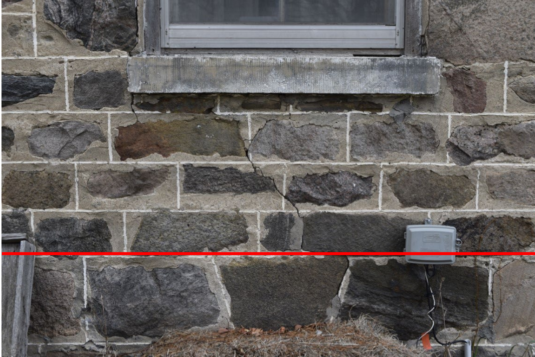
Figure 20: Exposure of fieldstone foundation on main structure. Red line indicates the divide between foundation and upper structure
