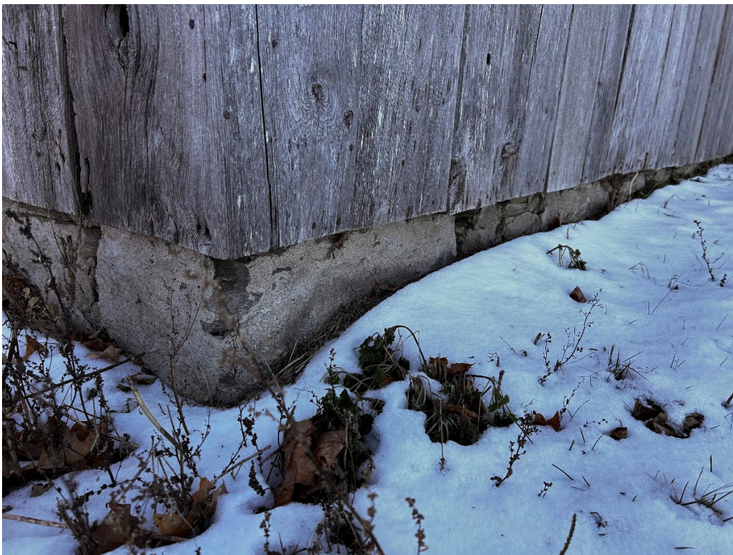
Figure 21: Field stone foundation with concrete repairs under rear wing
