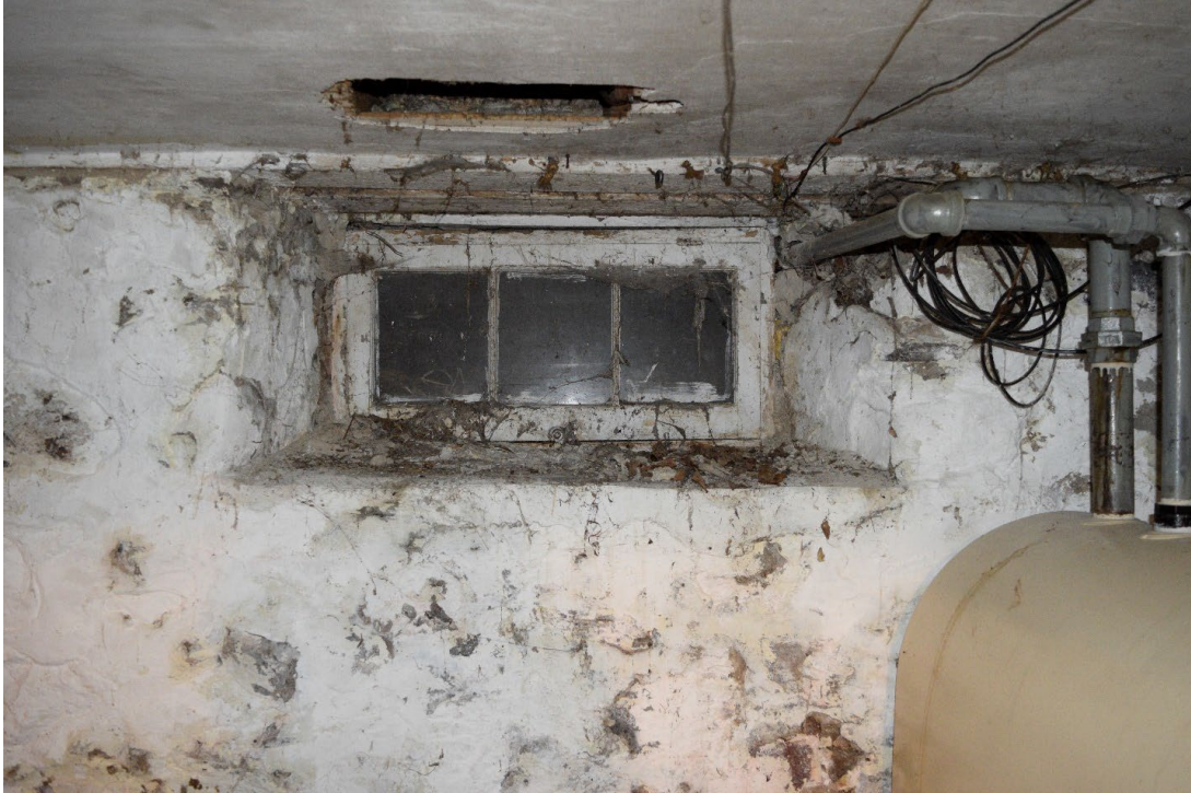
Figure 48: Typical example of an original awning style casement window in basement
