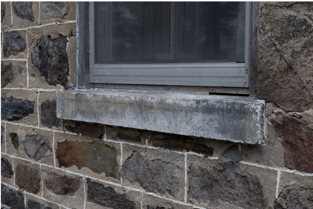
Figure 28: Typical example of finely crafted cut limestone lug sill used at all structural openings
