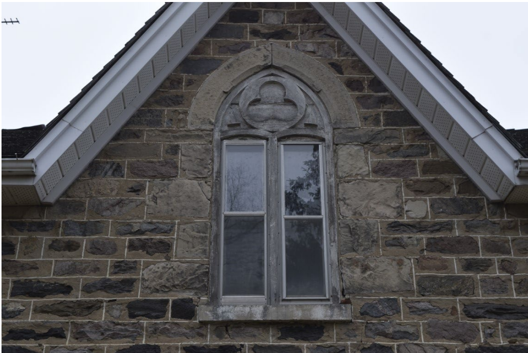
Figure 26: Lancet window in center gable, note the tri-foil detail, note the use of ribbon pointing (white lines) to create the appearance of fine coursed block on front façade
