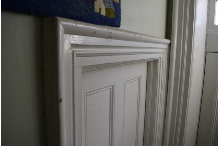
Figure 56: Original trim finish of main entrance, profile is more elaborate from that used in remainder of first floor and depicted in Figure 57
