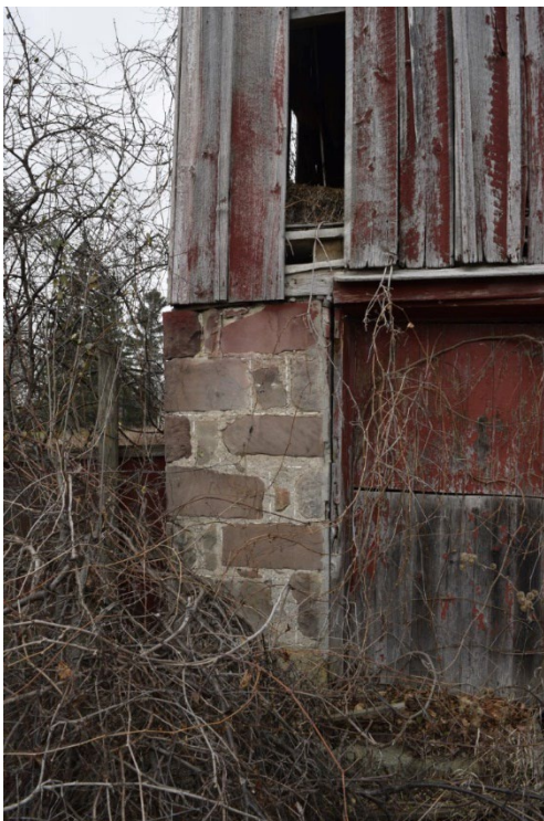
Figure 74: Use of red sandstone in southeast face of foundation of bank barn
