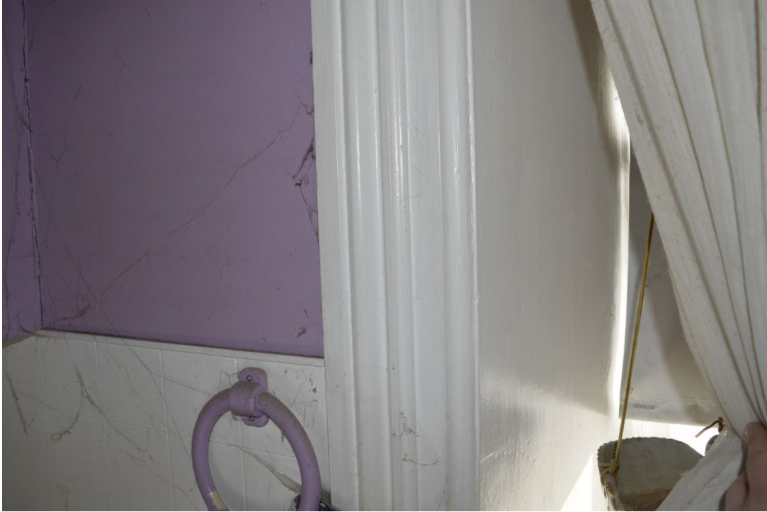
Figure 58: Original window trim profile as seen in washroom, first floor
