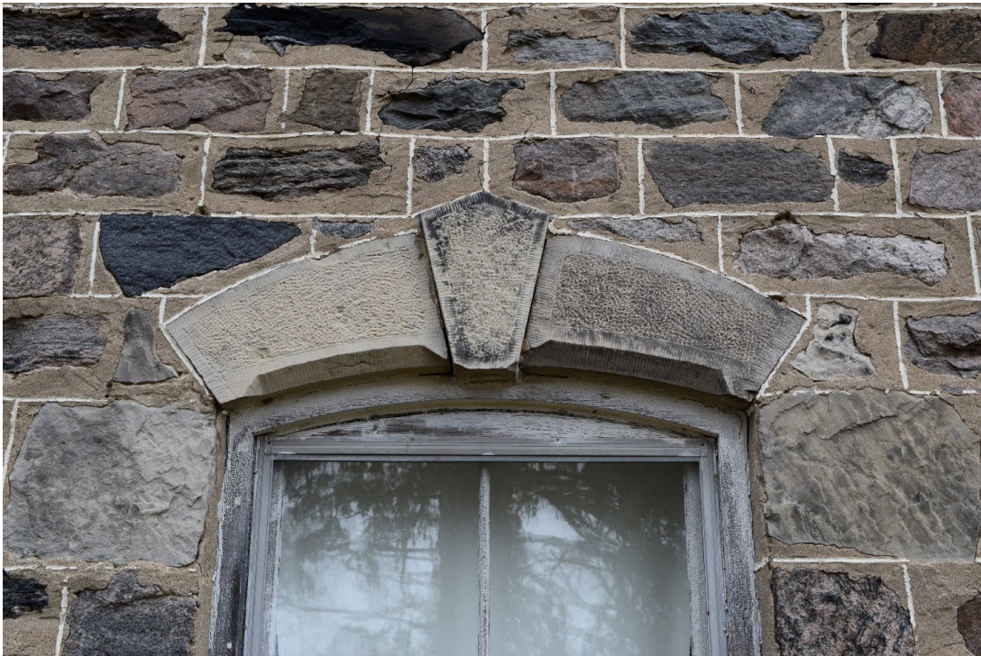
Figure 27: Typical example of finely crafted cut limestone lintel used at all structural openings
