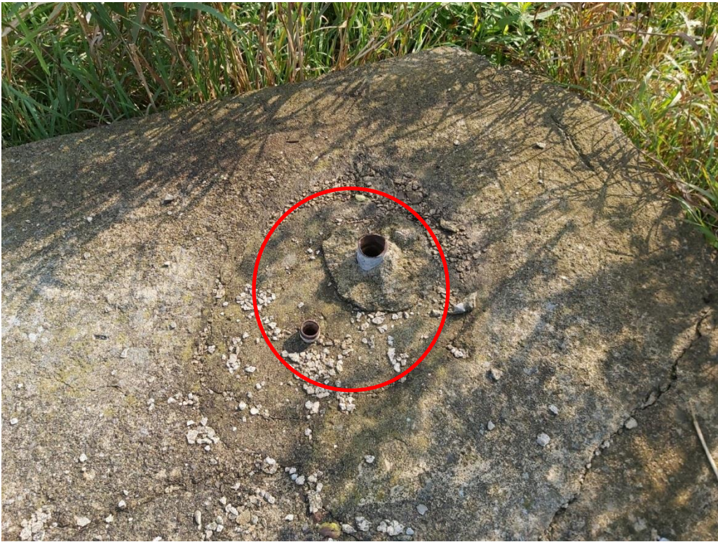
Photograph No. 19 – View of the two cut-off pipes extending through the concrete slab.
