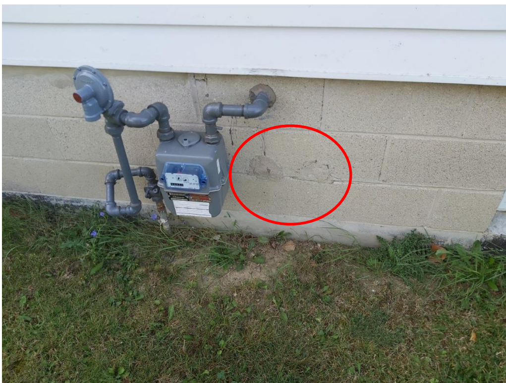
Photograph No. 22 – View of evidence of two former pipes associated with the former fuel oil AST located along the north exterior wall of the 12824 Dixie Road residential dwelling.
