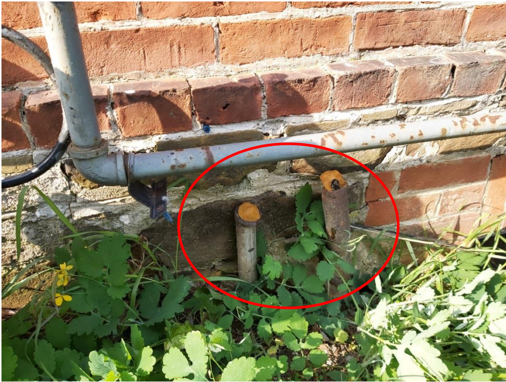
Photograph No. 5 – View of the two cut-off pipes associated with the former fuel oil AST located along the east exterior wall of the 12892 Dixie Road farmhouse.
