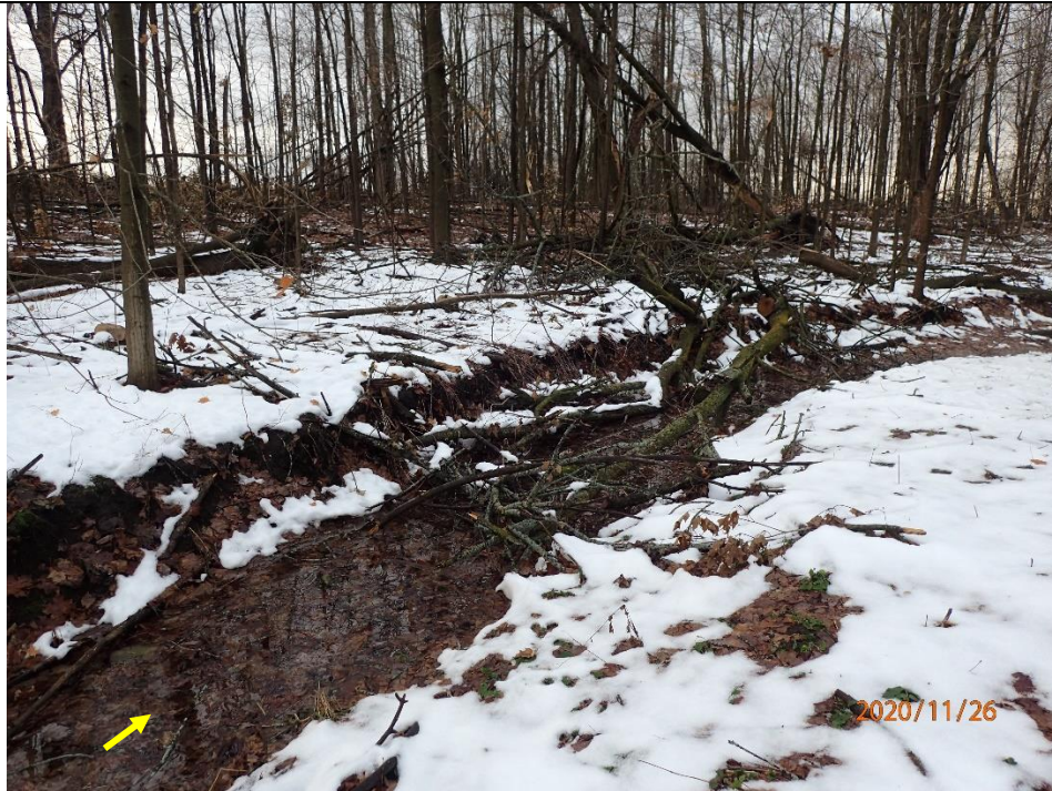
Photograph taken facing downstream. Approximately 50 to 70% of the bank network was considered stable, with recent signs of bank sloughing, slumping, and failure quite common. Further, stream bend areas were considered unstable.
