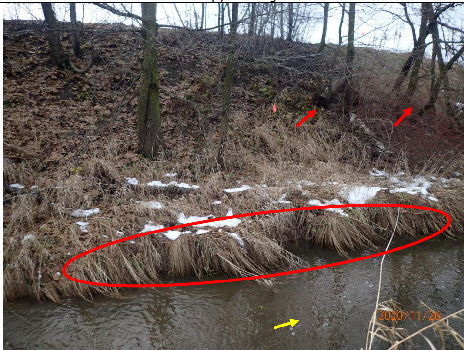
Photograph taken looking towards the left bank (facing downstream). Leaning and fallen trees were observed along the valley wall (arrows) and undercuts measured to 0.15 m in depth (circled). These observations indicated evidence of widening.
