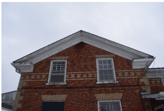
Plate 18: Cornice, eaves, and dichromatic brickwork, looking west
