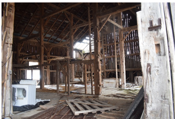
Plate 45: Loft, looking west showing hand hewn beams, posts, and joists
