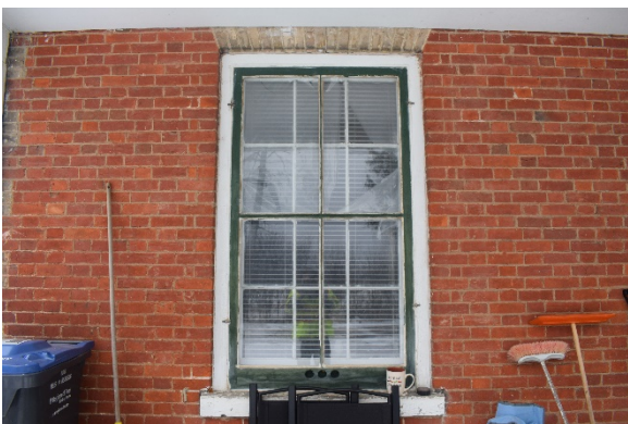
Plate 15: 6/6 windows and four pane storm window, looking north
