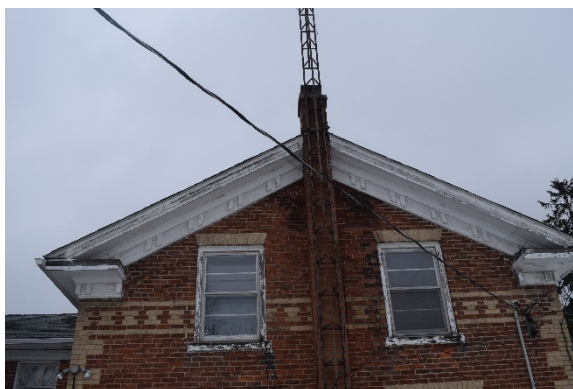
Plate 24: Cornice, return eaves, and dichromatic brick work, looking east
