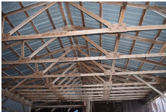
Plate 35: Interior of drive shed addition, showing machine cut beams, looking north
