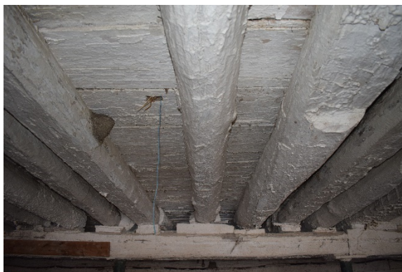
Plate 41: Hand hewn beams in stable
