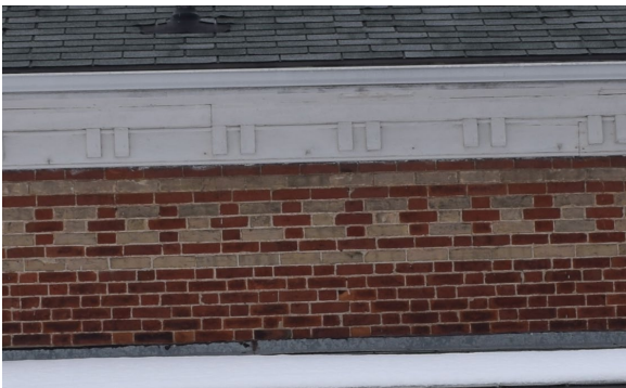
Plate 13: Denticulated cornice and dichromatic brick work, looking north
