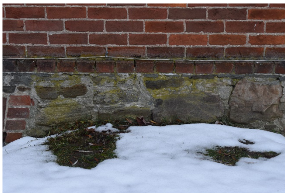
Plate 20: Field stone foundation, looking west
