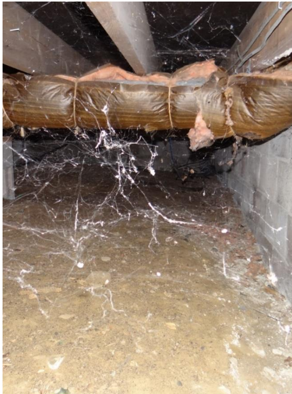
Plate 18: Crawl space underneath the eastern addition (ASI 2021)
