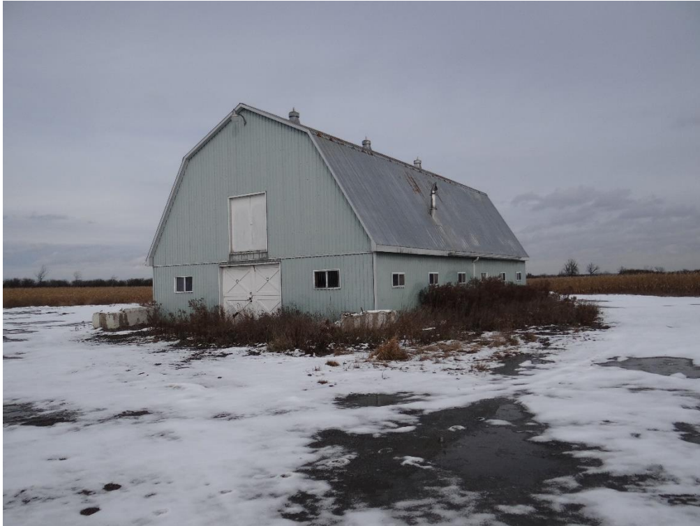
Plate 31: West façade of barn, looking northeast (ASI 2021)
