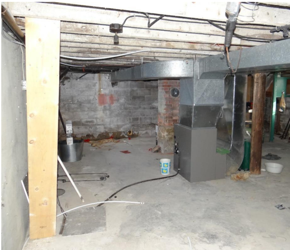
Plate 16: Concrete block walls and wood beams in basement (ASI 2021)
