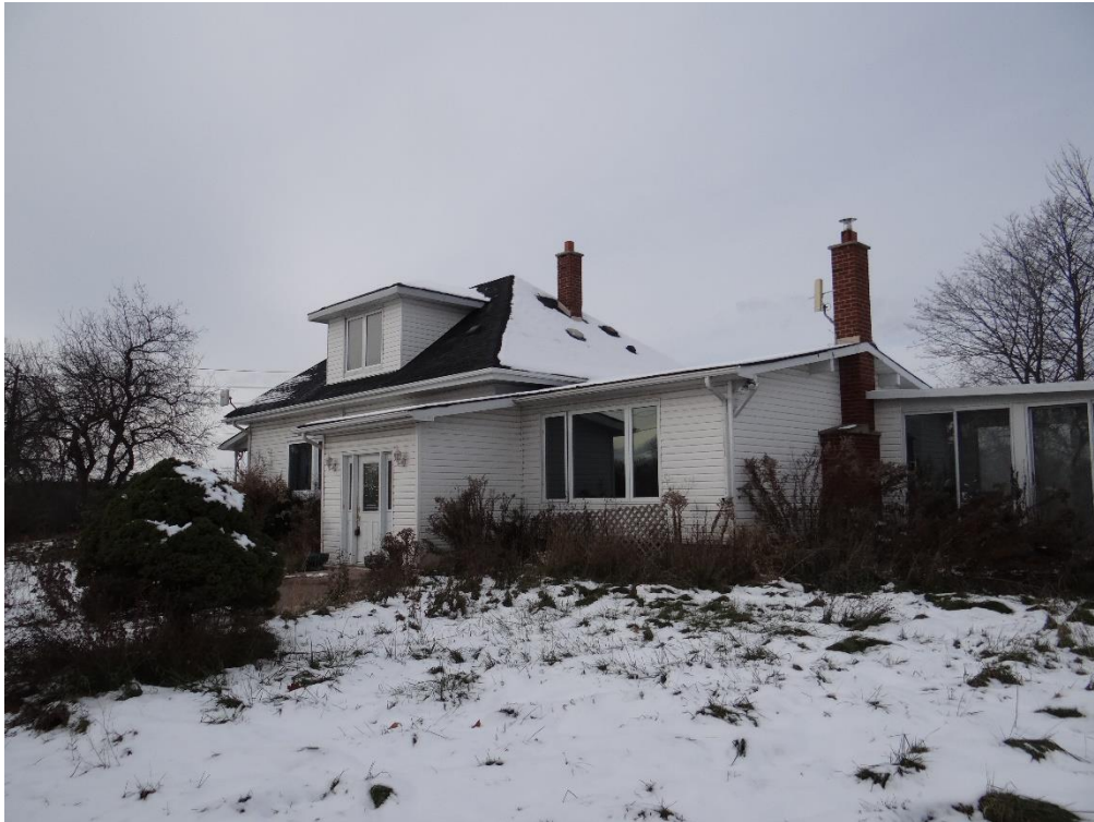
Plate 15: Chimney from original building and from rear (east) addition, looking northwest (ASI 2021)
