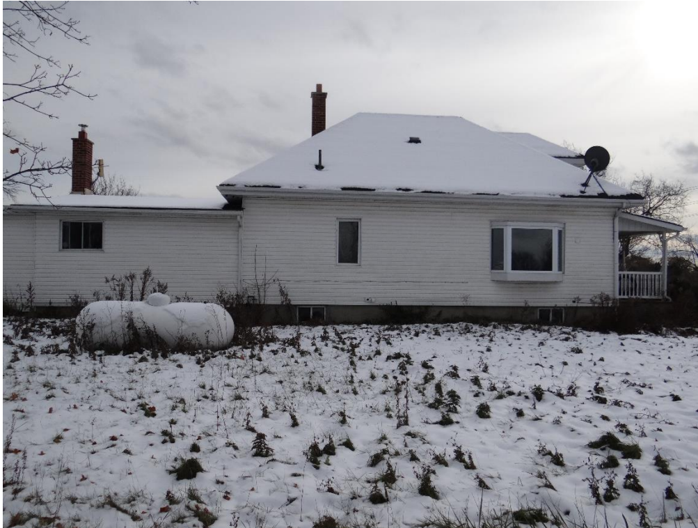
Plate 13: Northern elevation of 12541 Airport Road (ASI 2021)
