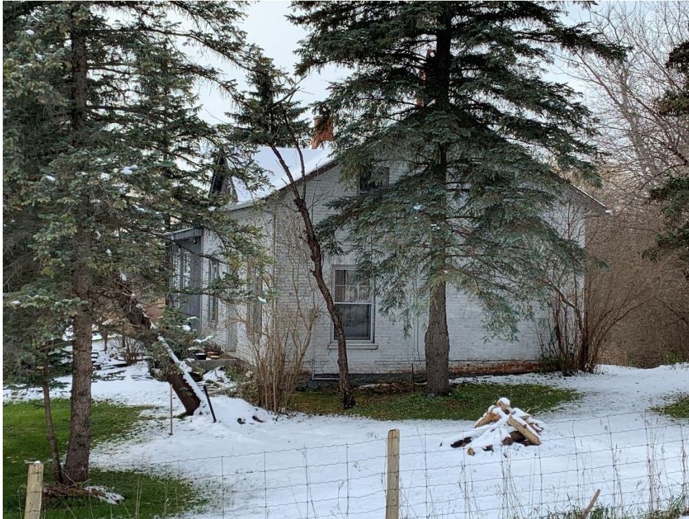
Plate 7: Residence at 12542 Airport Road (ASI 2021)
