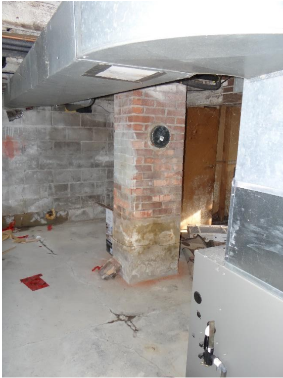
Plate 17: View of the chimney base (ASI 2021)
