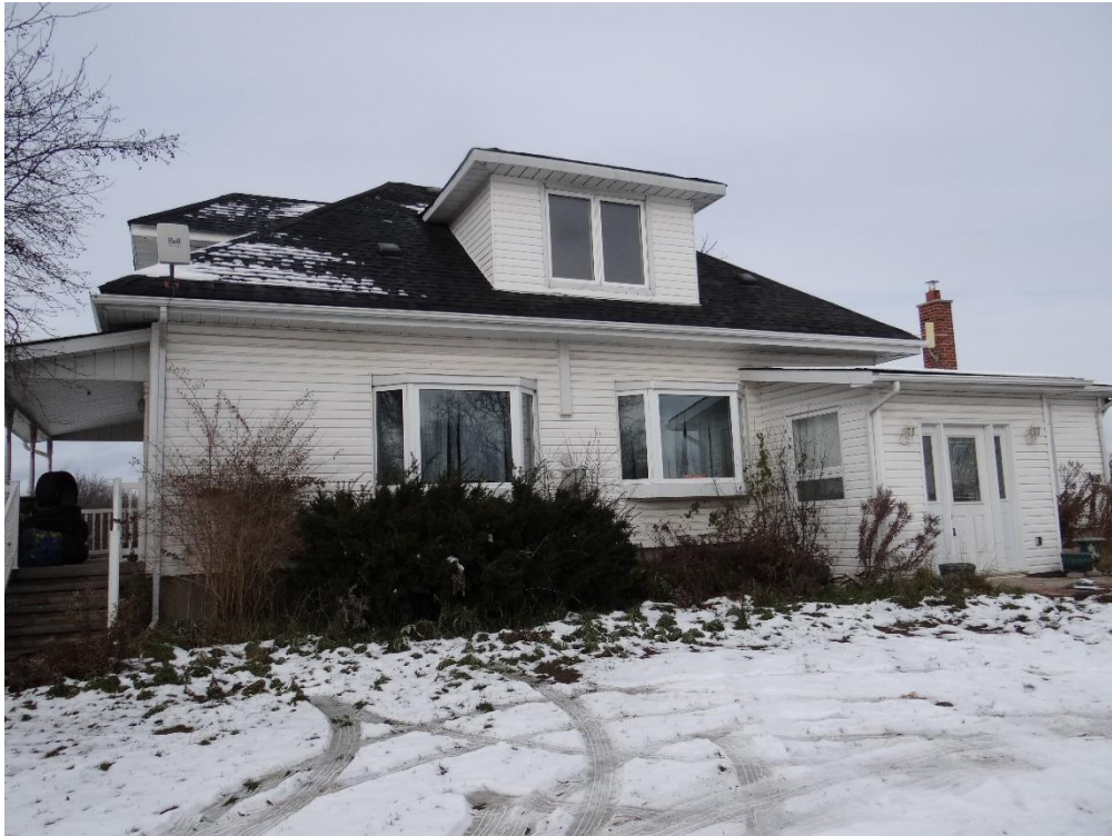
Plate 11: Southern elevation of 12541 Airport Road (ASI 2021)
