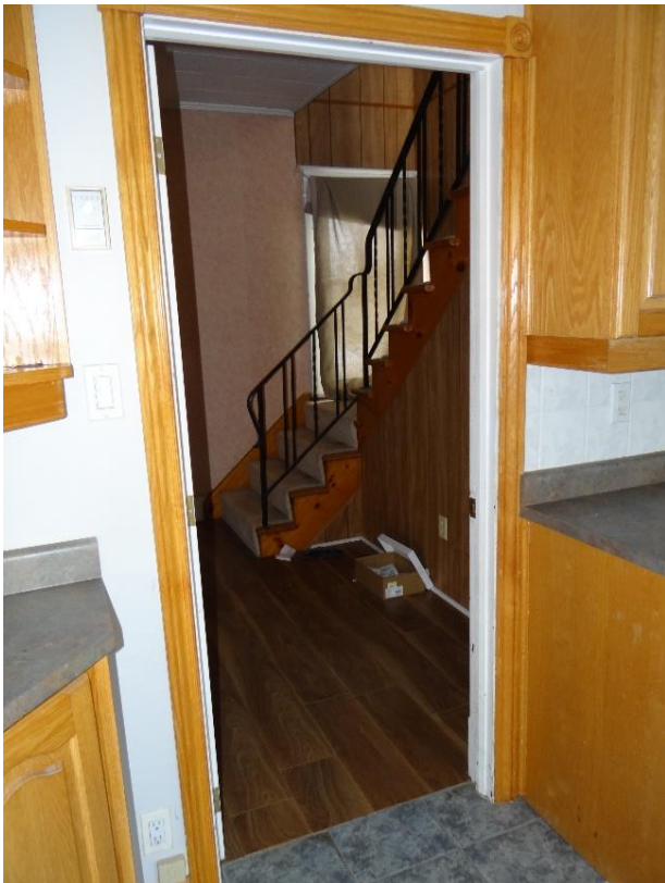
Plate 23: Staircase landing area off kitchen on main floor (ASI 2021)
