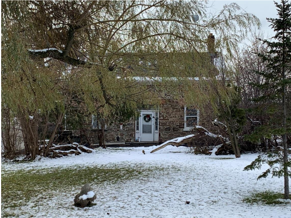
Plate 8: Residence at 12620 Airport Road (ASI 2021)
