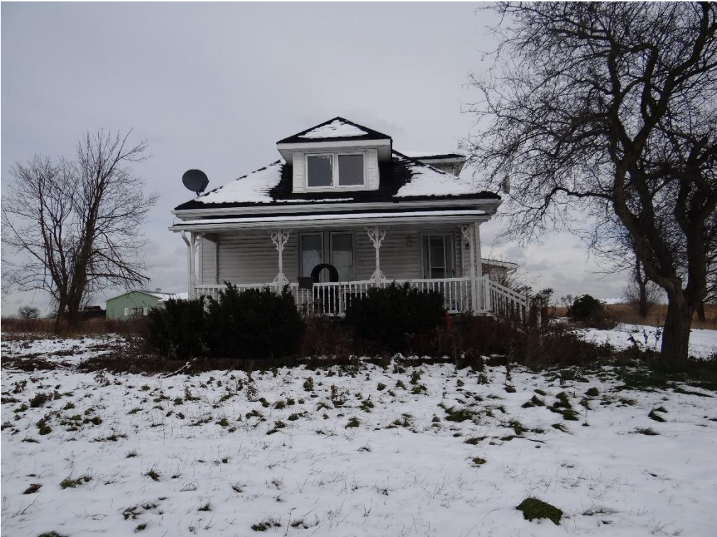
Plate 9: Western elevation of 12541 Airport Road (ASI 2021)
