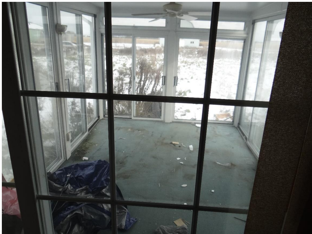
Plate 25: Enclosed sunroom off the rear addition (ASI 2021)
