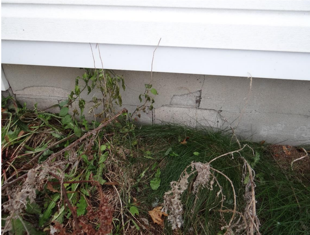
Plate 14: Concrete block foundation and parging (ASI 2021)
