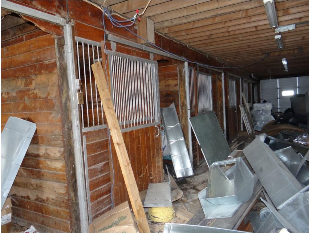
Plate 33: Barn's interior, featuring former horse pens (ASI 2021)
