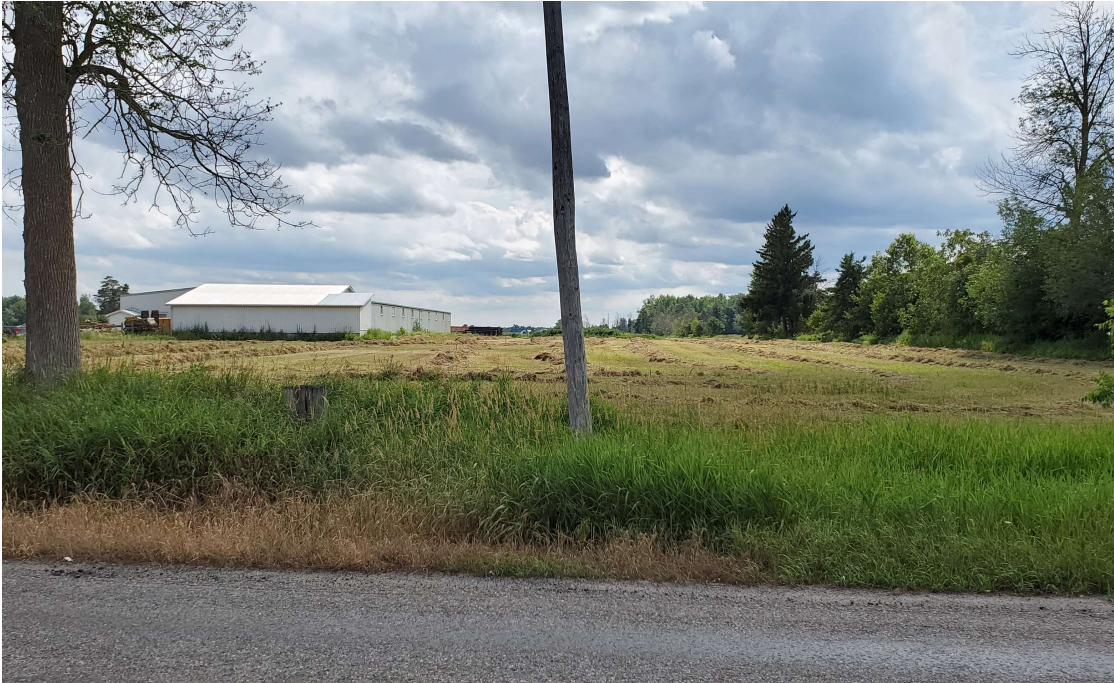
Photo No. 1 - Looking at west to north side of barn and property at 12472 Chinguacousy Road. No evidence of livestock use of the barn and paddocks removed for cropping hay. (July 21, 2020)
