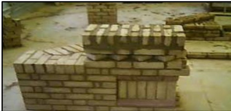
Photograph 8: Examples of Freeze Boards, Soldier Coursing, Quoining and Lintels
