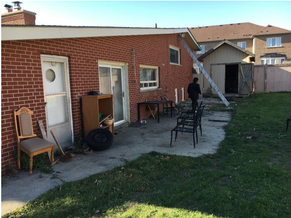
Photo 6: View of the east side of the house, looking north.
