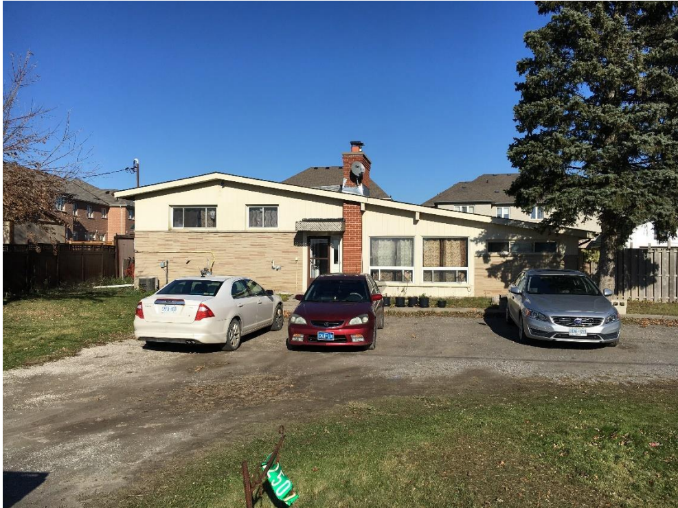
Photo 2: View of the two-storey house at the central-northern portion of the Site, looking east.
