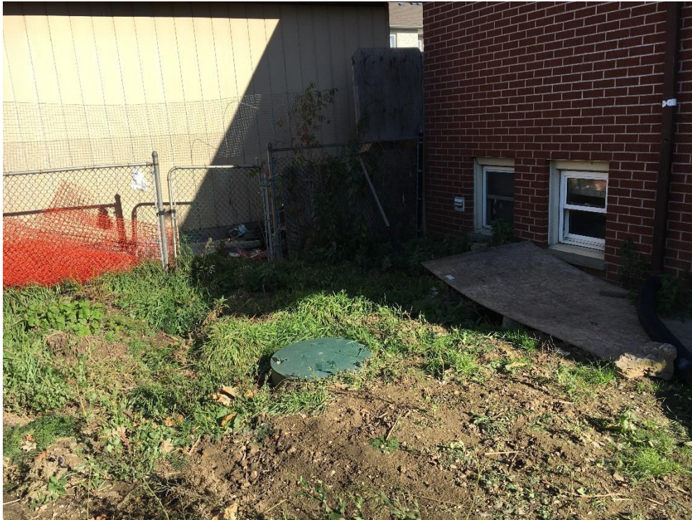
Photo 4: View of the septic tank situated north of the house, looking southeast.
