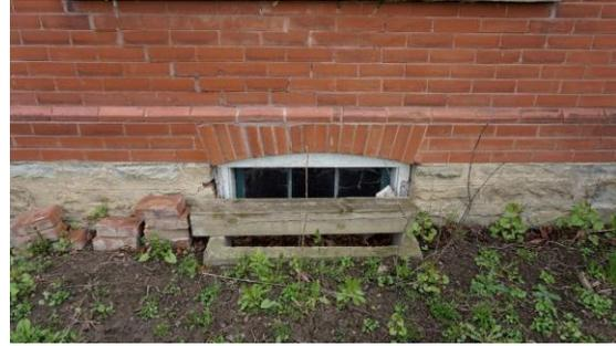
**Photo 5: Example of a basement window with a segmental frame and brick voussoir**
