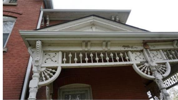
**Photo 9: Detail of spindle work on the porch**
