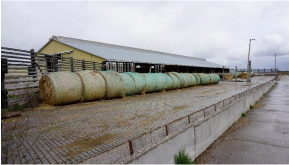
Photo 76: Cattle outbuilding, south elevation looking northeast
