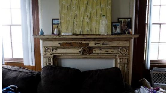
Photo 22: Fireplace mantle in front living room looking west
