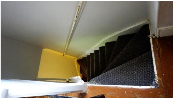
Photo 46: Winding staircase to second floor of rear tail
