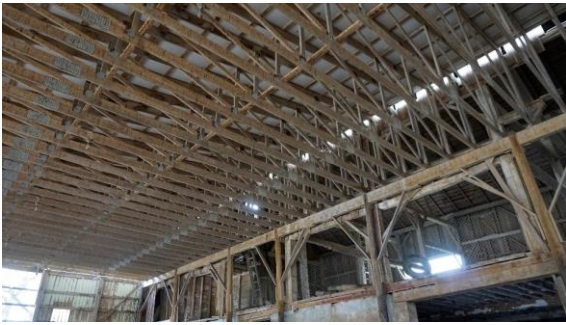
Photo 73: Addition wood framing with steel braces
