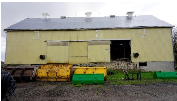
Photo 56: North elevation looking south
