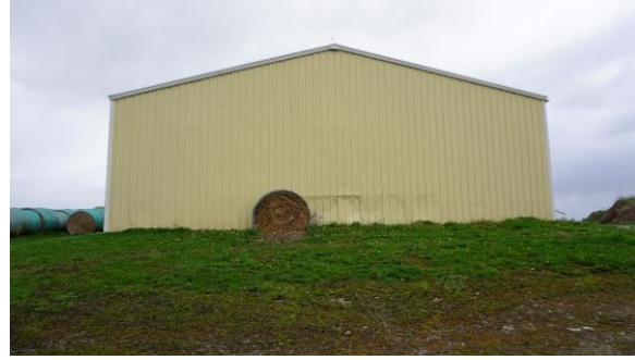
Photo 81: East outbuilding, west elevation looking east
