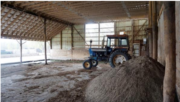
Photo 71: Addition looking southwest
