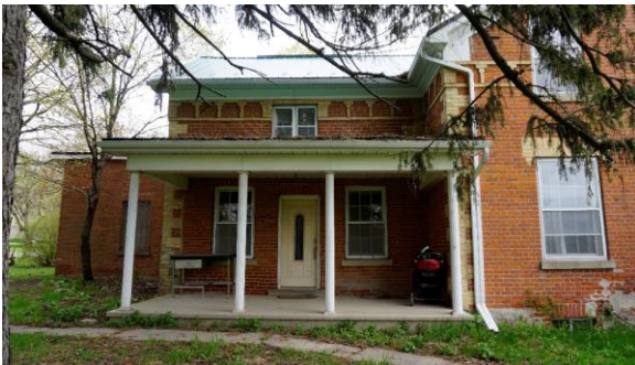
Photo 15: West elevation rear tail porch
