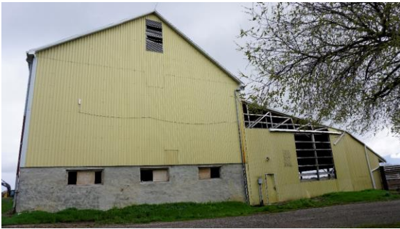
Photo 58: West elevation looking southeast
