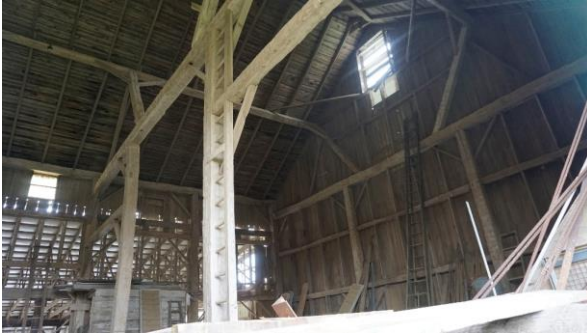
Photo 66: Upper storey looking southwest
