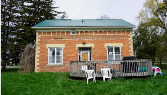
Photo 5: Front façade looking north
