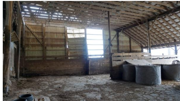
Photo 72: Addition looking southeast
