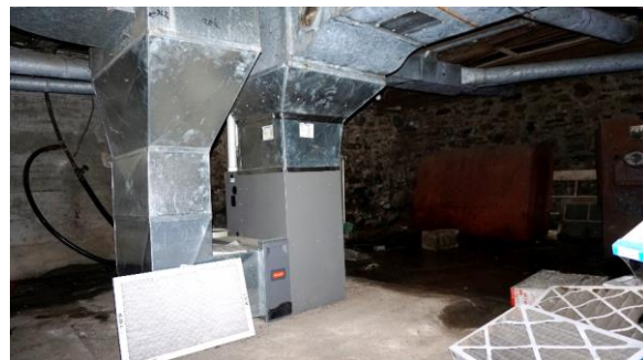
Photo 54: Basement looking southeast
