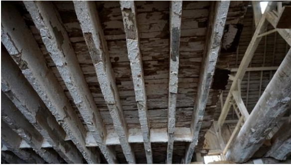
Photo 69: Machine cut wood beams
