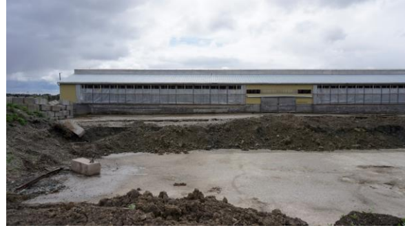
Photo 77: Cattle outbuilding, north elevation looking south
