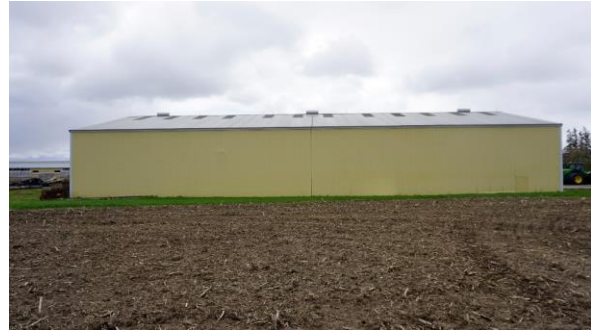
Photo 87: West outbuilding, north elevation looking south
