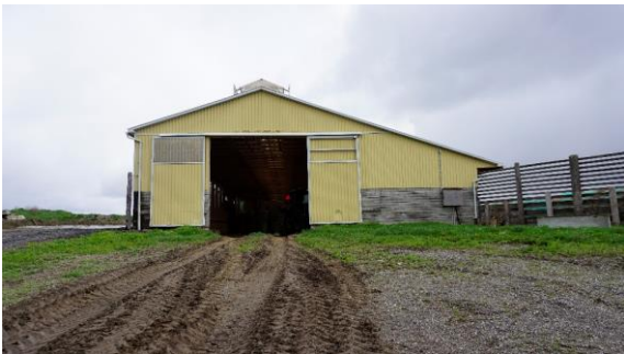
Photo 74: Cattle outbuilding, west elevation looking east
