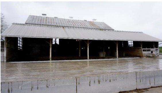
Photo 60: South elevation looking northeast
