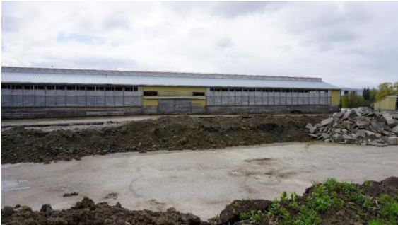
Photo 78: Cattle outbuilding, north elevation looking southwest
