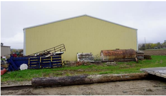
Photo 88: West outbuilding, east elevation looking west
