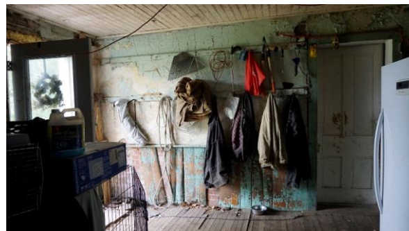
Photo 36: Rear addition looking south
