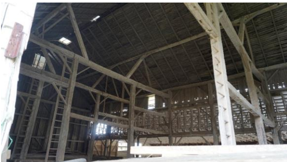
Photo 64: Upper storey looking southeast
