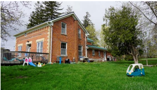
Photo 7: Front façade and east elevation looking northwest
