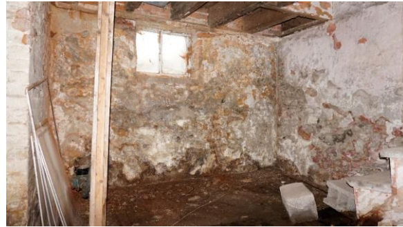
Photo 52: Basement looking northwest
