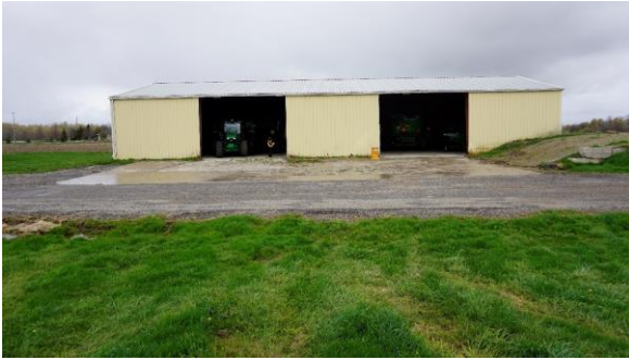
Photo 80: East outbuilding, south elevation looking north
