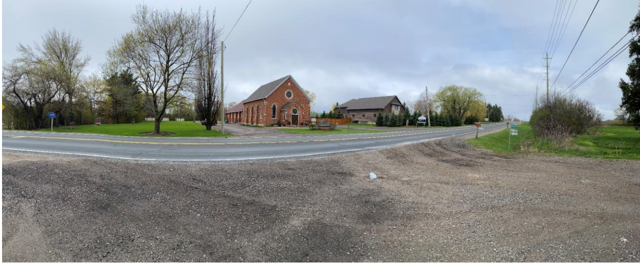
Photo 4: Adjacent Mayfield United Church, looking northwest from Study Area
