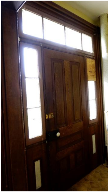
Photo 17: Front entry door
