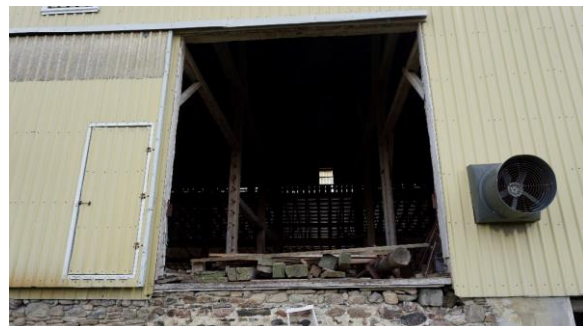
Photo 57: North elevation sliding door and ventilator fan
