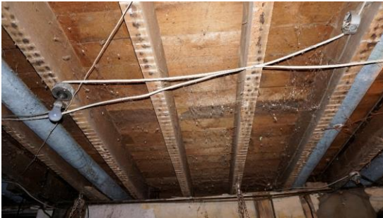
Photo 55: Basement machine cut beams
