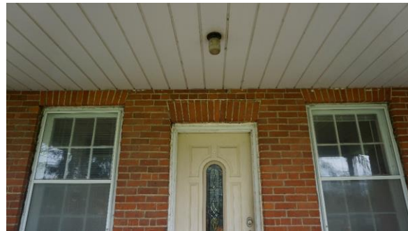
Photo 16: West elevation rear tail entrance and windows
