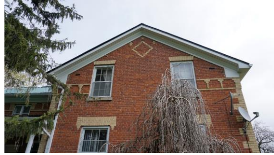
Photo 14: West elevation of gabled end
