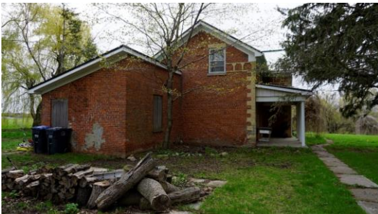
Photo 11: North elevation looking south
