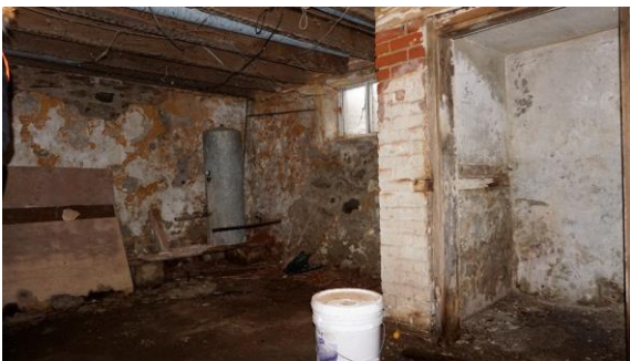
Photo 53: Basement looking southwest
