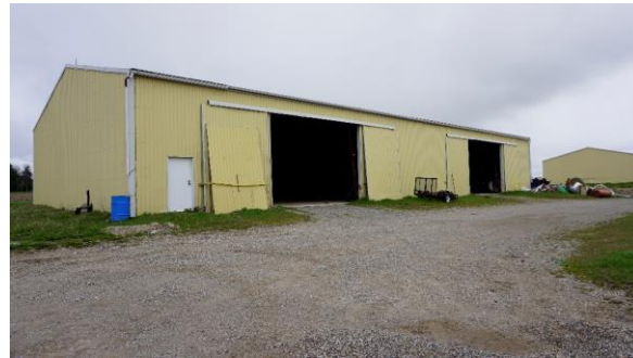
Photo 85: West outbuilding, south elevation looking northeast
