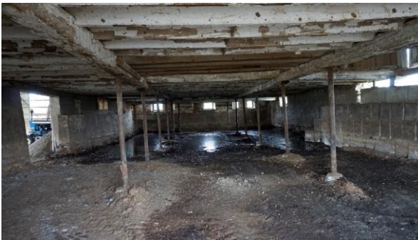
Photo 67: Lower storey looking northwest
