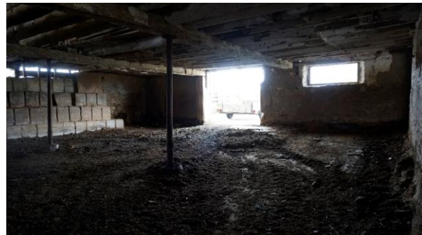
Photo 68: Lower storey looking northeast
