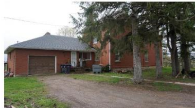
Photo 20: North elevation of addition looking southwest
