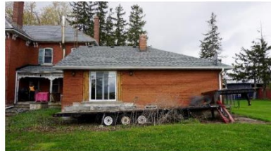
Photo 14: South elevation of addition looking north
