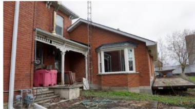
Photo 13: West elevation of addition looking northeast
