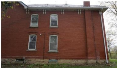
Photo 17: North elevation looking south
