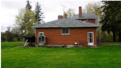
Photo 15: East elevation of addition looking west
