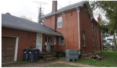
Photo 16: East elevation of the original residence looking southwest
