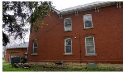
Photo 18: North elevation looking southeast
