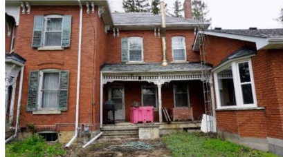
Photo 12: South elevation porch looking north
