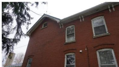
Photo 19: North elevation gabled bay looking southeast
