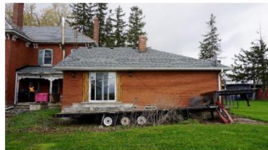
Photo 14: South elevation of addition looking north
