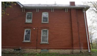
Photo 17: North elevation looking south
