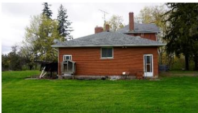
Photo 15: East elevation of addition looking west
