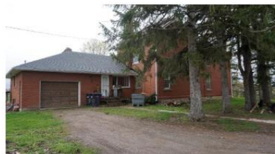
Photo 20: North elevation of addition looking southwest
