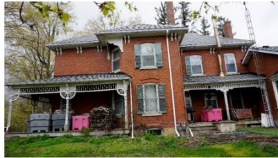
Photo 11: South elevation looking north
