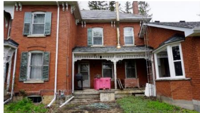
Photo 12: South elevation porch looking north
