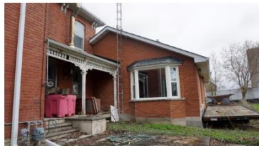
Photo 13: West elevation of addition looking northeast
